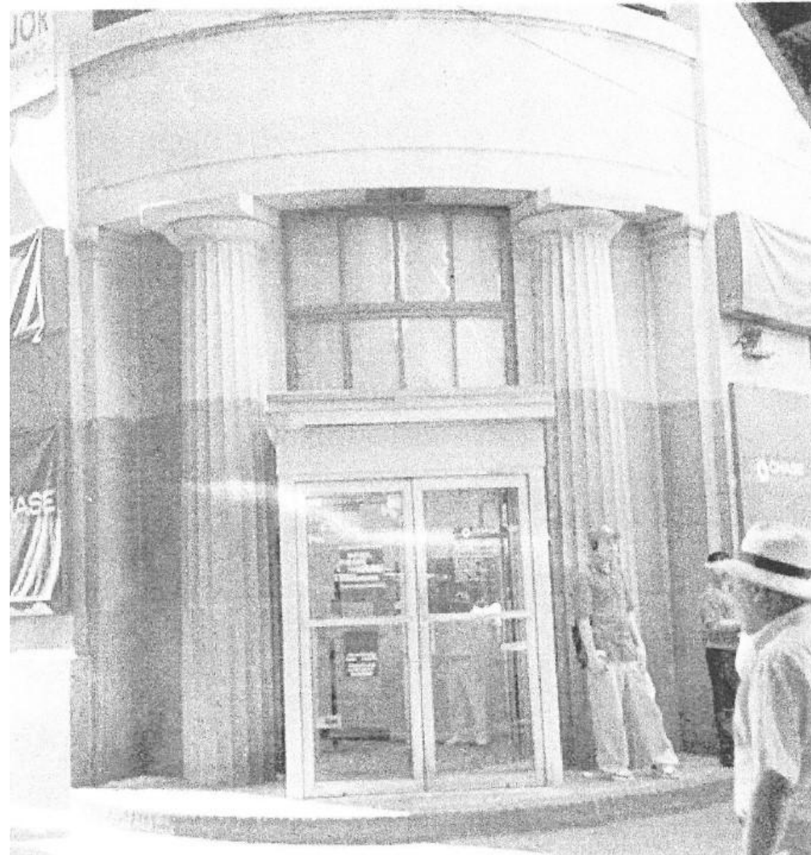
VESTIBULE PRIOR TO VESTIBULE REMOVAL
