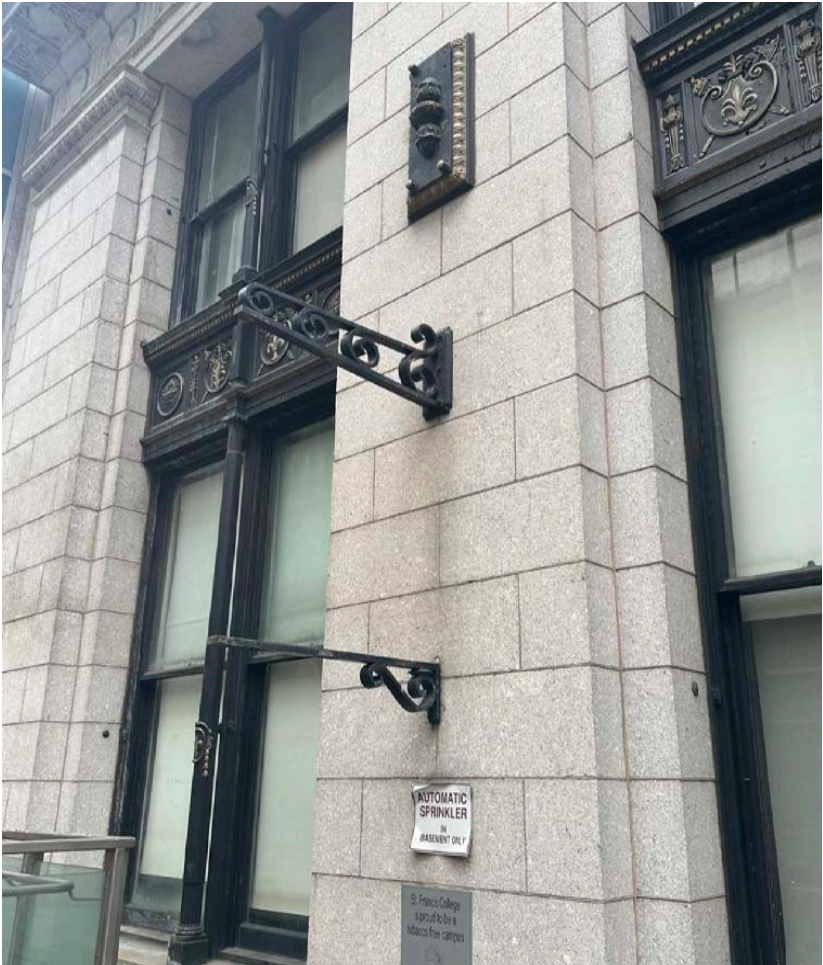
Exist. Signage Brackets on Left Side of Entrance
