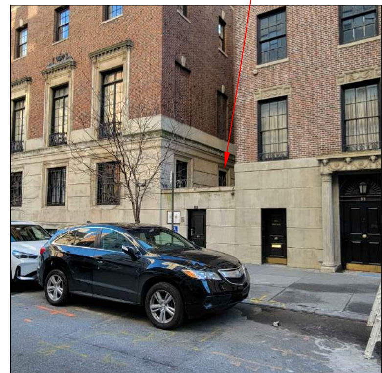
DOOR TO REAR COURT ON 69TH STREET
