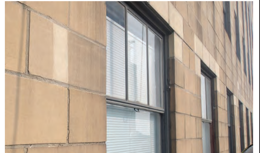
AREA OF PREVIOUSLY REPLACED TERRA COTTA UNITS
