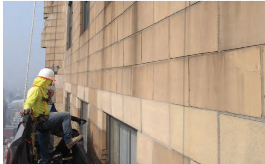
AREA OF PREVIOUSLY REPLACED TERRA COTTA UNITS
