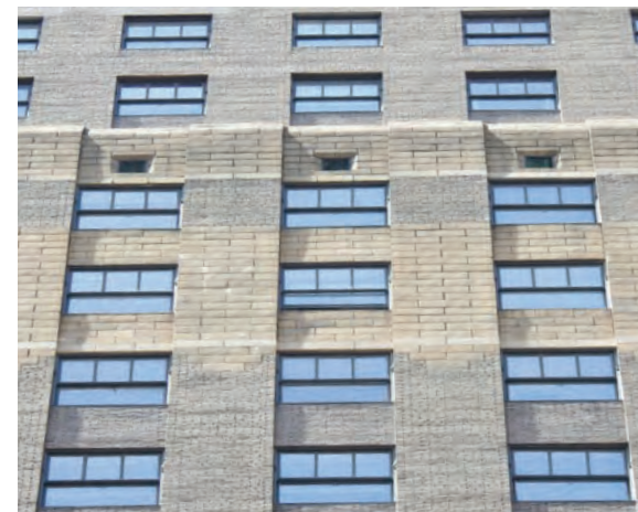
AREA OF PREVIOUSLY REPLACED TERRA COTTA UNITS
