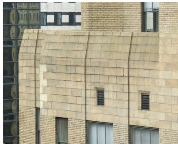
AREA OF PREVIOUSLY REPLACED TERRA COTTA UNITS
