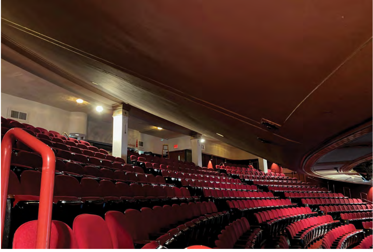
VIEW F - EXISTING PLASTERED CEILING AT MEZZANINE LEVEL
