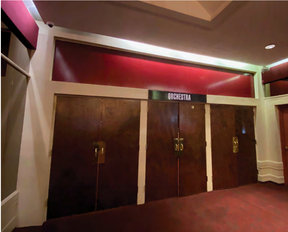
EXISTING NON-HISTORIC AUDITORIUM DOORS FROM LOBBY SIDE
