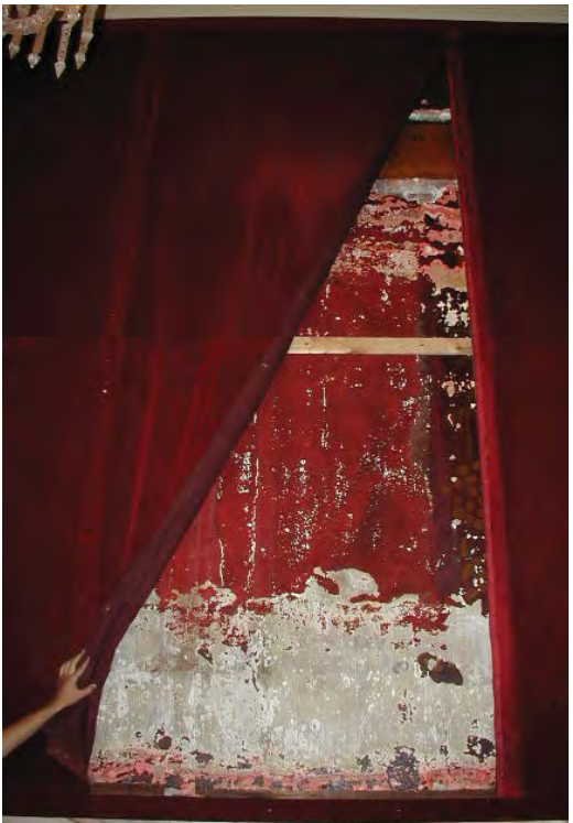
EXISTING CONDITIONS OF PLASTER WALLS UNDERNEATH FABRIC WRAPPED WALL PANELING
