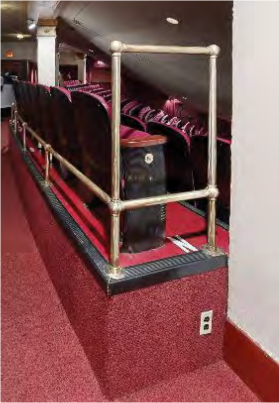
VIEW D - MEZZANINE LEVEL, LOOKING NORTH
