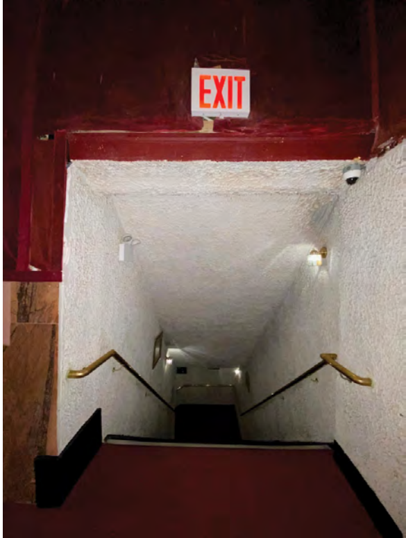
VIEW C - EXISTING STAIR ENTRANCE OPENING AT BALCONY LEVEL
