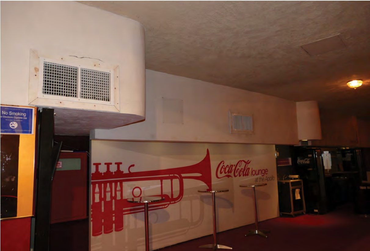
VIEW E - REAR WALL OF MEZZANINE LEVEL
