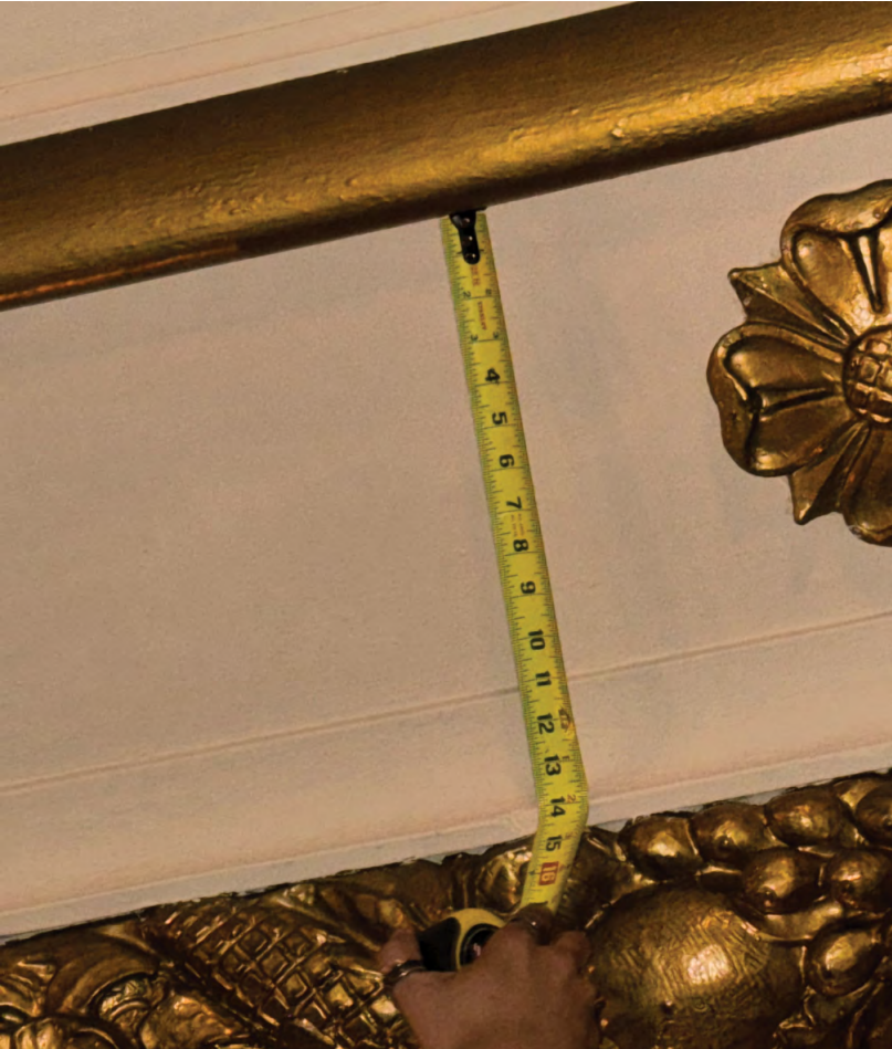
EXISTING CONDITION AT DECORATIVE PLASTER MOLDING AT AUDITORIUM CEILING WITH 11" WIDE FLAT SURFACE
