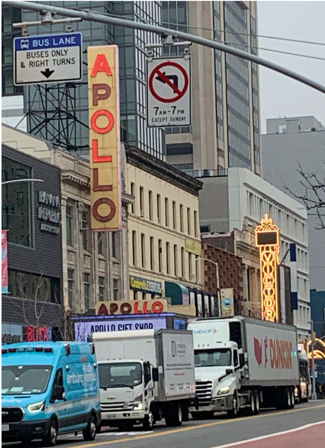
MALFUNCTIONING NEON LETTERS DUE TO HUMIDITY AND RAIN
