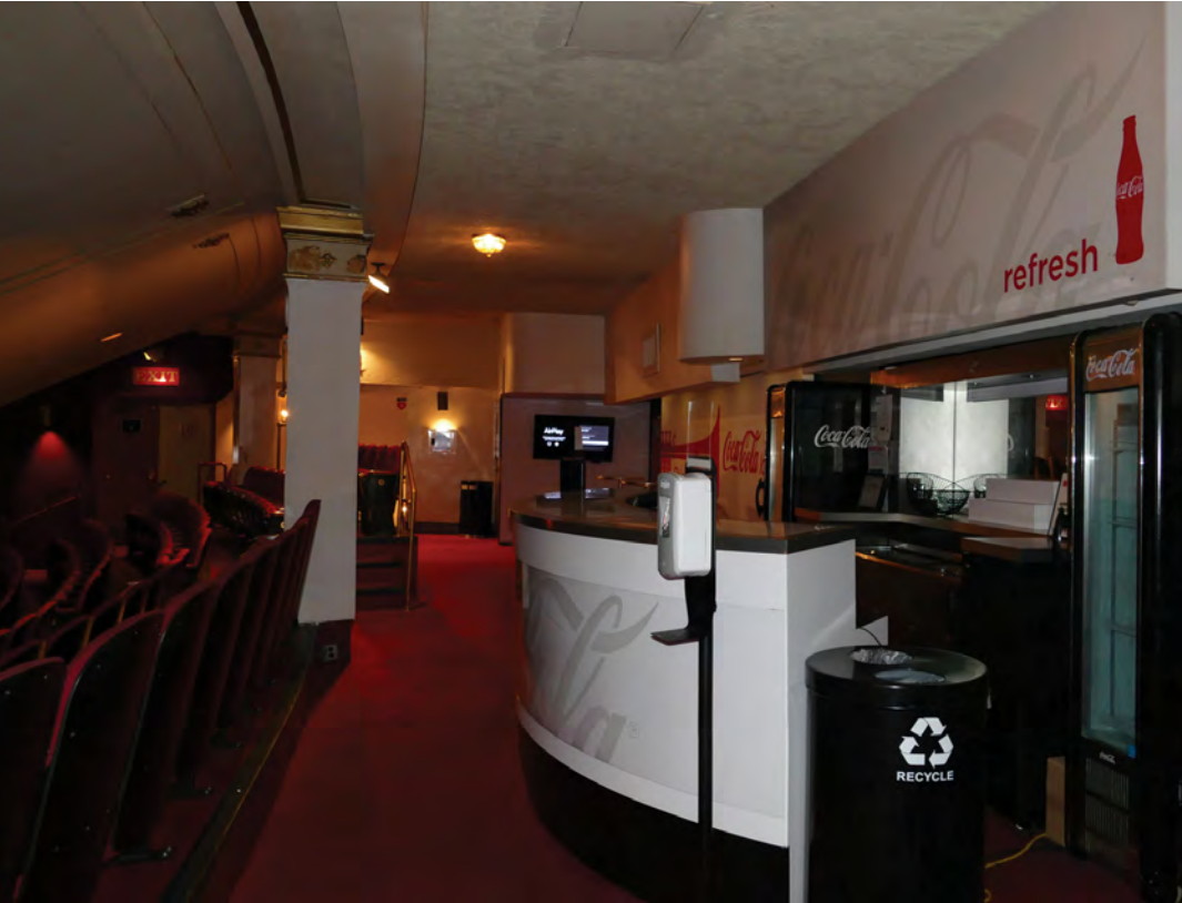
VIEW A - MEZZANINE LEVEL, LOOKING SOUTH. AN EXISTING SOFFIT EXISTS ALONG THE WEST WALL WITH ENCLOSED HVAC DUCTWORK & DIFFUSERS
