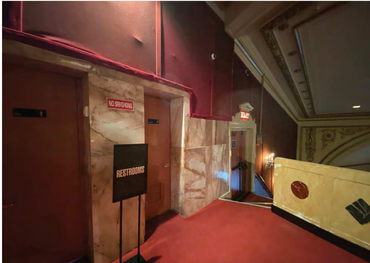
EXISTING FABRIC WRAPPED WALL PANELING CONDITIONS
