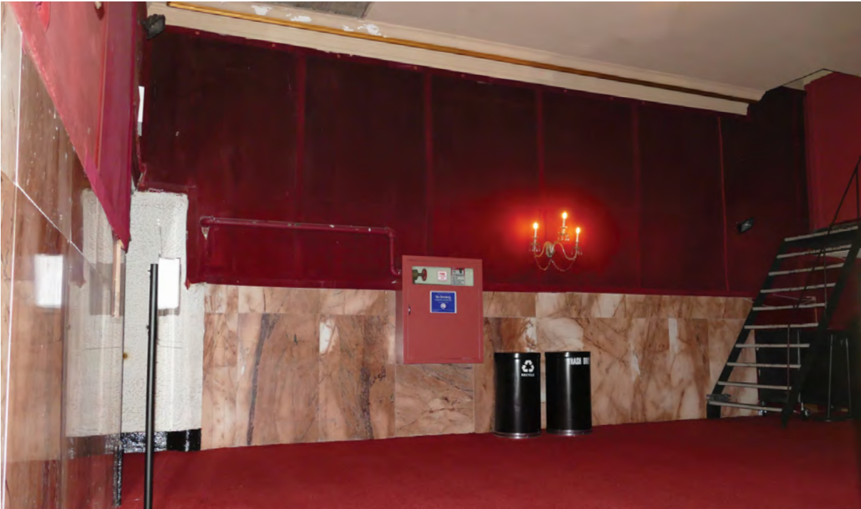
VIEW D - REAR WALL AT BALCONY LEVEL
