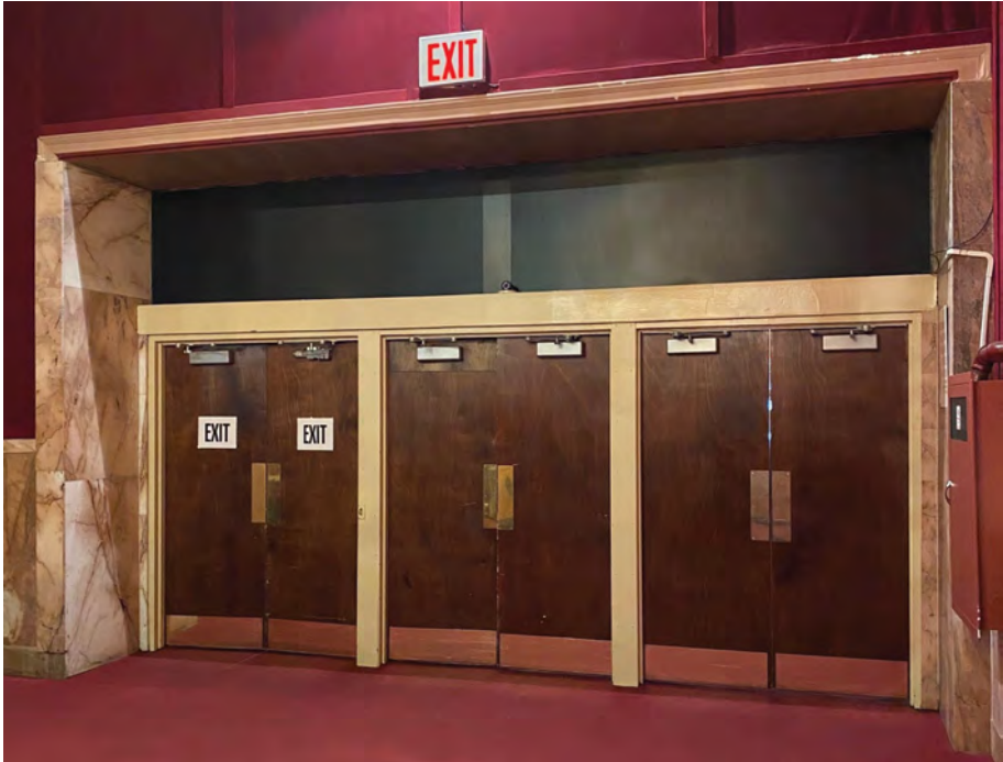
EXISTING EXIT SIGN AT AUDITORIUM, CODE COMPLIANT, REPLACED WITH EX-01 EXIT SIGN
