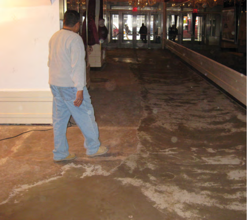
VIEW C - REMNANTS OF EXISTING LOBBY TERRAZZO FLOORING UNDER CARPET IN POOR CONDITIONS, DAMAGED AND PATCHED
