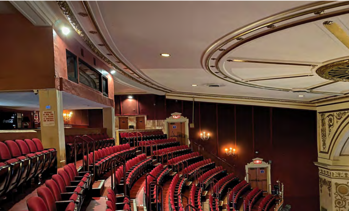
VIEW E - EXISTING PAINTED PLASTER CEILING & DECORATIVE MOLDING AT BALCONY LEVEL
