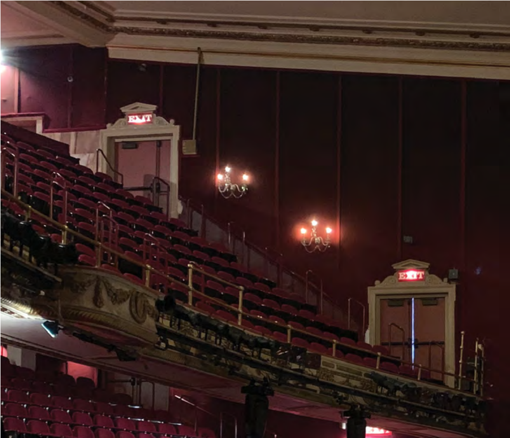
EXISTING FABRIC WRAPPED WALL PANELING DETAIL
