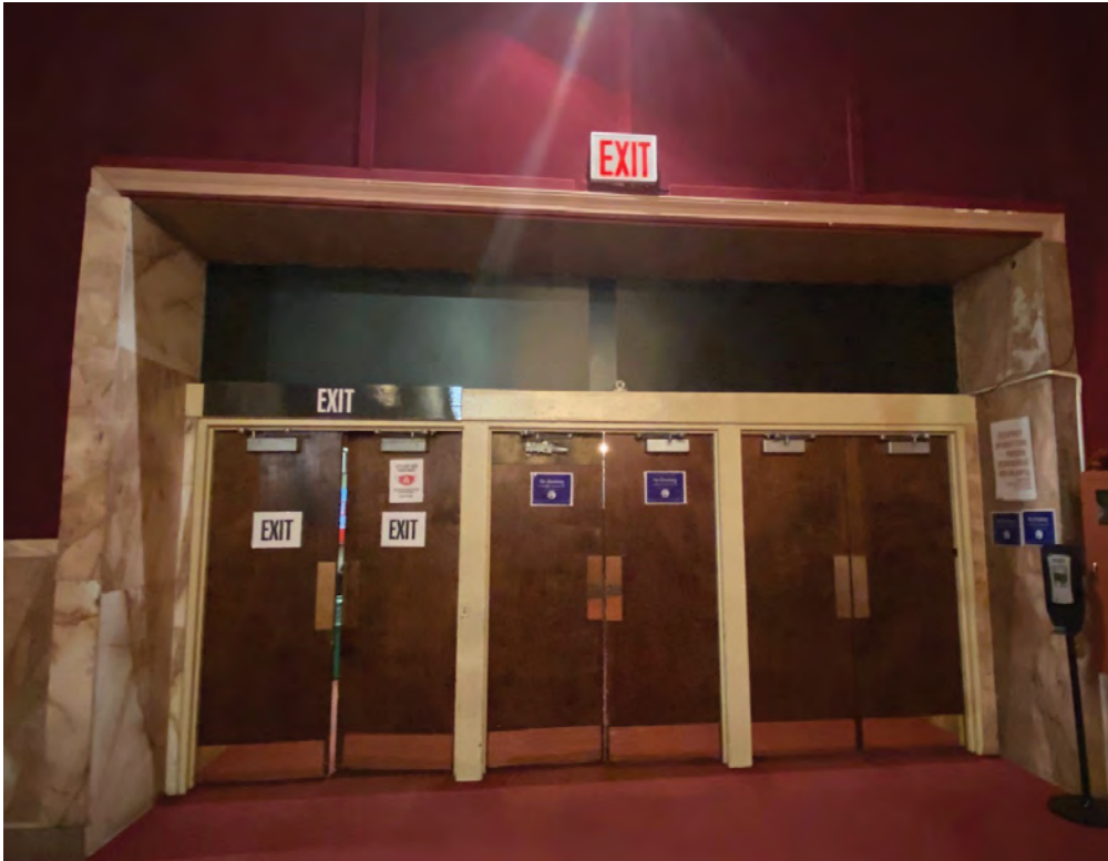
EXISTING NON-HISTORIC AUDITORIUM DOORS FROM AUDITORIUM SIDE
