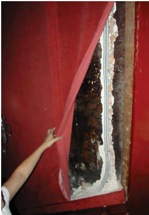
EXISTING CONDITIONS OF PLASTER WALLS UNDERNEATH FABRIC WRAPPED WALL PANELING
