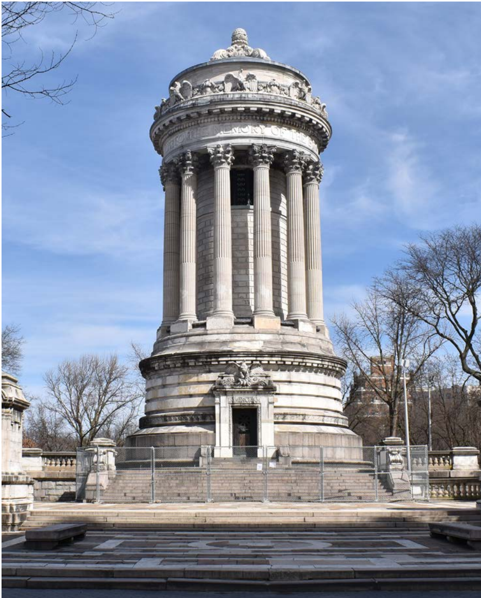
Tower Exterior Repair — Remediate deteriorated mortar & masonry joints — Repair & replace roofing and flashing — Repair & restore corroded metal elements
