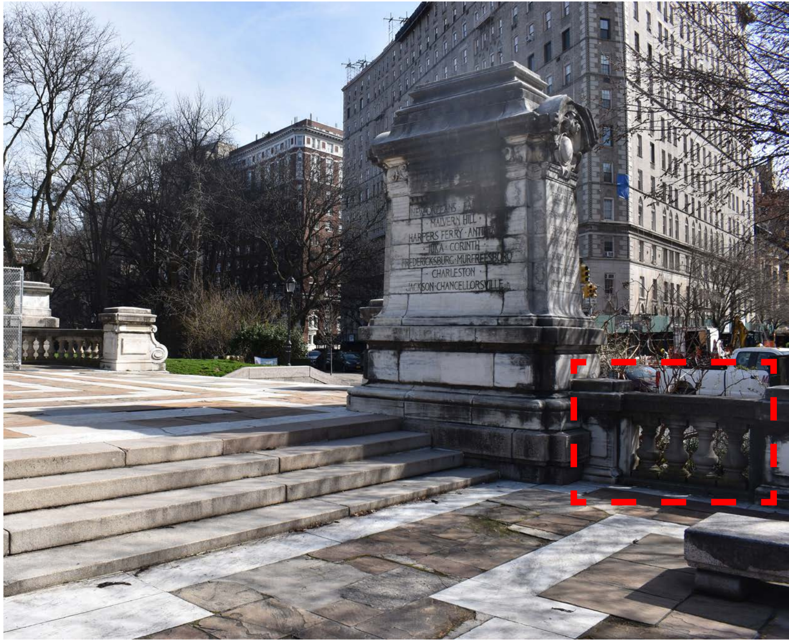
1962 Balustrade components to be removed and salvaged for use where needed in monument restoration
