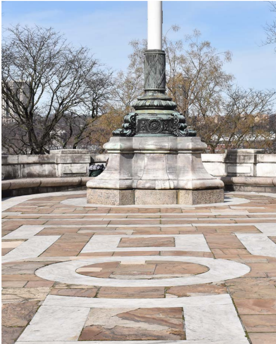
Terrace Reconstruction & Repaving — Rebuild sub-grade assembly — Install new drainage — Reset & replace existing materials
