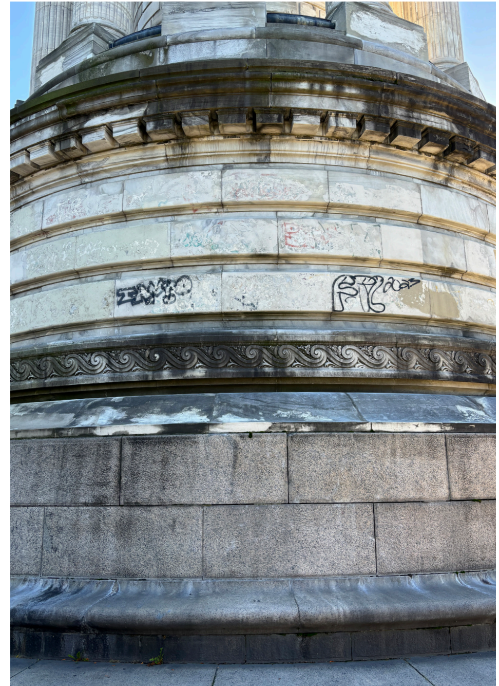
3— Deterioration of masonry elements
