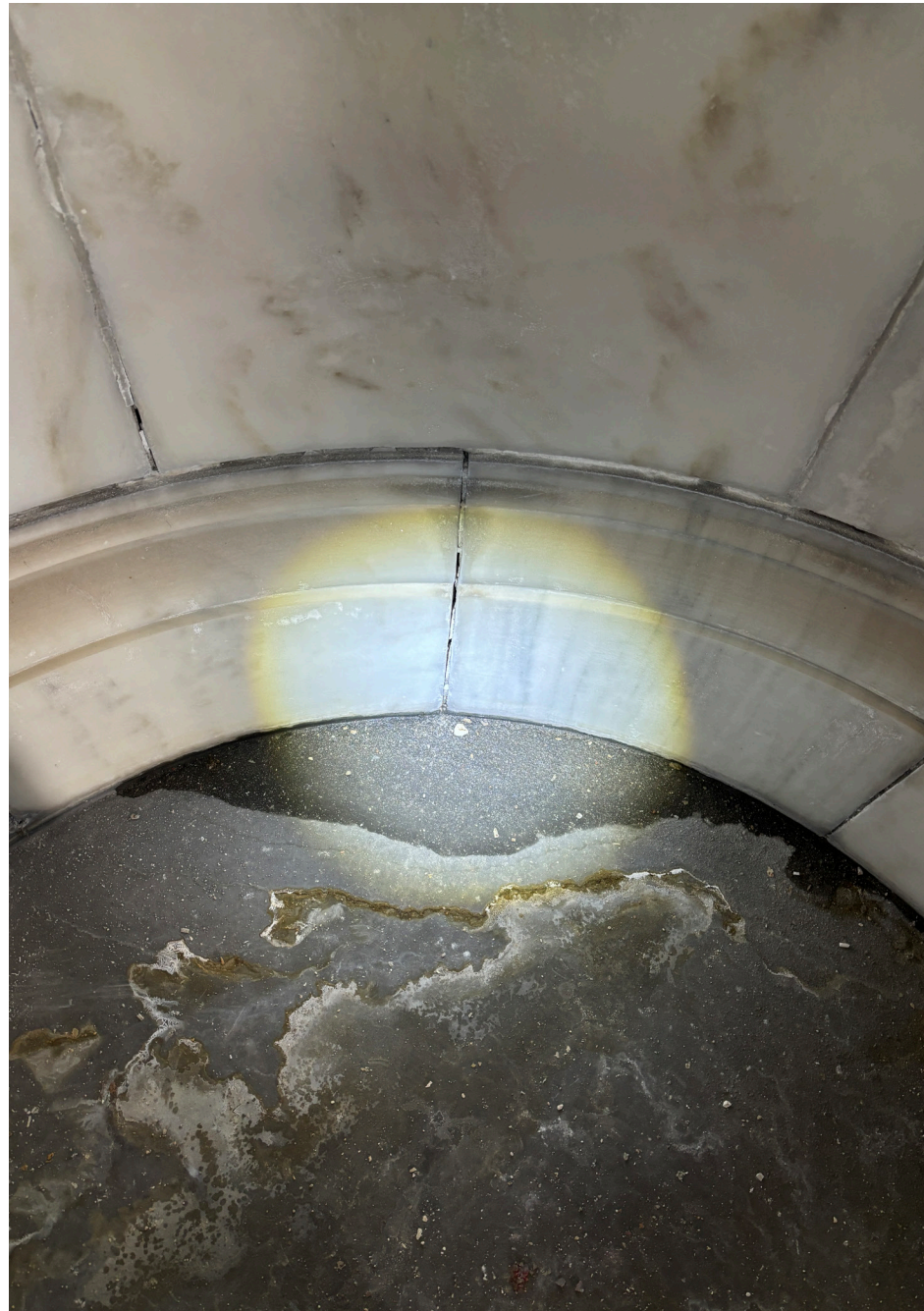
2— Evidence of water intrusion & damage
