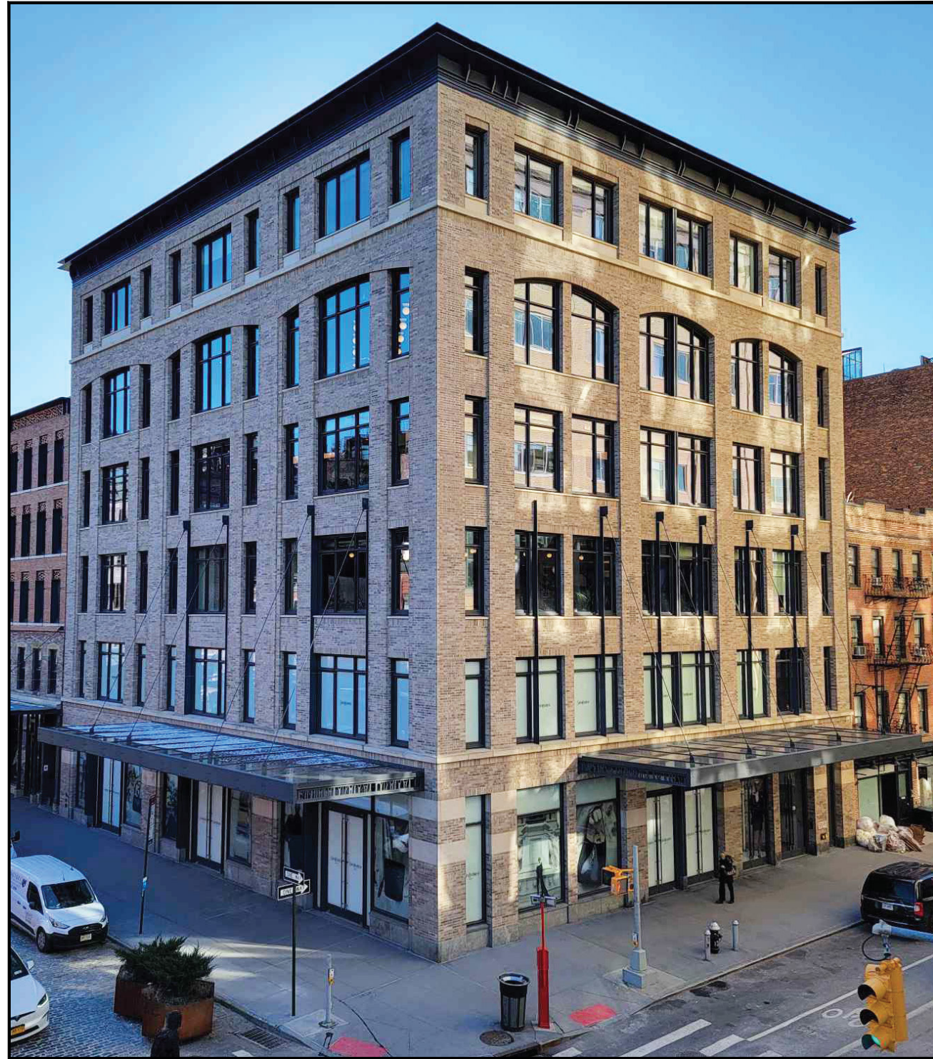
EXISTING FACADE - VIEW FROM NORTH OF GANSEVOORT STREET AND WASHINGTON STREET
