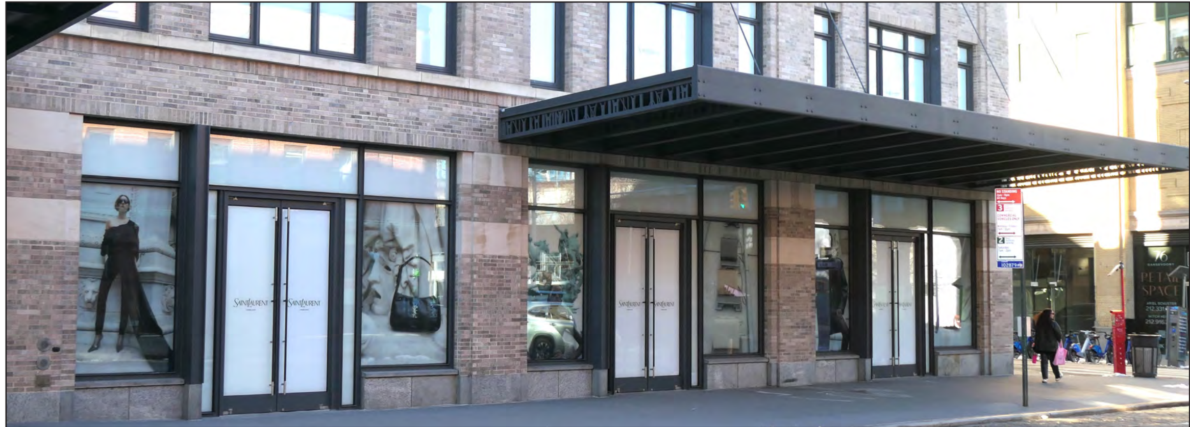
GANSEVOORT STREET FACADE - EXISTING CONDITION
