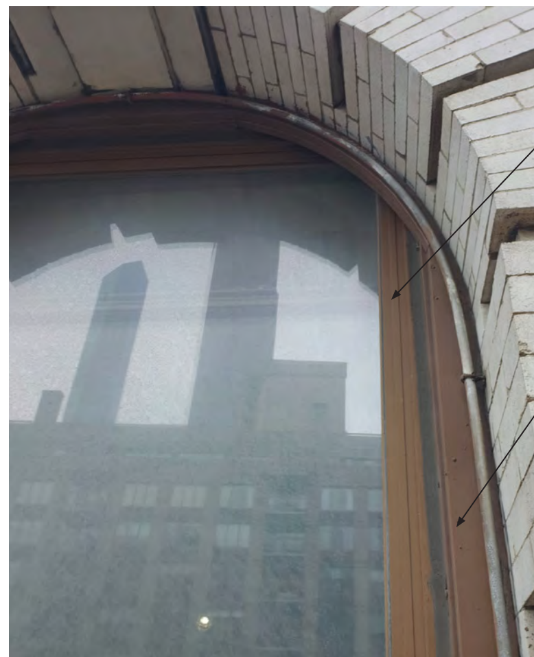
① HEAD DETAIL - EXISTING 2004 DOUBLE HUNG WINDOW
