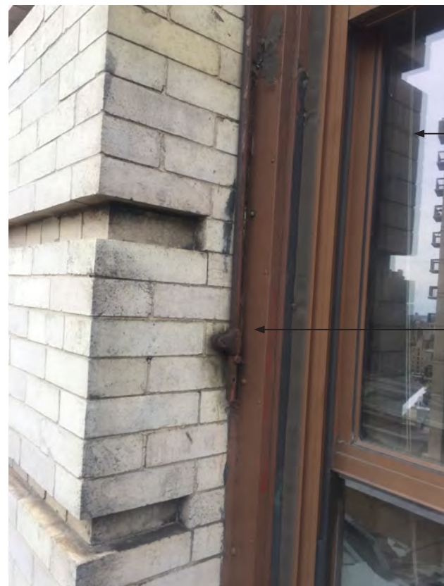
② JAMB DETAIL - EXISTING 2004 DOUBLE HUNG WINDOW
