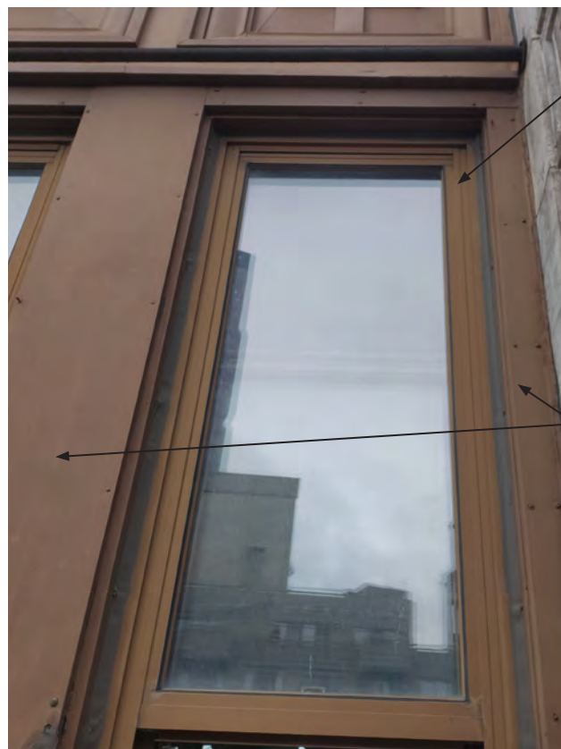
① HEAD DETAIL - EXISTING 2004 DOUBLE HUNG WINDOW
