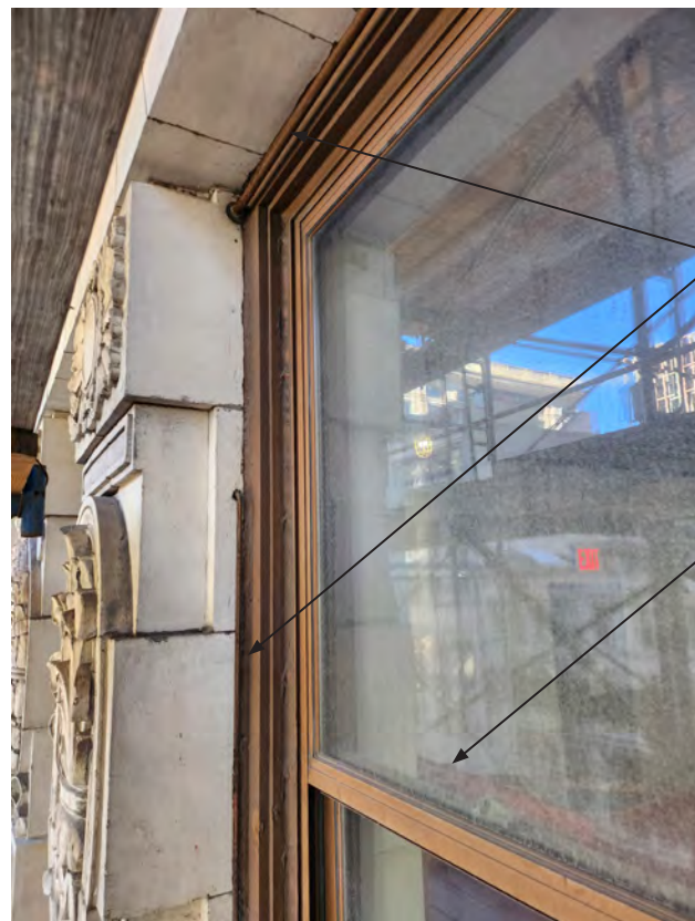
① HEAD DETAIL - EXISTING 2004 DOUBLE HUNG WINDOW
