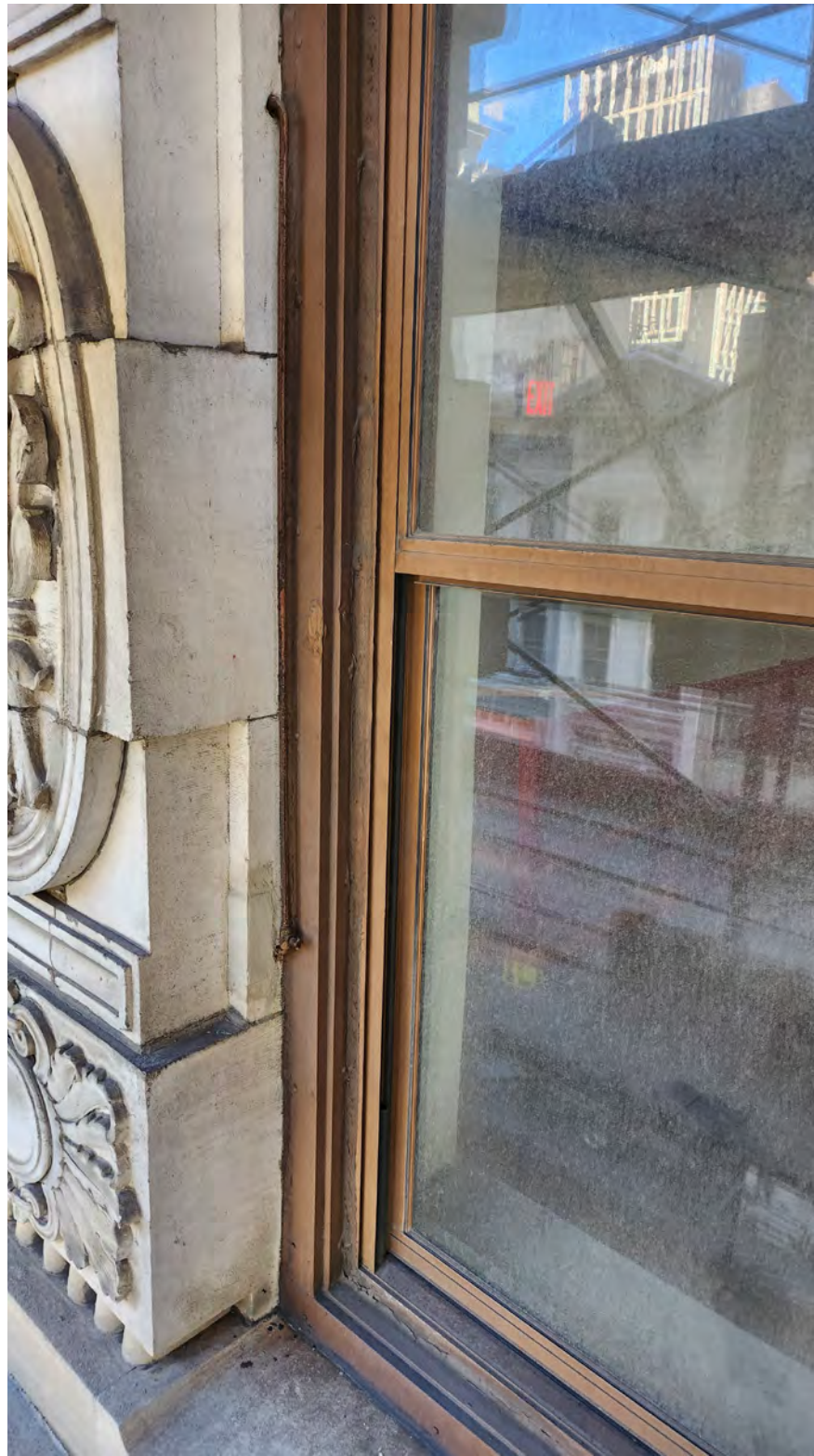
Ⓐ TYPICAL WINDOW PHOTO - 2004 DOUBLE HUNG ALUMINIUM WINDOW REPLACEMENT
