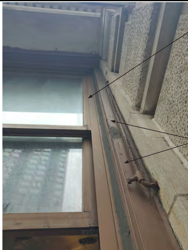
① HEAD DETAIL - EXISTING 2004 DOUBLE HUNG WINDOW
