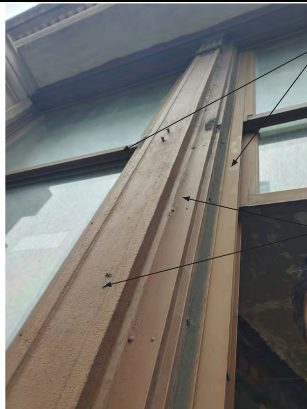
② JAMB DETAIL - EXISTING 2004 DOUBLE HUNG WINDOW
