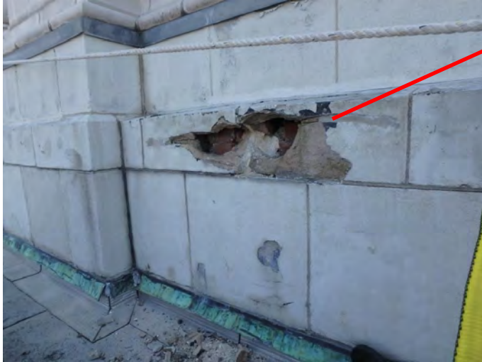
PHOTO # 1: West Elevation Main Roof Close-up photo of main roof spalled terracotta.
