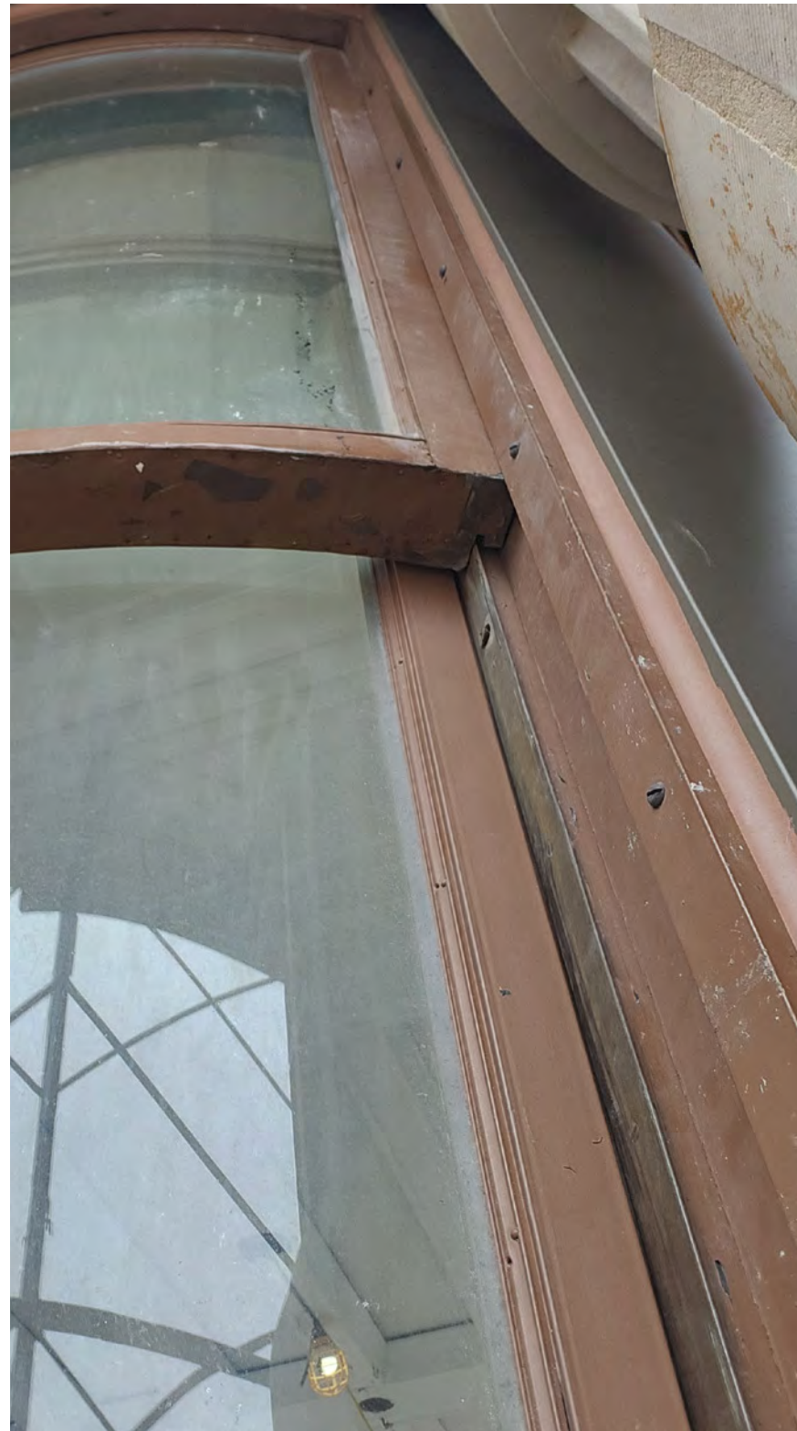
Ⓑ TYPICAL WINDOW PHOTO - 1902 ORIGINAL DOUBLE HUNG WINDOW
