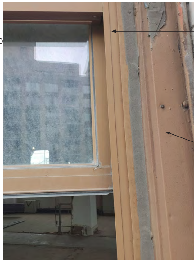
② JAMB DETAIL - EXISTING 2004 DOUBLE HUNG WINDOW
