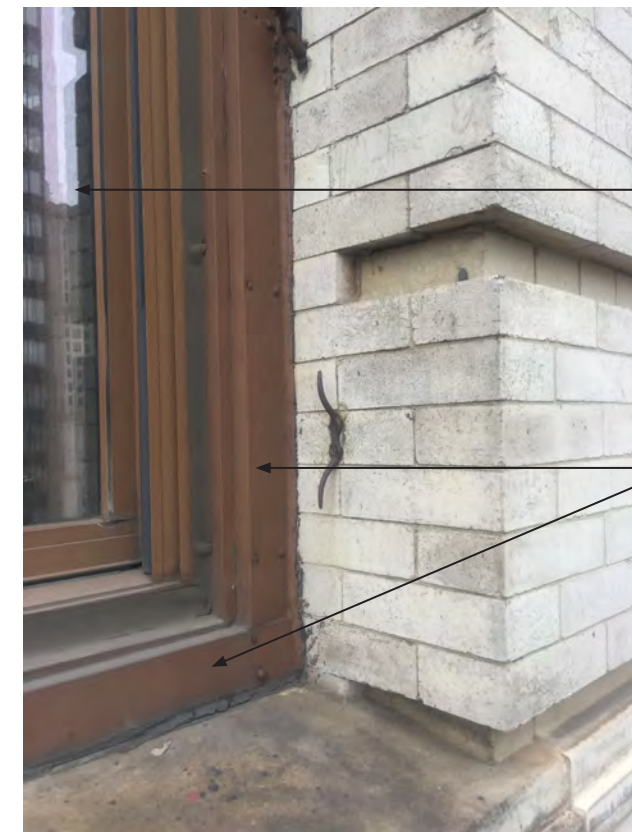
③ SILL DETAIL - EXISTING 2004 DOUBLE HUNG WINDOW
