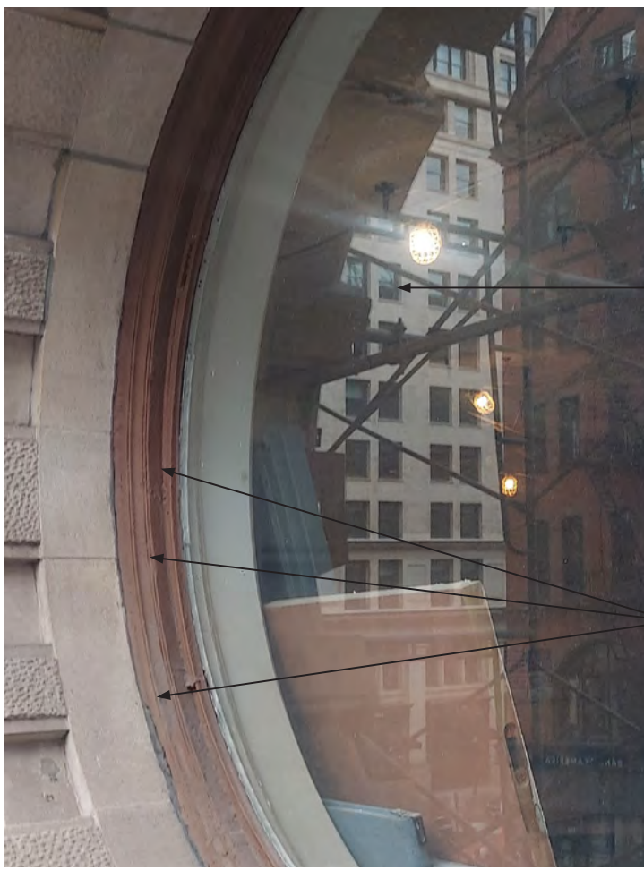
TYPE E - 1902 ROUND FIXED WINDOW TO BE REFURBISHED.
