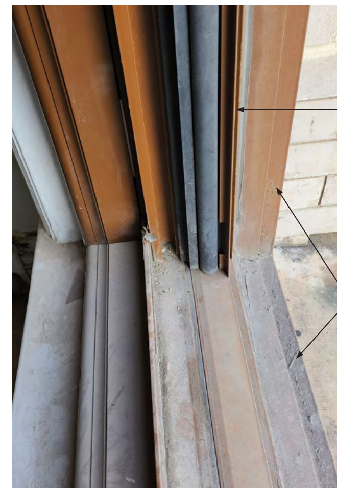
③ SILL DETAIL - EXISTING 2004 DOUBLE HUNG WINDOW
