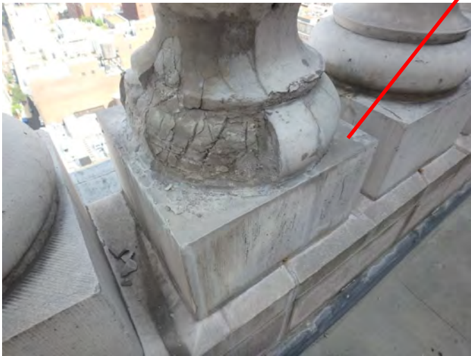
PHOTO # 2: West Elevation Main Roof Close-up photo of spalled precast balustrade at perimeter of main roof. Photos by CANY
