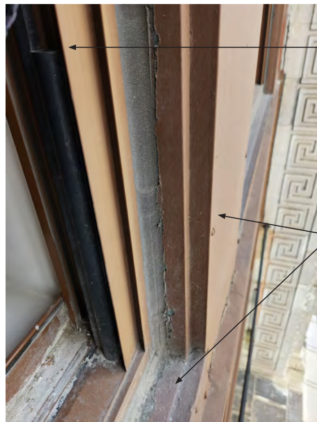
② JAMB DETAIL - EXISTING 2004 DOUBLE HUNG WINDOW
