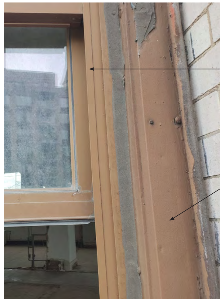
② JAMB DETAIL - EXISTING 2004 DOUBLE HUNG WINDOW
