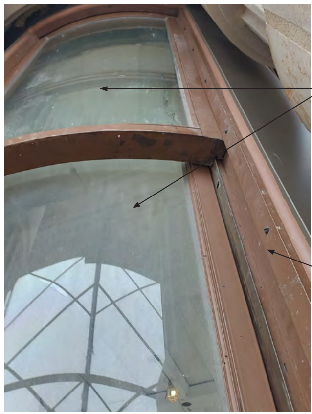
TYPE A - 1902 CURVED DOUBLE HUNG WINDOW TO BE REFURBISHED.
