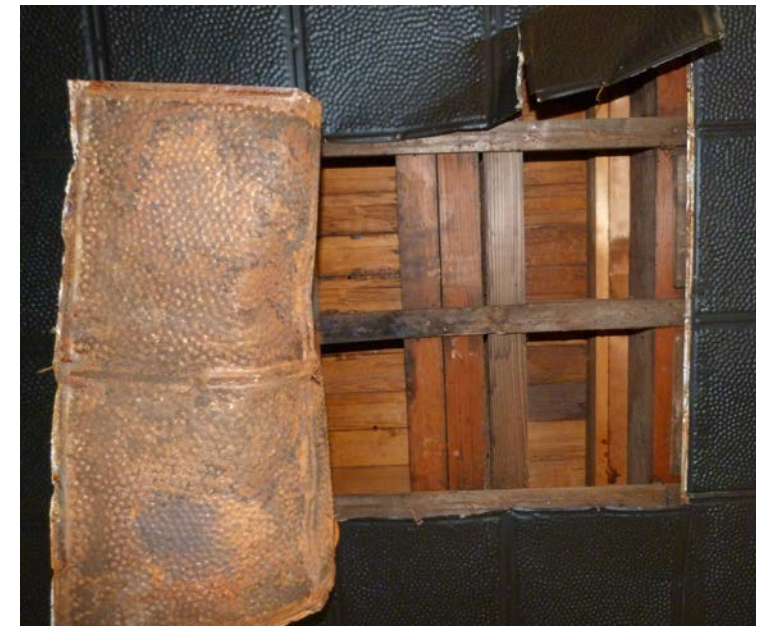
301 Canal Street Second floor structure showing non-historic construction
