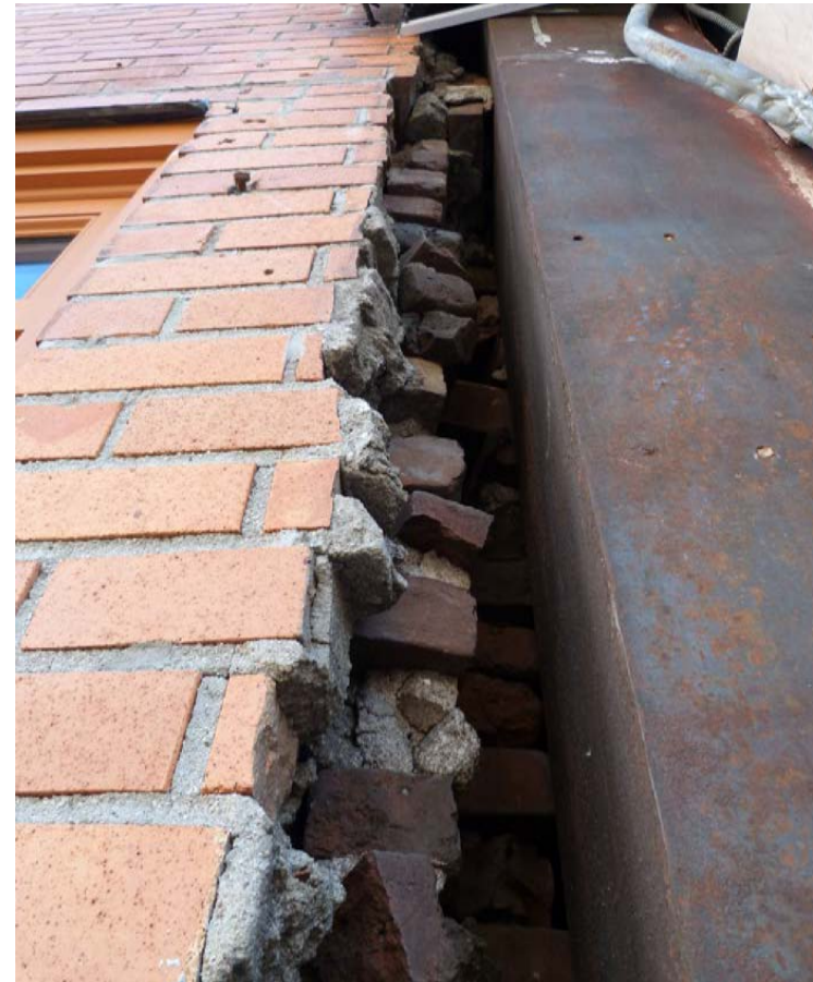
301 Canal Street East edge of exterior wall
