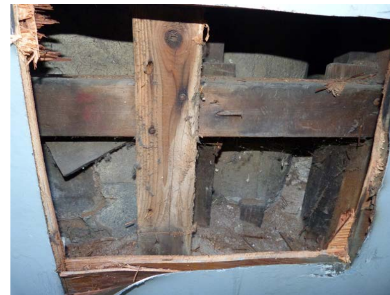
419 Broadway: concrete encased column at Canal Street elevation
