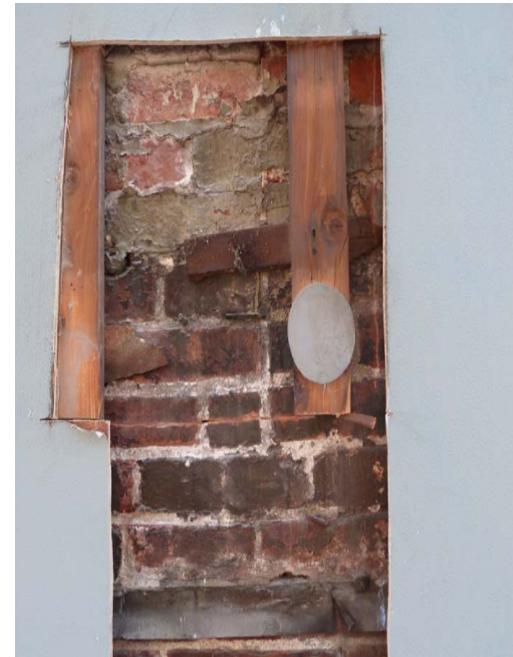
419 Broadway: brick spandrel at Canal Street elevation
