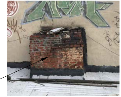
PHOTO OF EXISTING BRICK CHIMNEY
