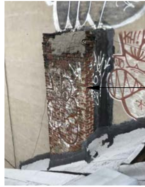
PHOTO OF EXISTING BRICK CHIMNEY
