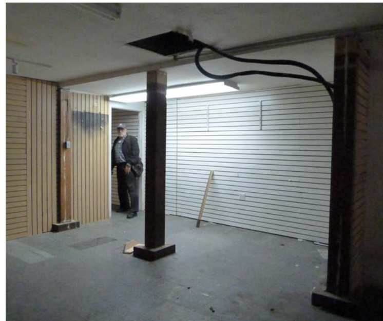
301 Canal Street Interior view showing steel columns, clad in wood, at 2nd story
