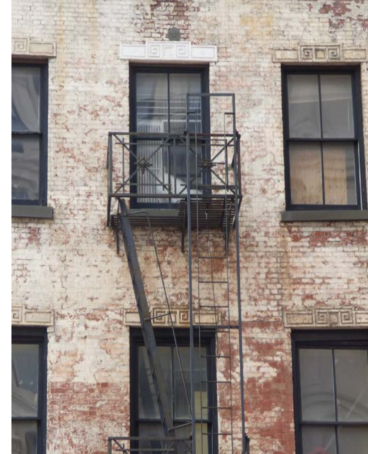
Central bay fire escape.
