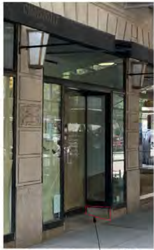
IMAGE 4 - JULY 2022 GRANITE BULKHEAD/CURB RETURNS TO BE REMOVED
