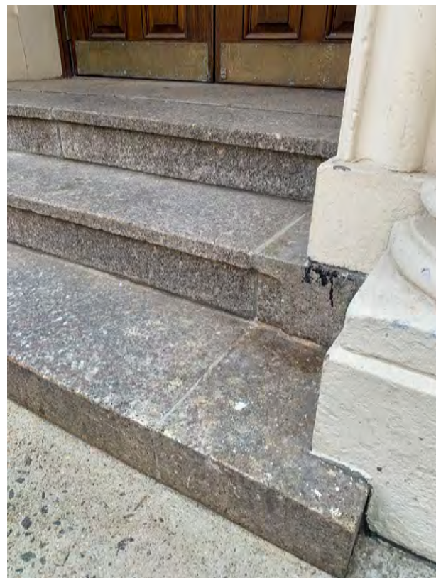
Front entrance steps detail
