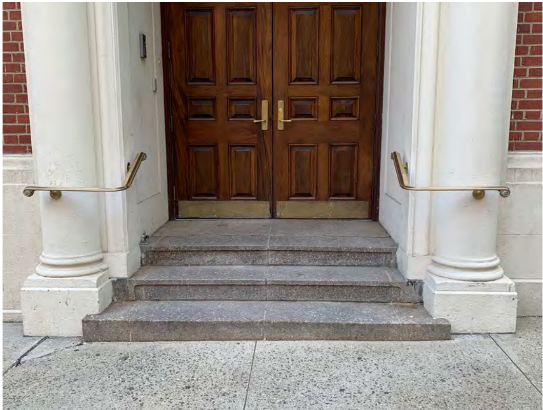
Front entrance steps, column and handrail
