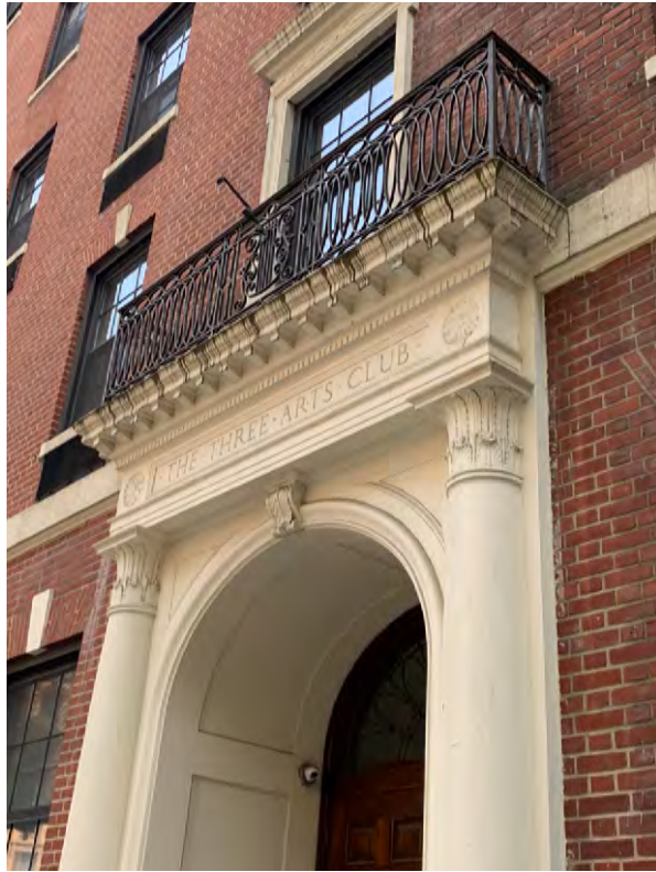
Front entrance archway and balconet
