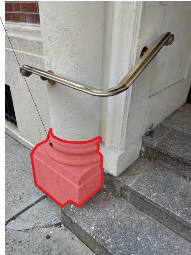
Front entrance steps, column and handrail
