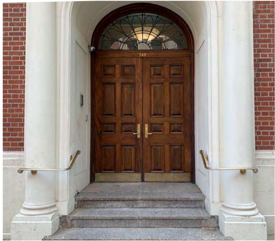
Front entrance door
