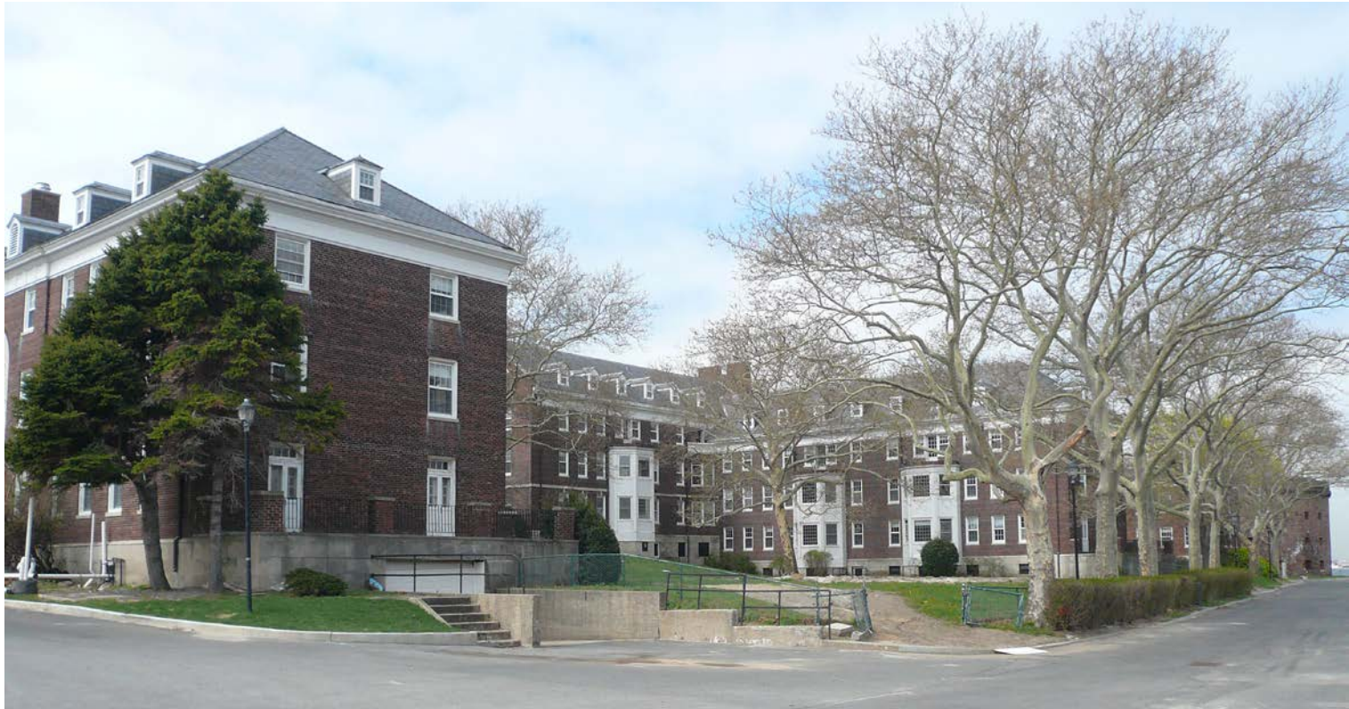
VIEW OF BUILDINGS 111 AND 112, LOOKING SOUTHWEST FROM CARDER ROAD
