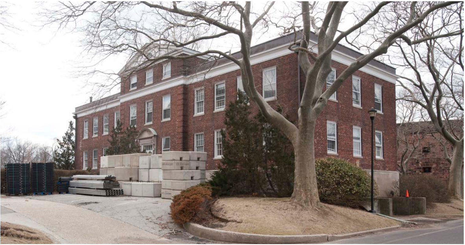
VIEW, LOOKING SOUTHWEST FROM CARDERROAD
