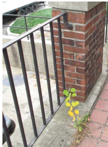
EXISTING TERRACE RAILING
