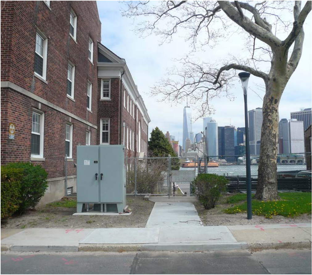
VIEW AA: BUILDING 111 AS SEEN FROM ANDES ROAD
