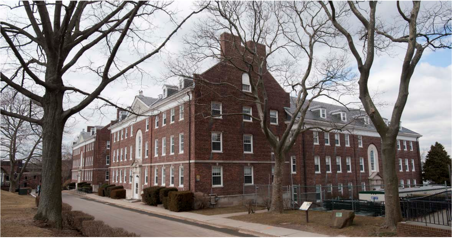
VIEW, LOOKING NORTHWEST FROM ANDES ROAD
