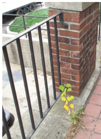
EXISTING TERRACE RAILING
