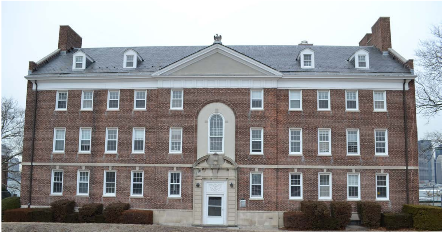
FRONT FACADE FROM ANDES ROAD
