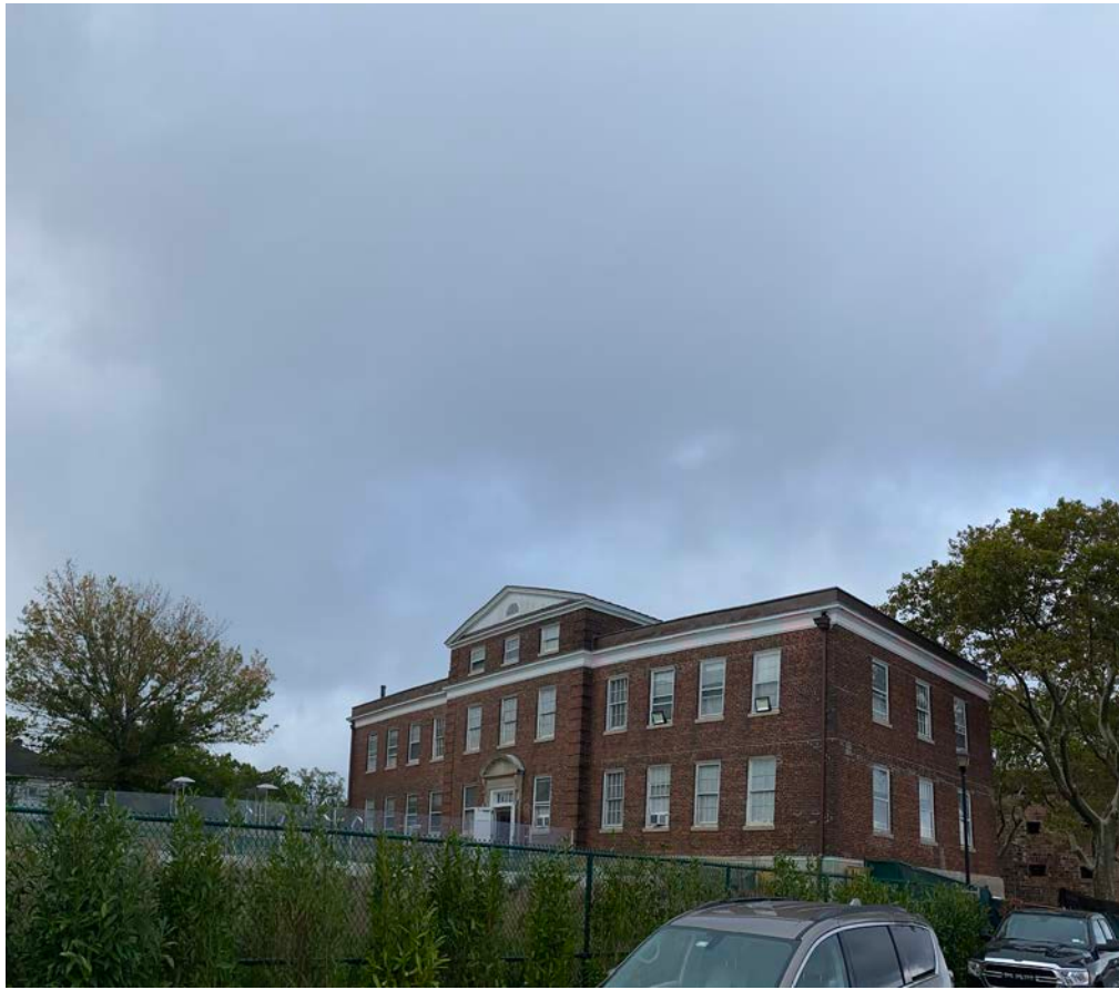
VIEW CC: BUILDING 114 AS SEEN FROM CARDER ROAD
