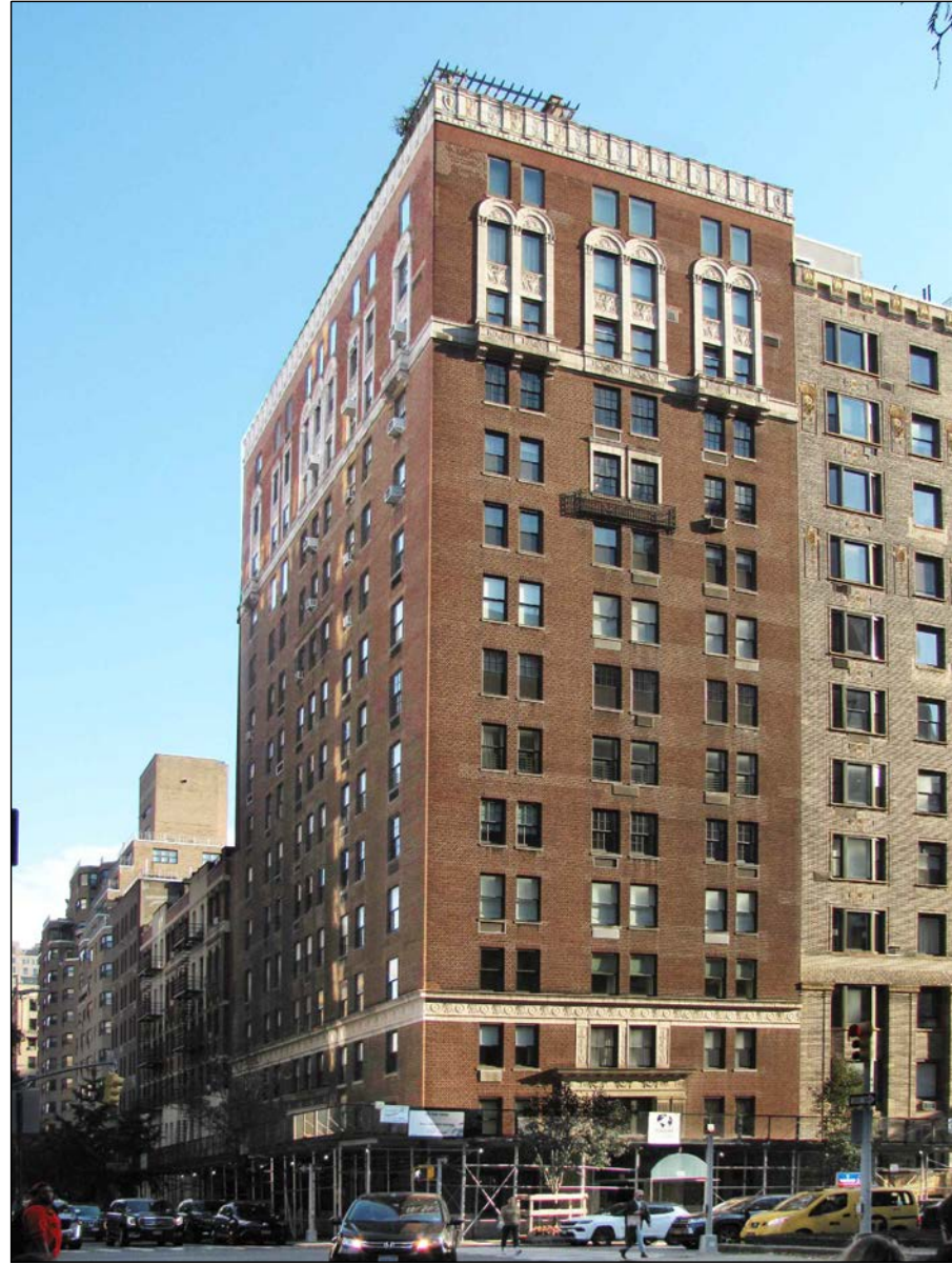
E 81st STREET VIEW C EXISTING CONDITION
