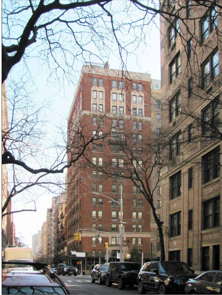
E 81st STREET VIEW B EXISTING CONDITION
