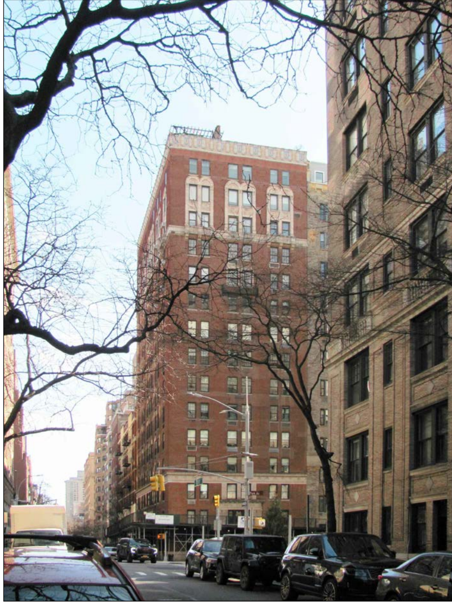
E 81st STREET VIEW B EXISTING CONDITION
