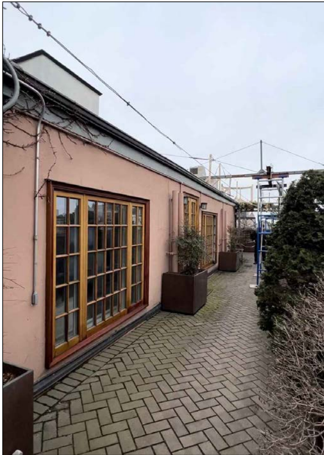
LOWER TERRACE ROOF
