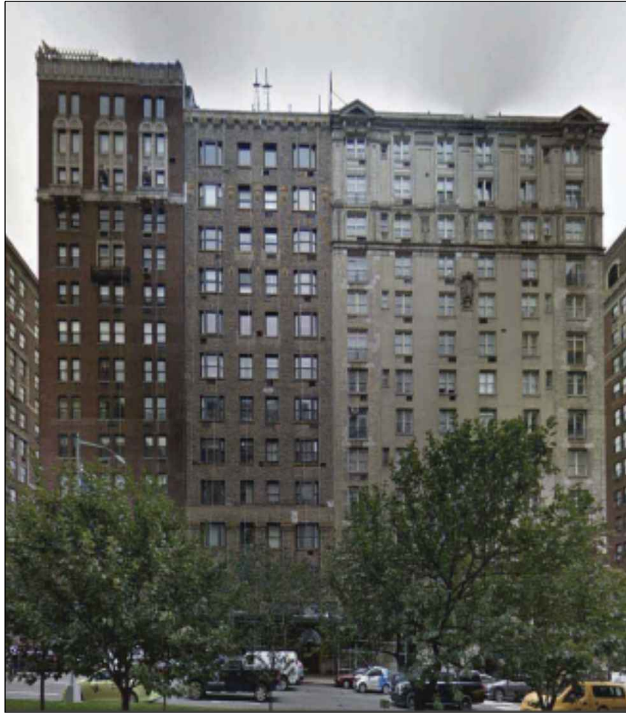
935 PARK AVE & ADJACENT BUILDINGS ALONG PARK AVE
