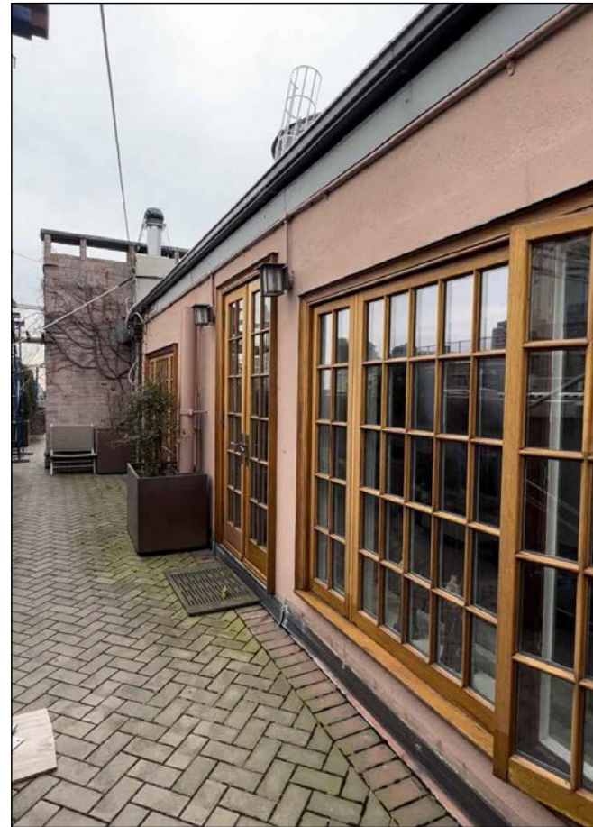
LOWER TERRACE ROOF
