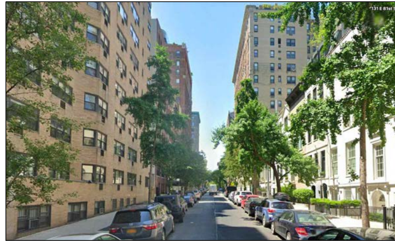
VIEW WEST ON 81ST STREET
