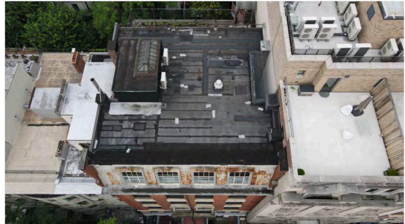
[FIGURE 2] EXISTING BUILDING ROOF TOP BIRDS EYE VIEW SOUTH
