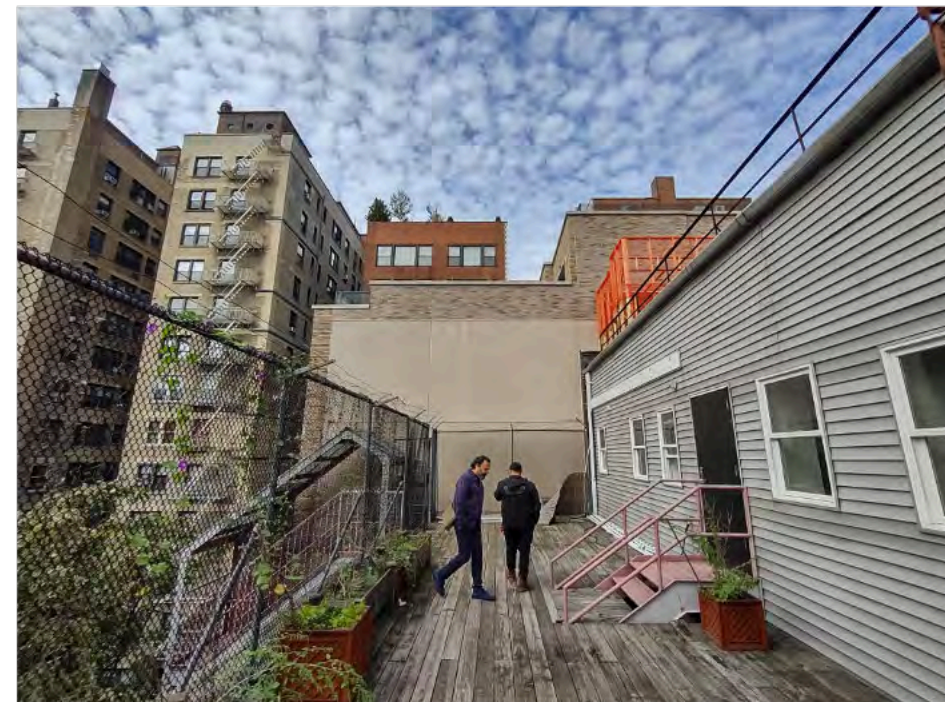
[4] TOP REAR [5TH FLOOR] TERRACE FACADE LOOKING WEST
