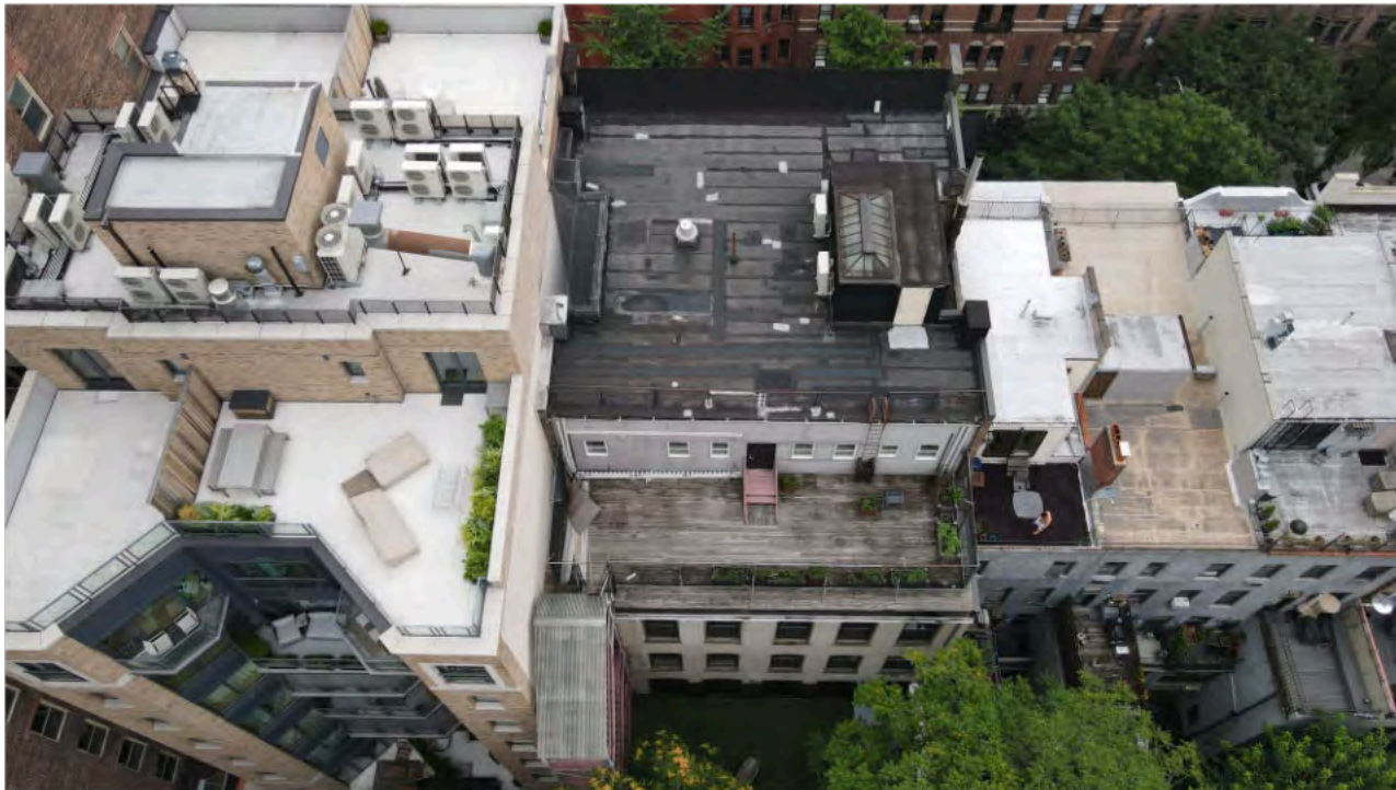
[FIGURE 1] EXISTING BUILDING ROOF TOP BIRDS EYE VIEW NORTH
