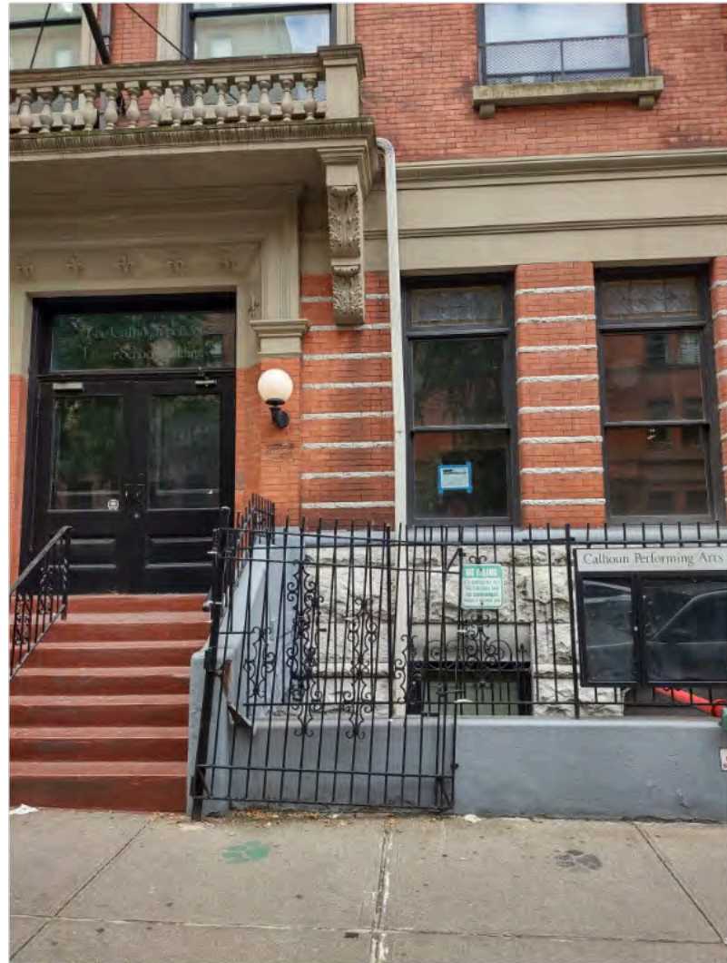
EXISTING AREAWAY PHOTO DATED (10-12-2023)
