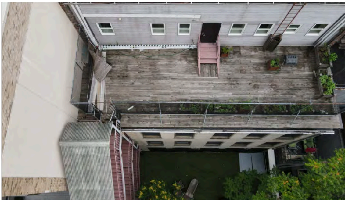
[FIGURE 3] EXISTING BUILDING 4TH FLOOR BIRDS EYE VIEW SOUTH
