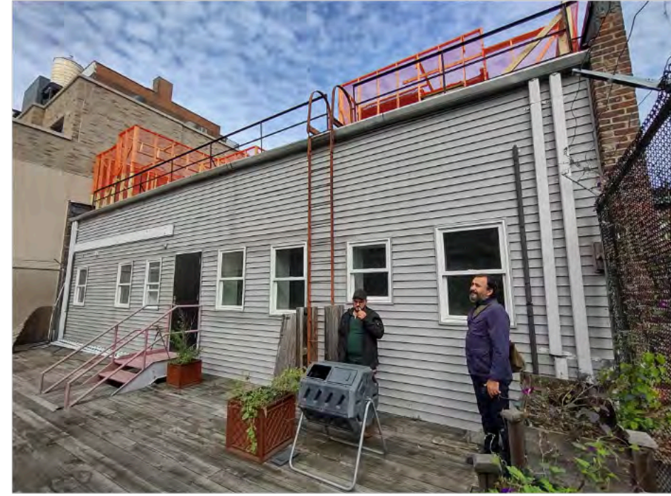
[3] TOP REAR [5TH FLOOR] TERRACE FACADE
