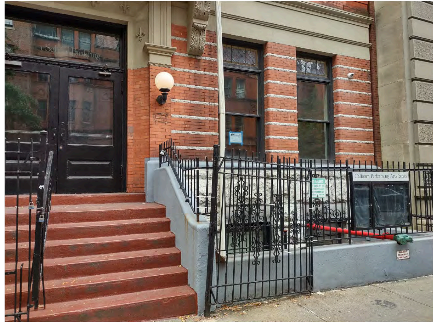
EXISTING AREAWAY PHOTO DATED (10-12-2023)
