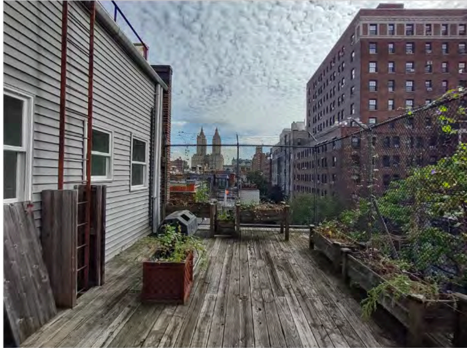
[5] TOP REAR [5TH FLOOR] TERRACE FACADE LOOKING EAST
