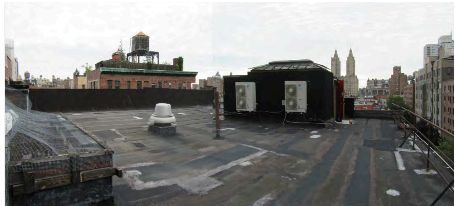
[FIGURE 4] EXISTING BUILDING ROOF TOP VIEW LOOKING WEST
