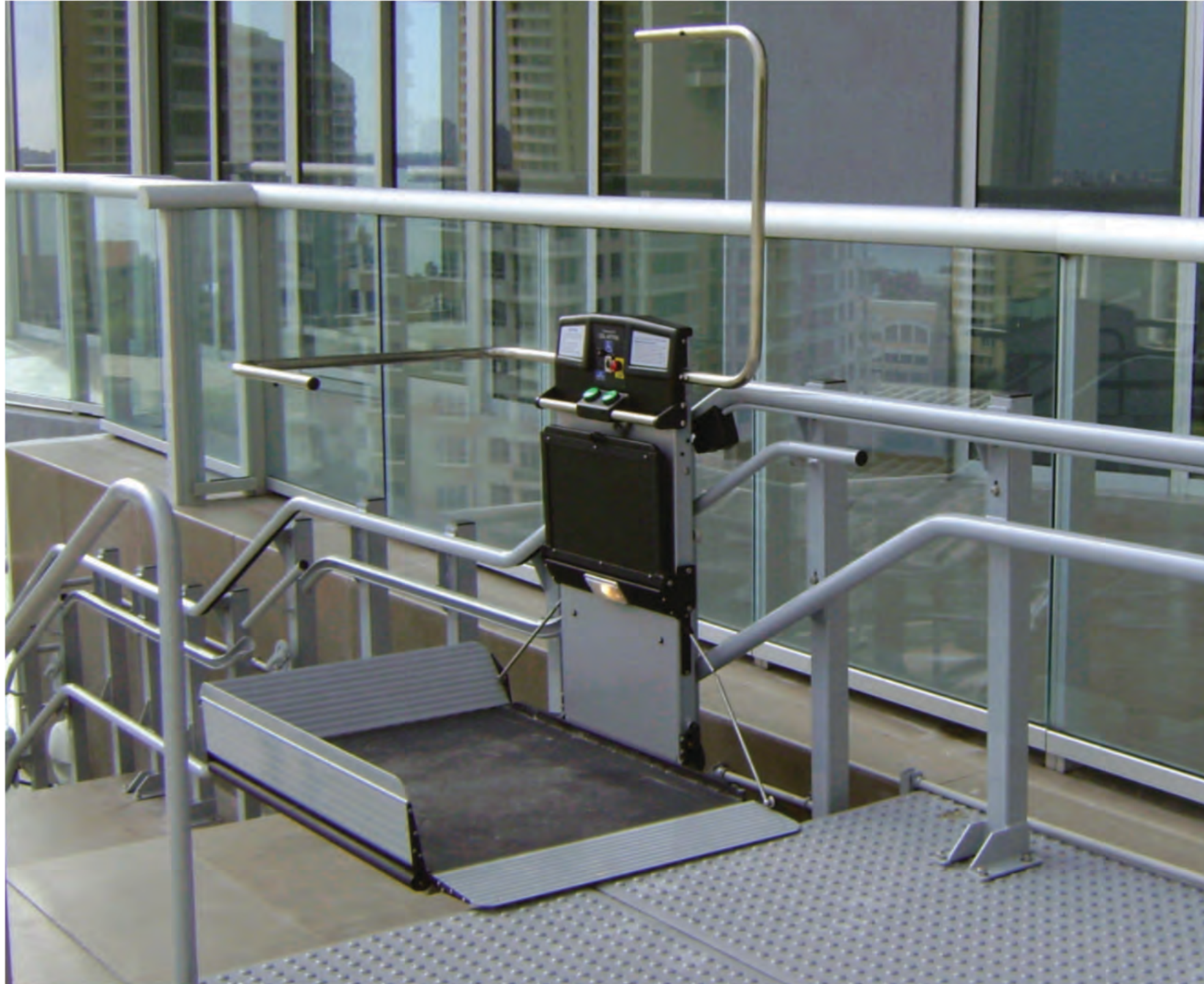
BASIS OF DESIGN : ARTIRA STAIR LIFT BY GARAVENTA LIFT
