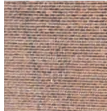
EXISTING BRICK COLOR SIDE FACADE
