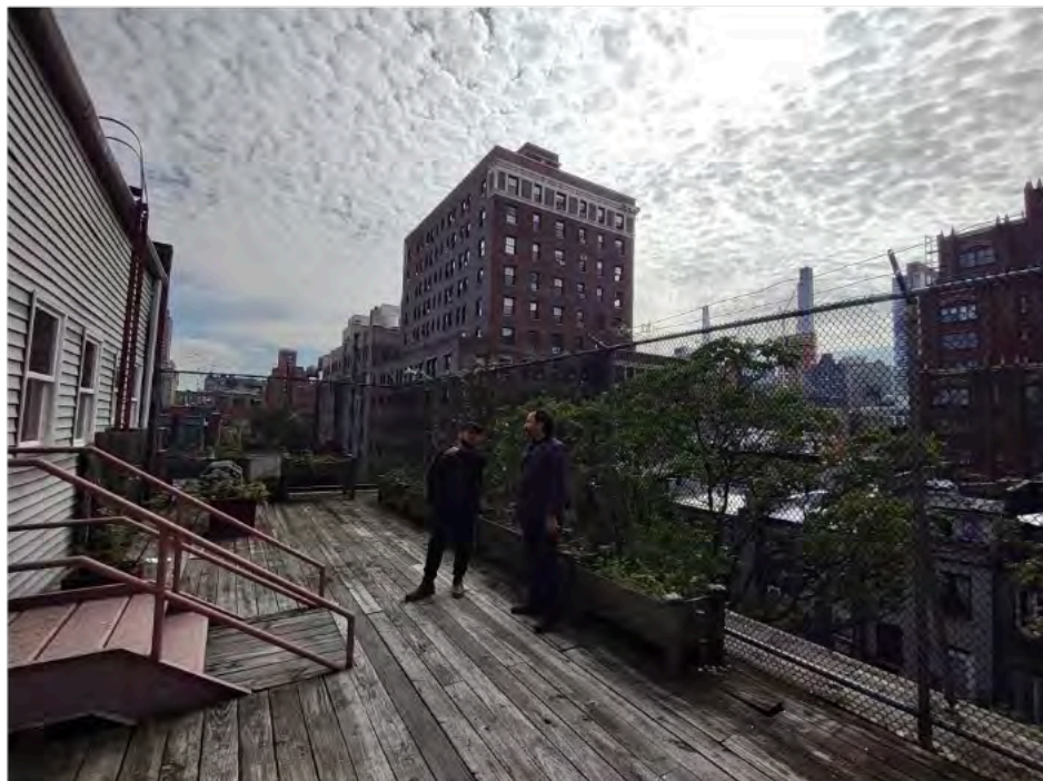
[6] TOP REAR [5TH FLOOR] TERRACE FACADE LOOKING SOUTH-EAST
