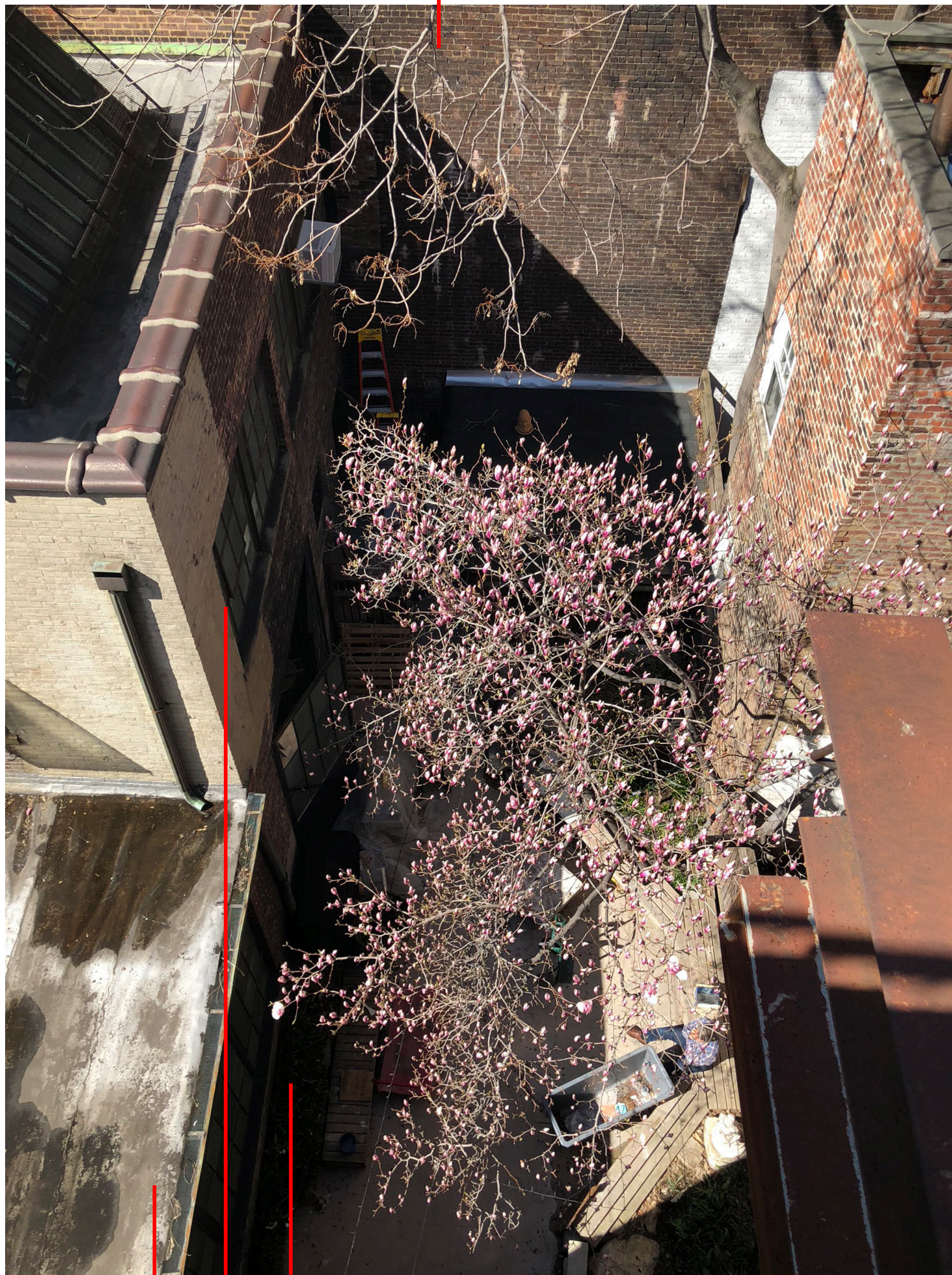
EXISTING REAR YARD EXISTING GREENWICH HOUSE (2 STORY BUILDING) EXISTING GREENWICH HOUSE (1 STORY BUILDING)
