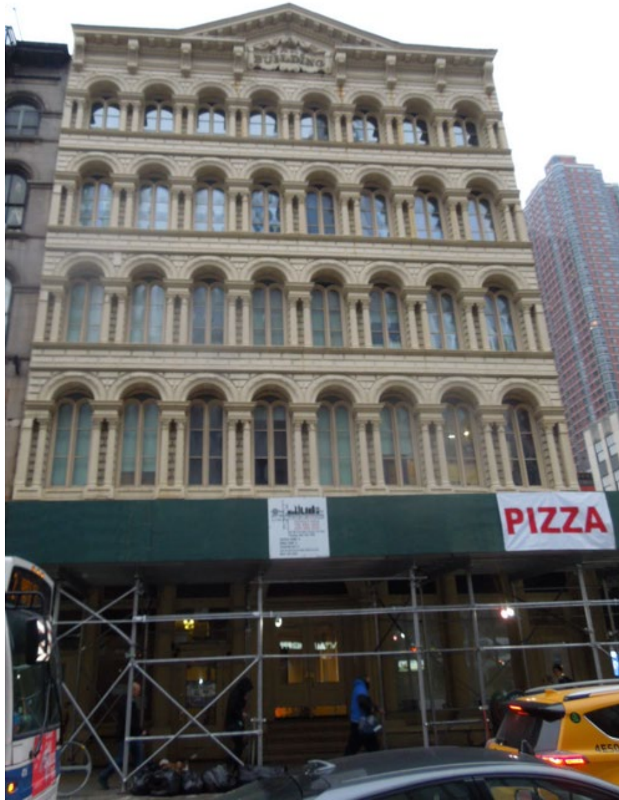
South Façade (Chambers St) - Existing Conditions
