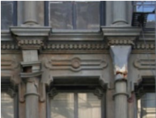
Before: Deteriorated cast iron capitals.
