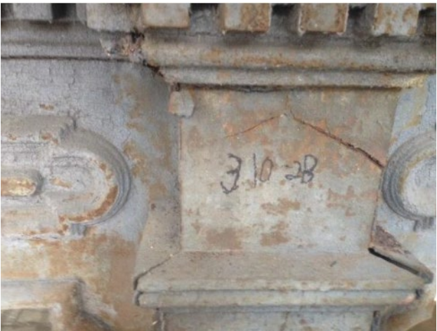
Before: Deteriorated cast iron capitals.
