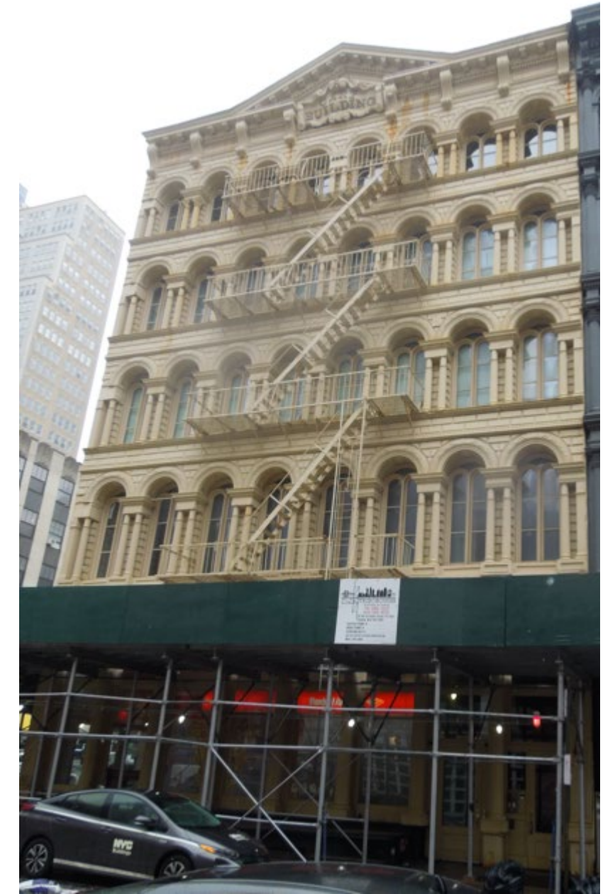
North Façade (Reade St) - Existing Conditions
