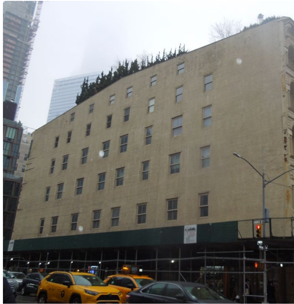
East Façade (Church St) - Existing Conditions
