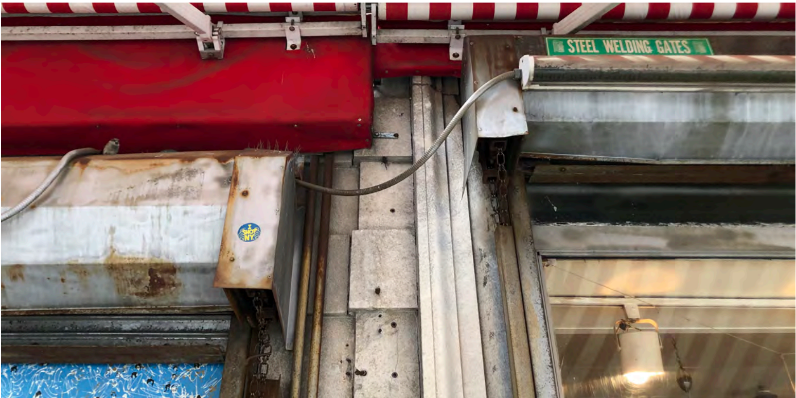
Photo of current state: outside lighting was an afterthought and electric installation is precarious.
