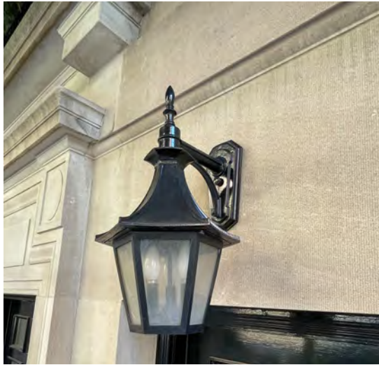
1. CURRENT LIGHT FIXTURES (NOT HISTORIC)
