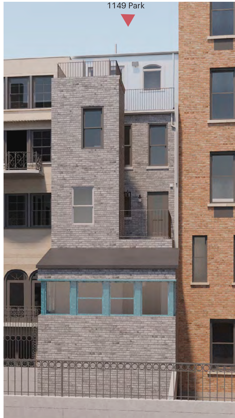
EXISTING REAR VIEW
