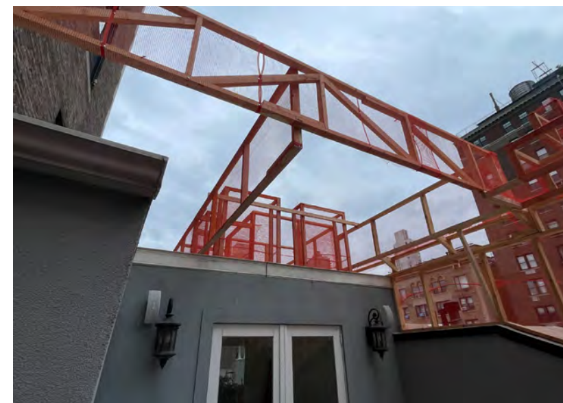
VIEW OF THE MOCK-UP FROM THE FRONT
