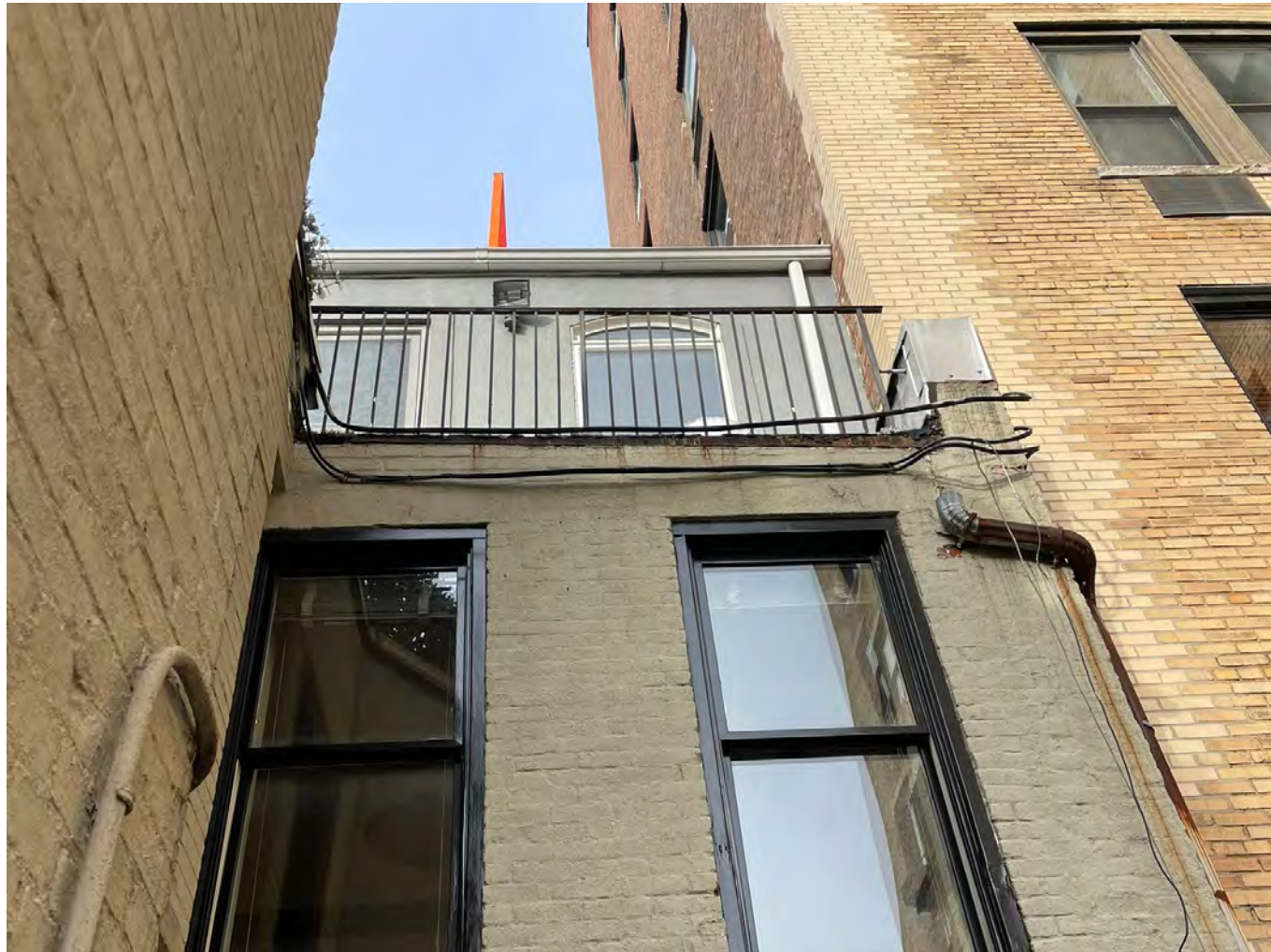
IMAGES OF THE REAR FACADE
