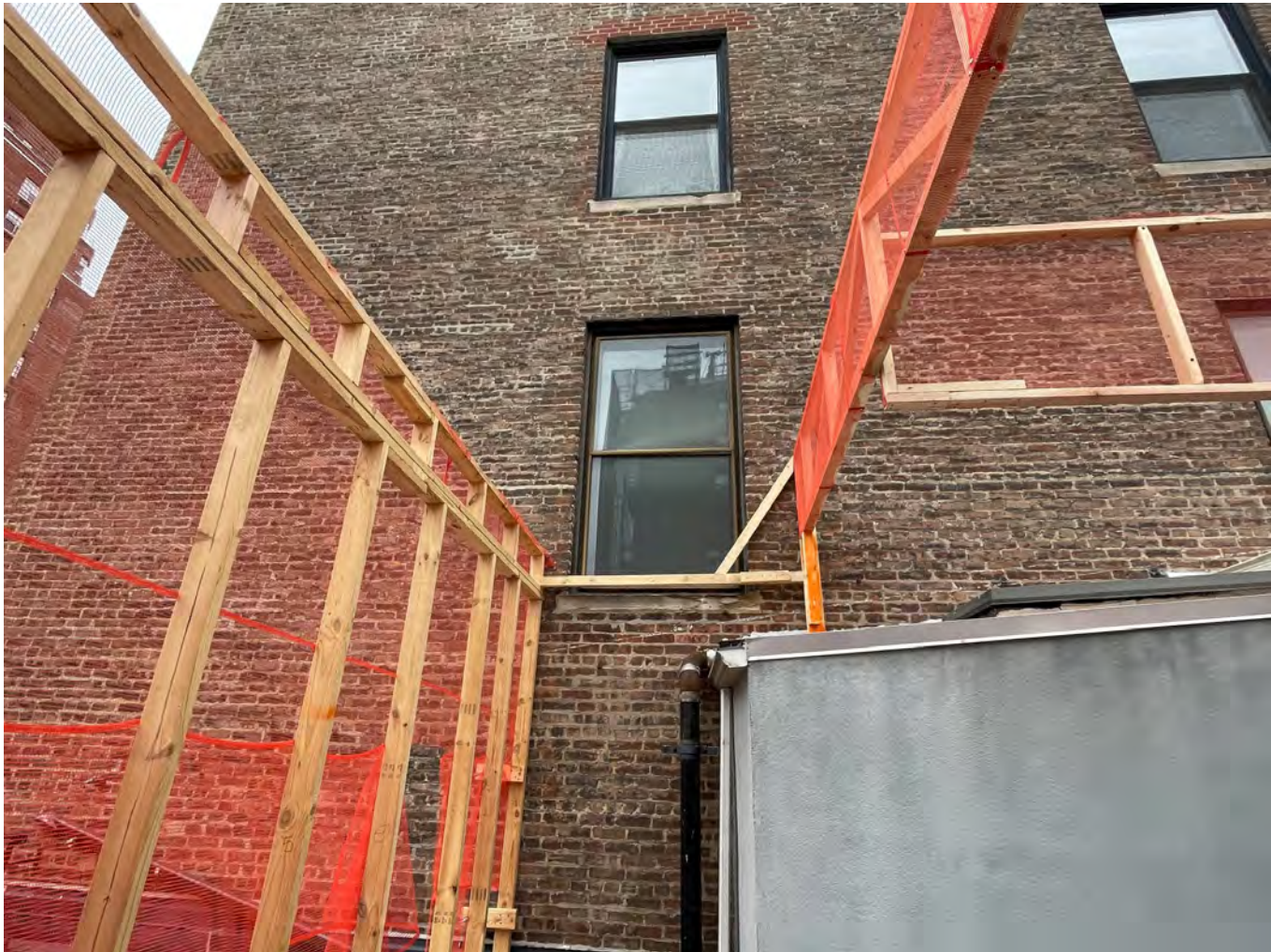
VIEW OF THE MOCK-UP FROM THE FRONT
