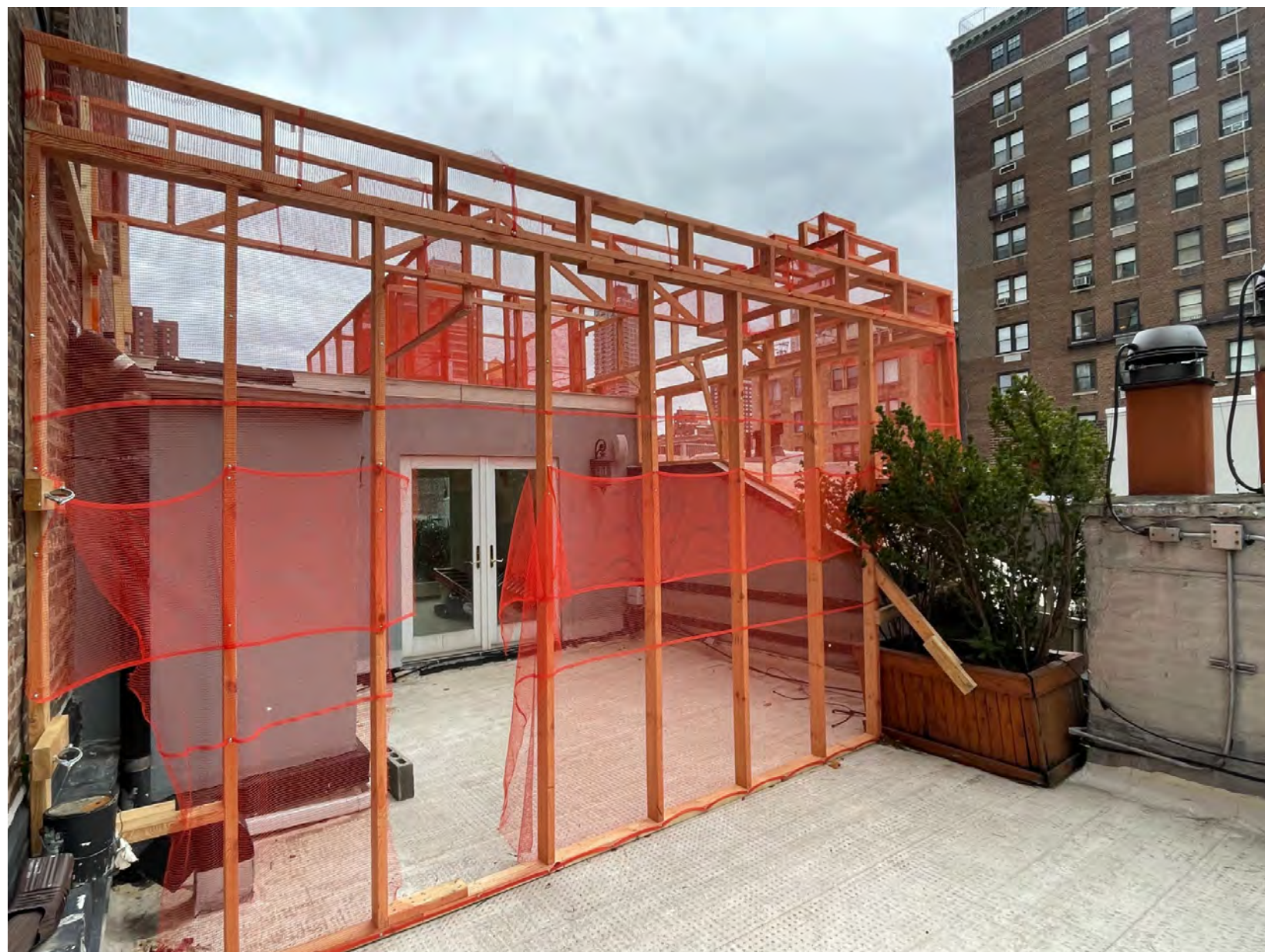
VIEW OF THE MOCK-UP FROM THE FRONT
