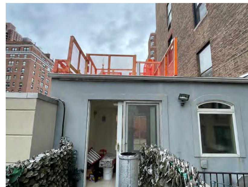
VIEW OF THE MOCK-UP FROM THE REAR
