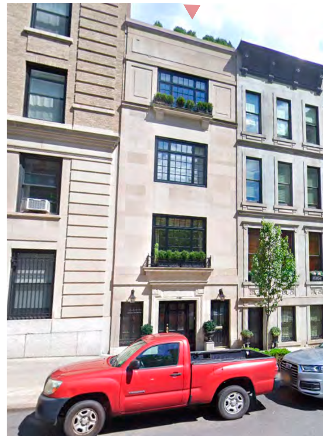
CURRENT STREET FACADE
