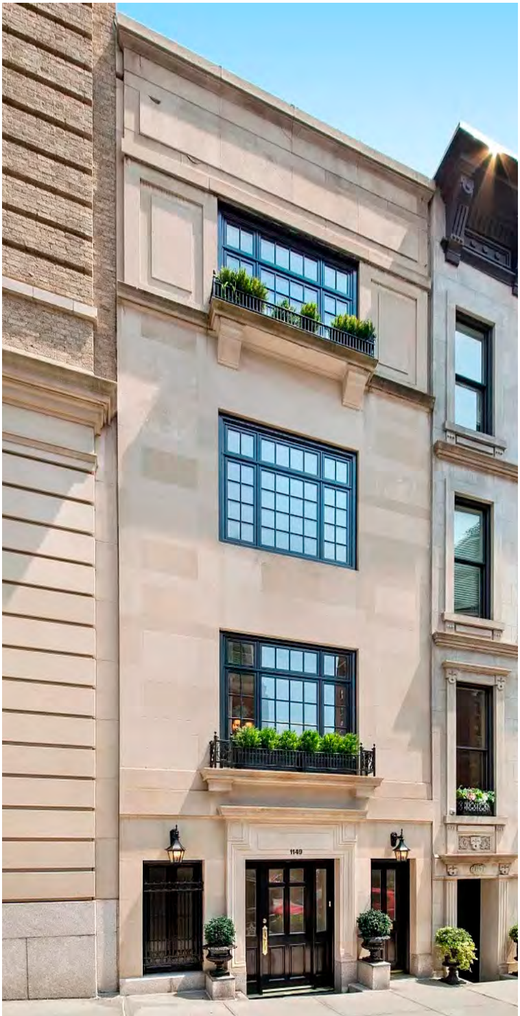
CURRENT STREET FACADE
