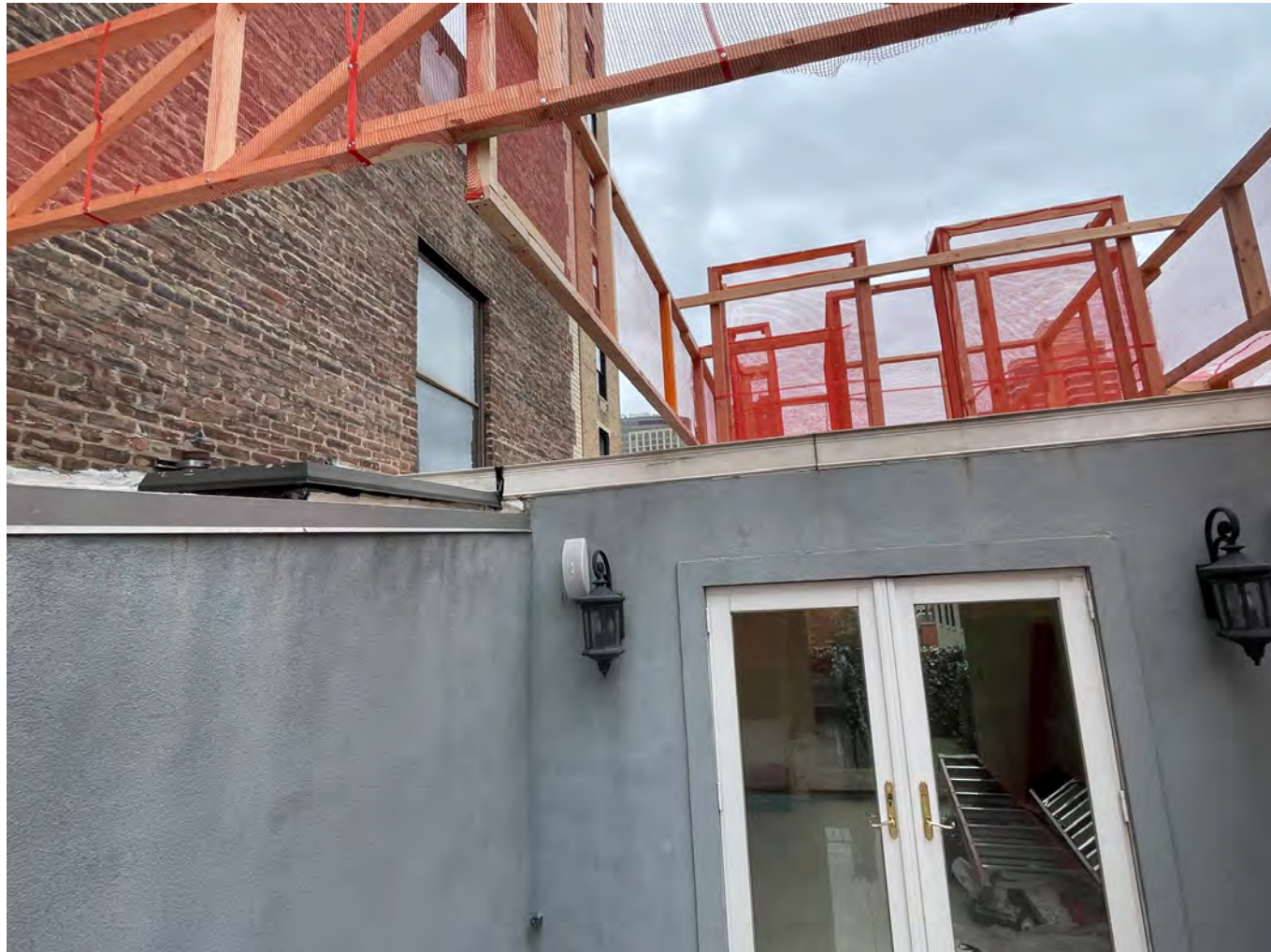
VIEW OF THE MOCK-UP FROM THE FRONT
