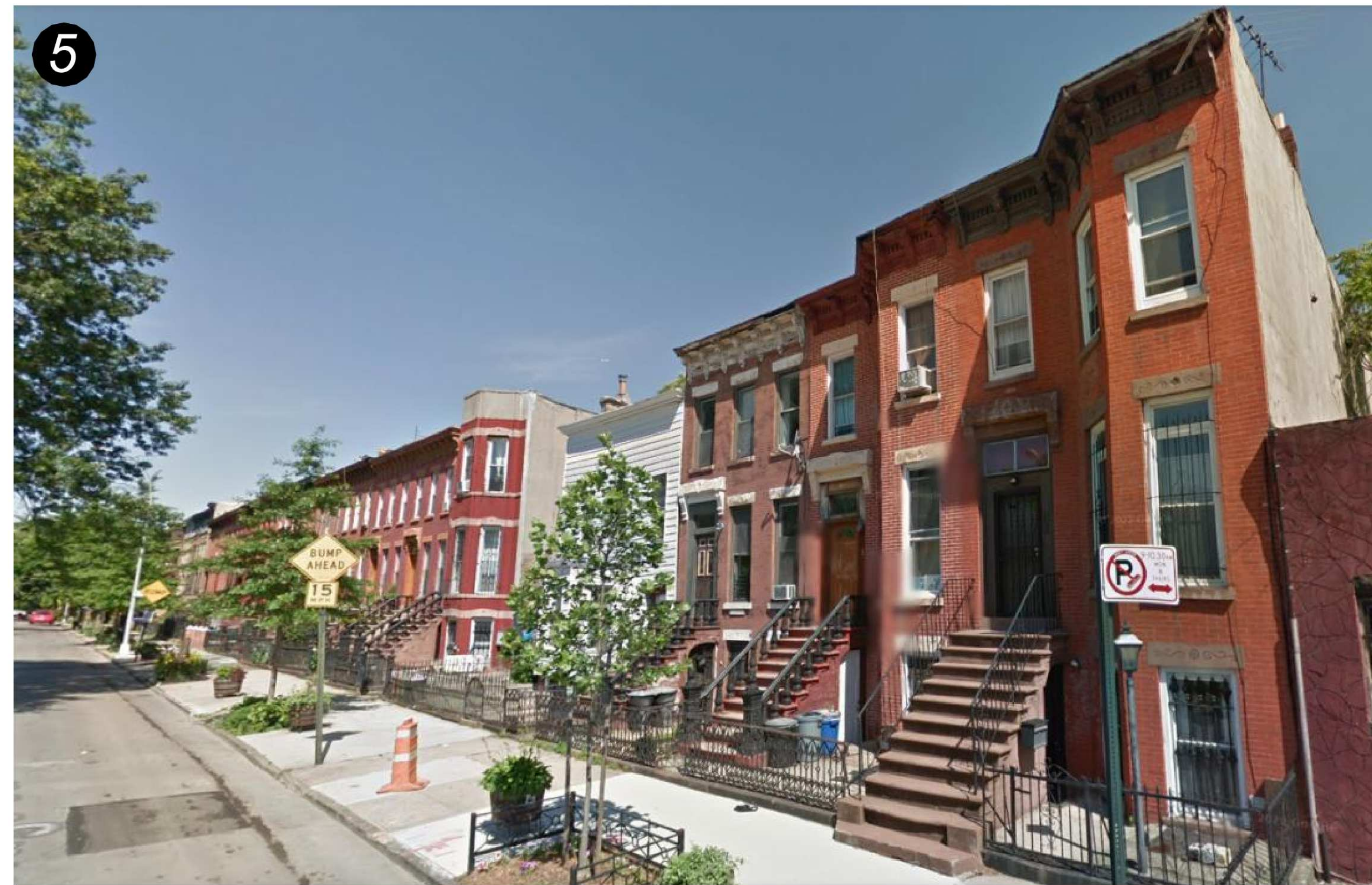
BAINBRIDGE STREET NORTH SIDE / TYPICAL ROW STYLE
