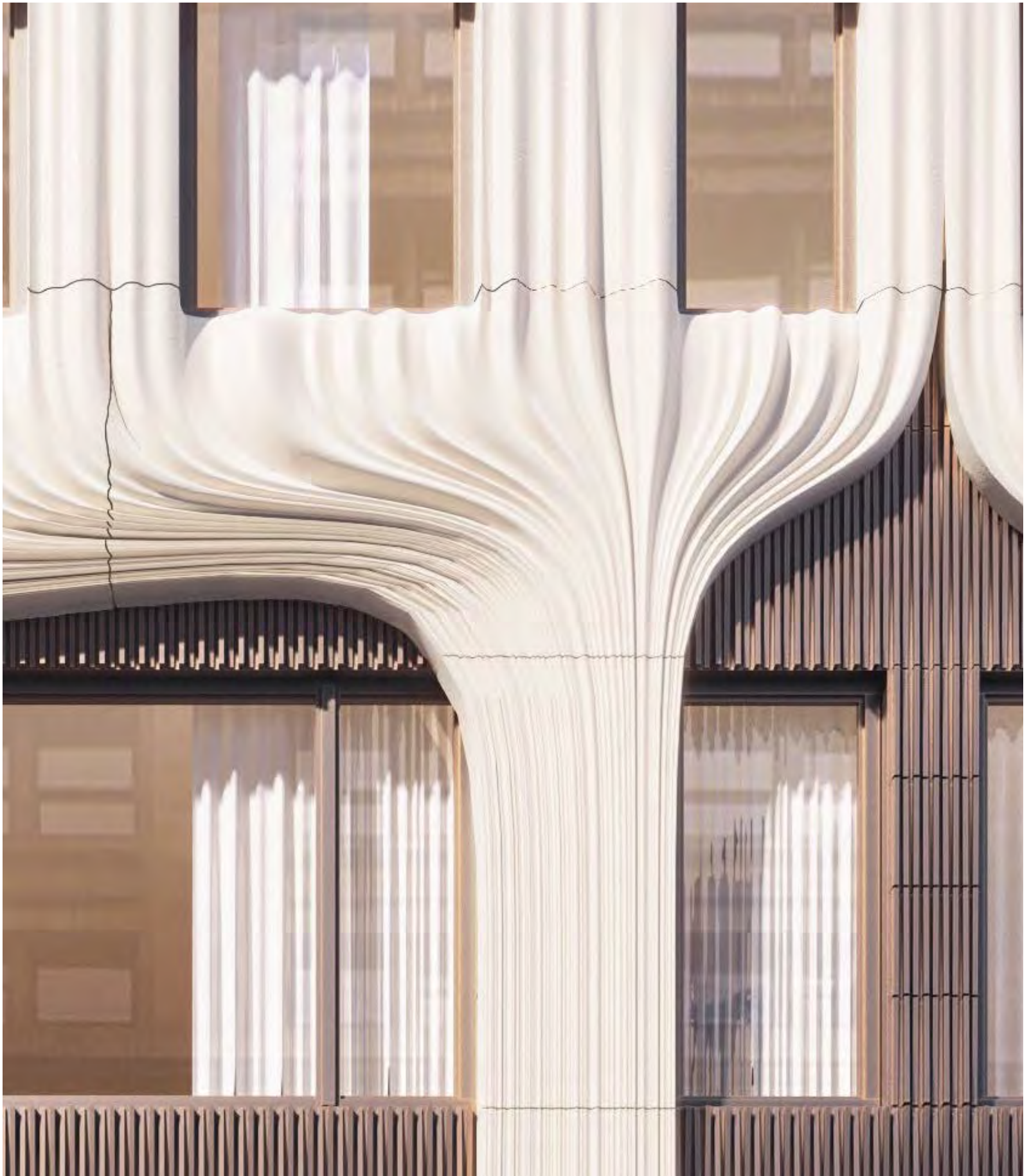
10 WEST 17 — FACADE - VISUALIZATION - STREET ELEVATION & CLOSE UP OF SEAMS BETWEEN PANELS
