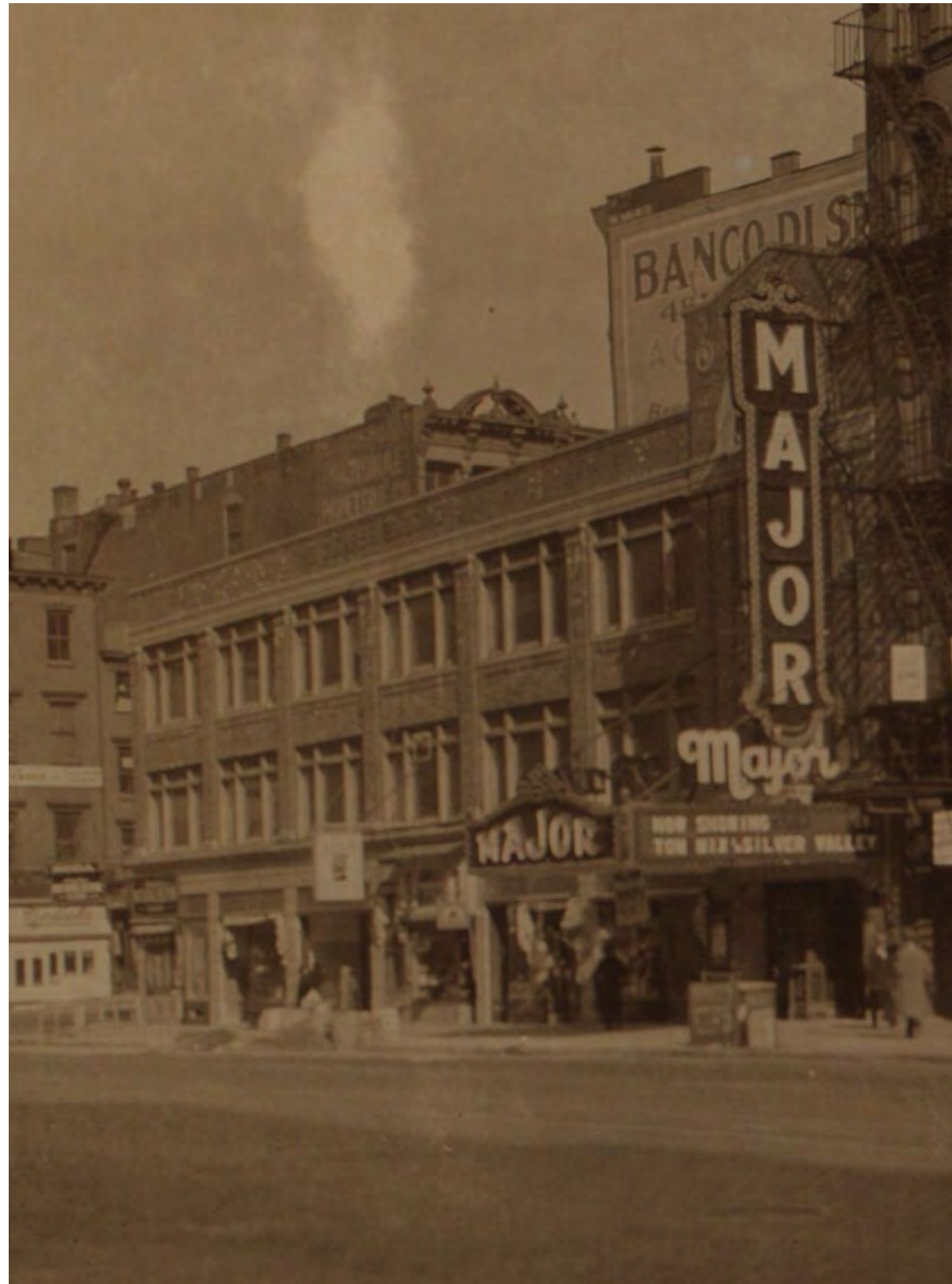
277 Canal Street, 1928 (NYPL)
