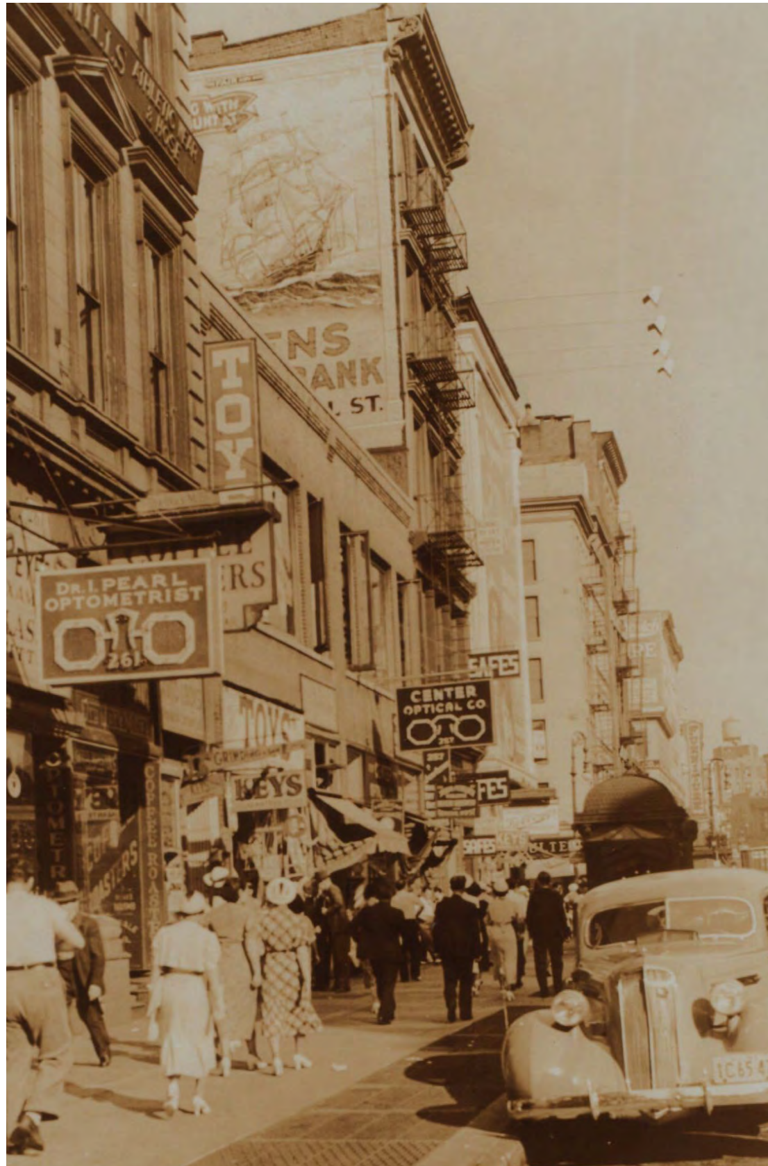
Canal Street near Broadway, 1937 (NYPL)
