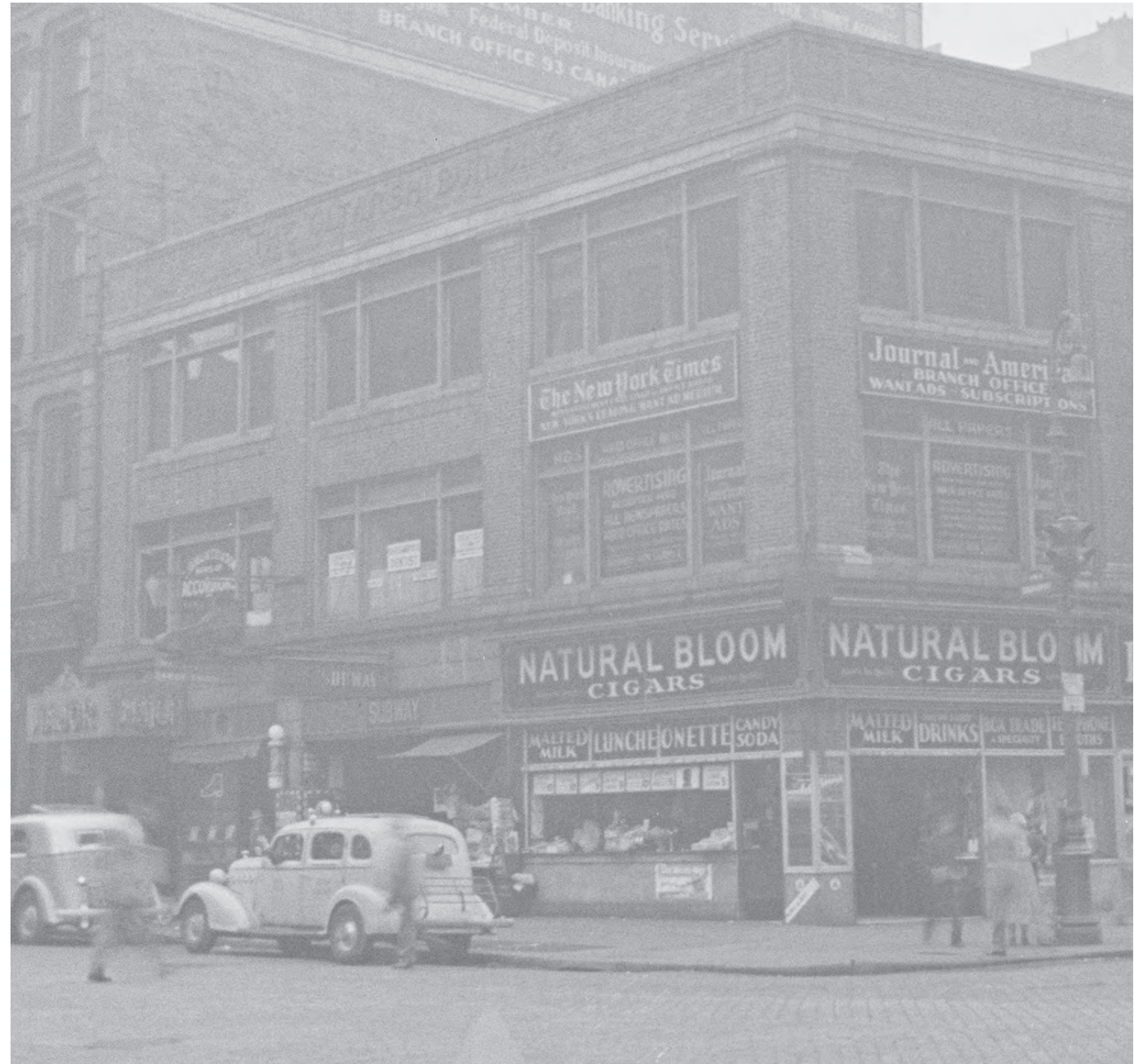
277 Canal Street, ca. 1940 Tax Photo (Municipal Archives)
