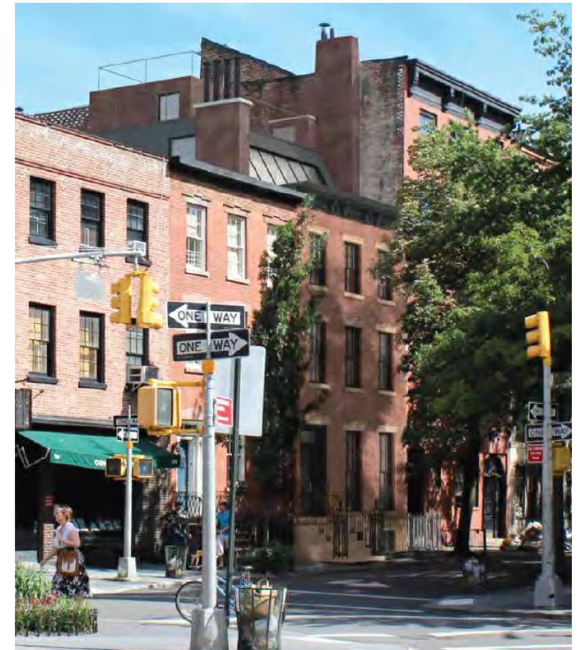
327 WEST 4TH STREET. STUDIO WINDOW ADDITION APPROVED IN 2017
