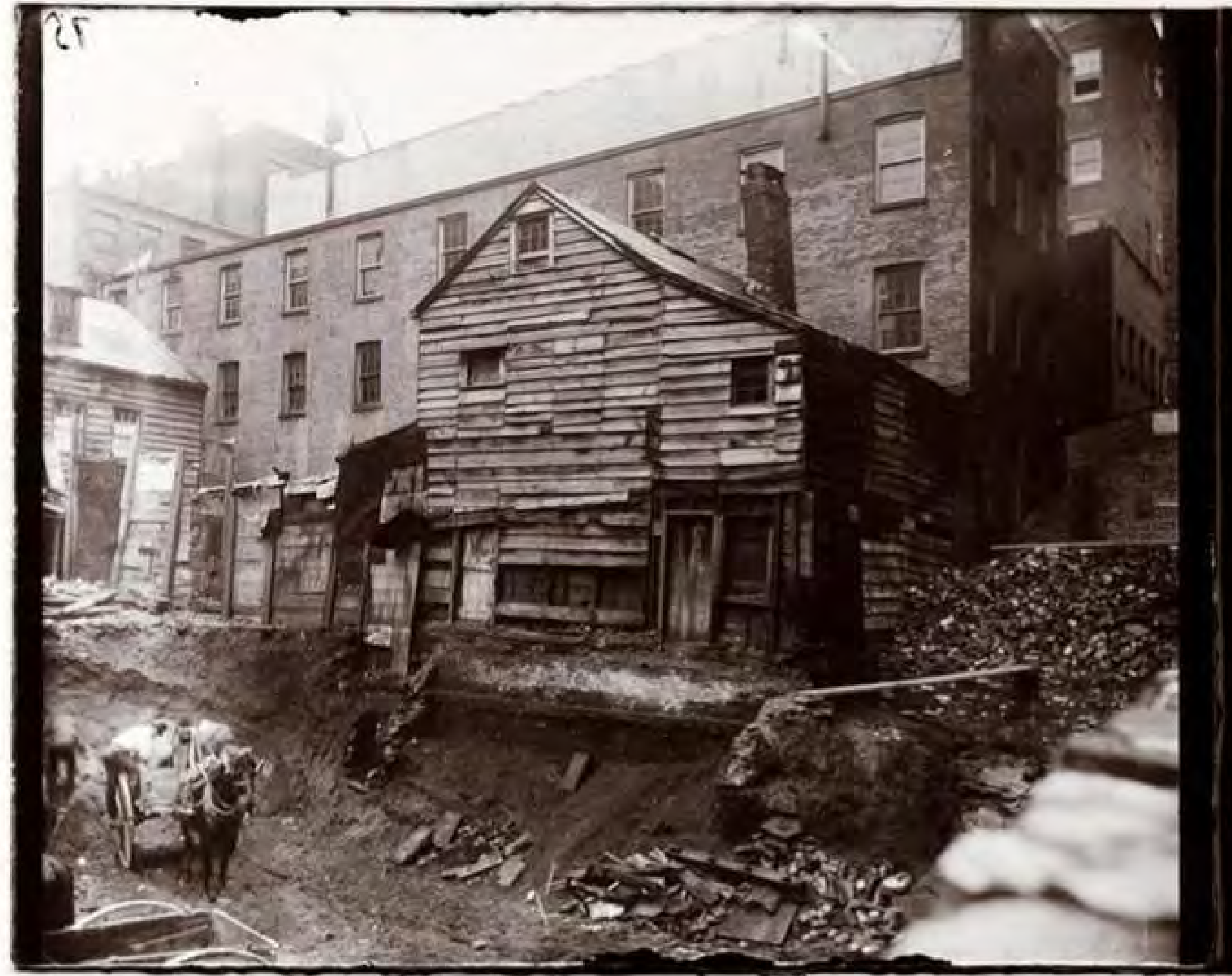
BACK HOUSE ON BLEECKER STREET, 1890 (MCNY)
