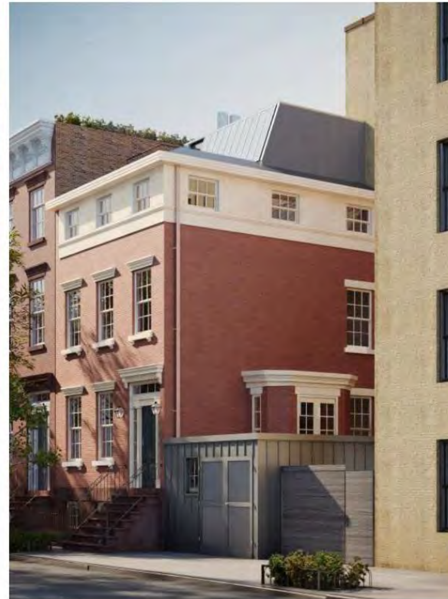
65 HORATIO STREET, SIDE AND ROOFTOP ADDITIONS APPROVED IN 2020
