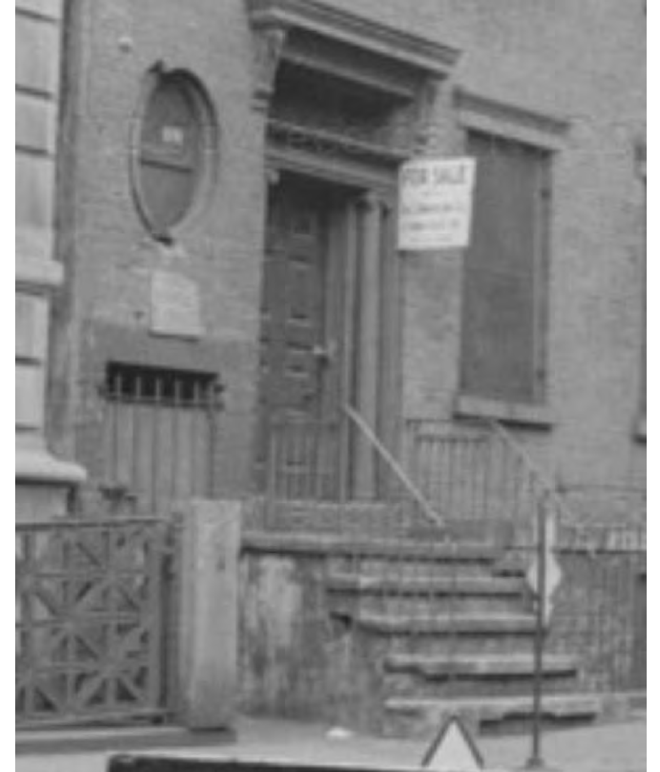
DETAIL OF 1940's 131 CHARLES STREET
