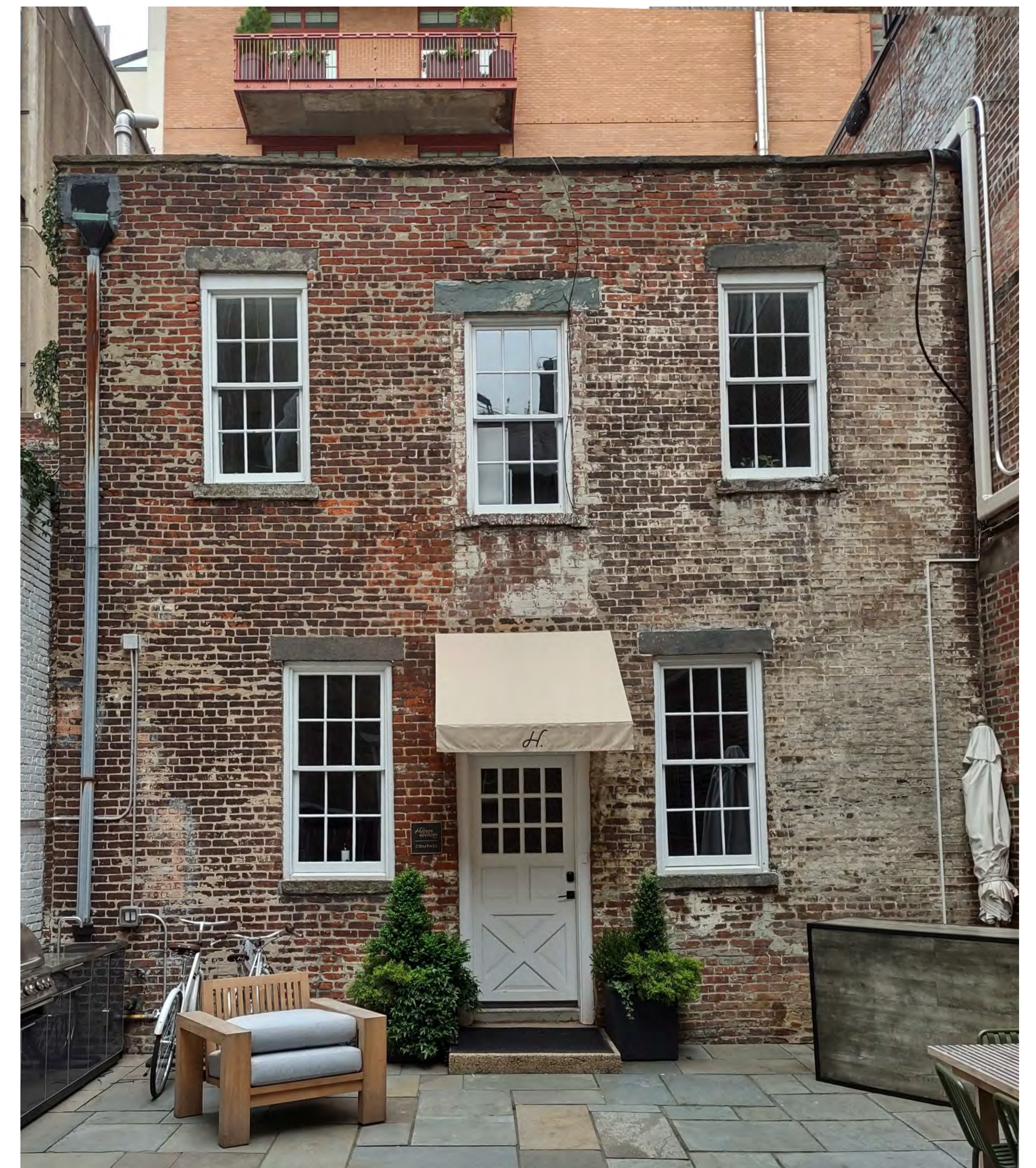
REAR BUILDING - FRONT FACADE
