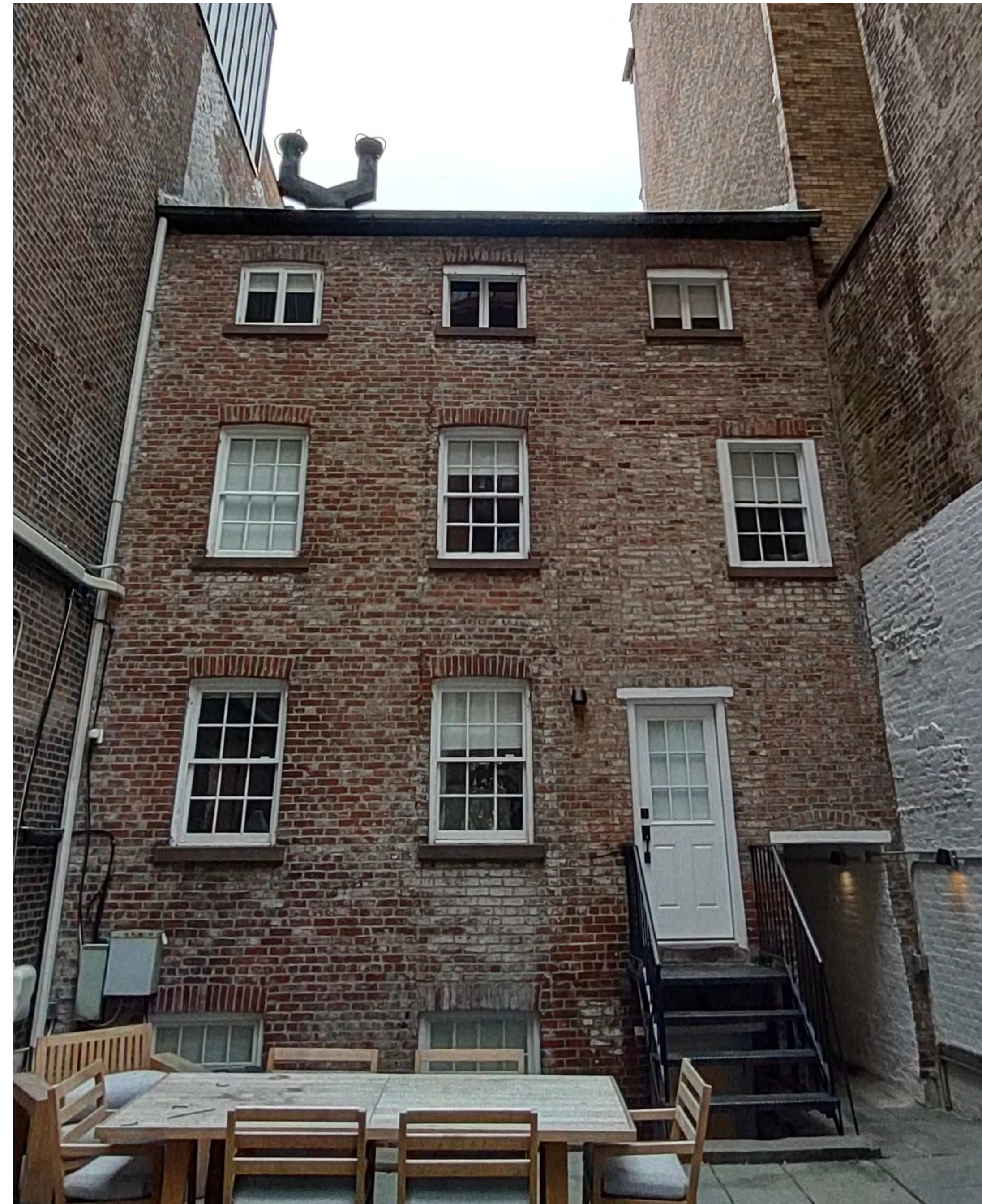
FRONT BUILDING - REAR FACADE
