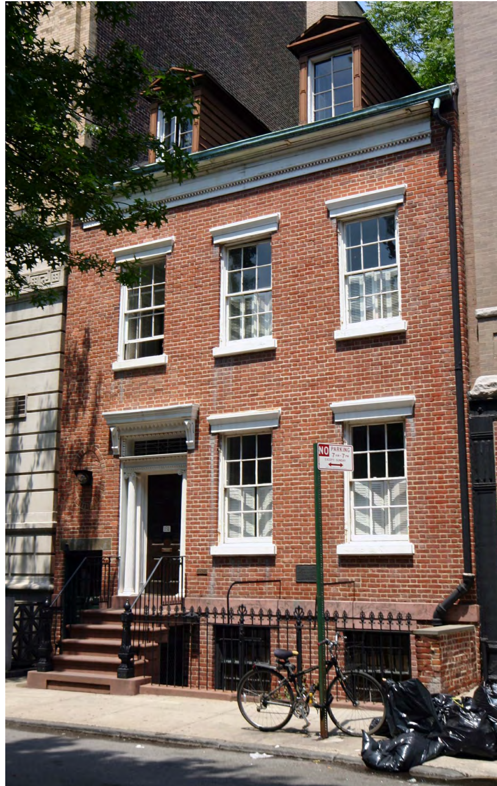
FRONT BUILDING - FRONT FACADE
