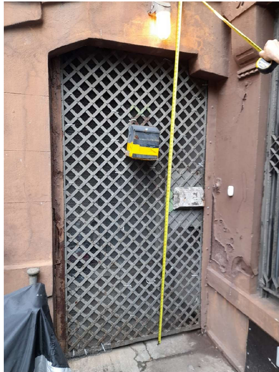
OVERALL HEIGHT OF BASEMENT ENTRANCE UNDER STOOP
