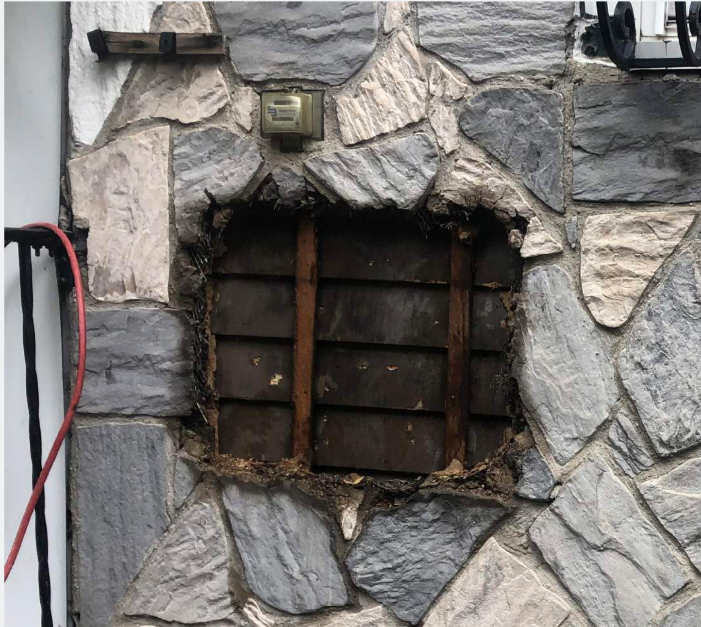
Facade probe above porch - clapboard siding
