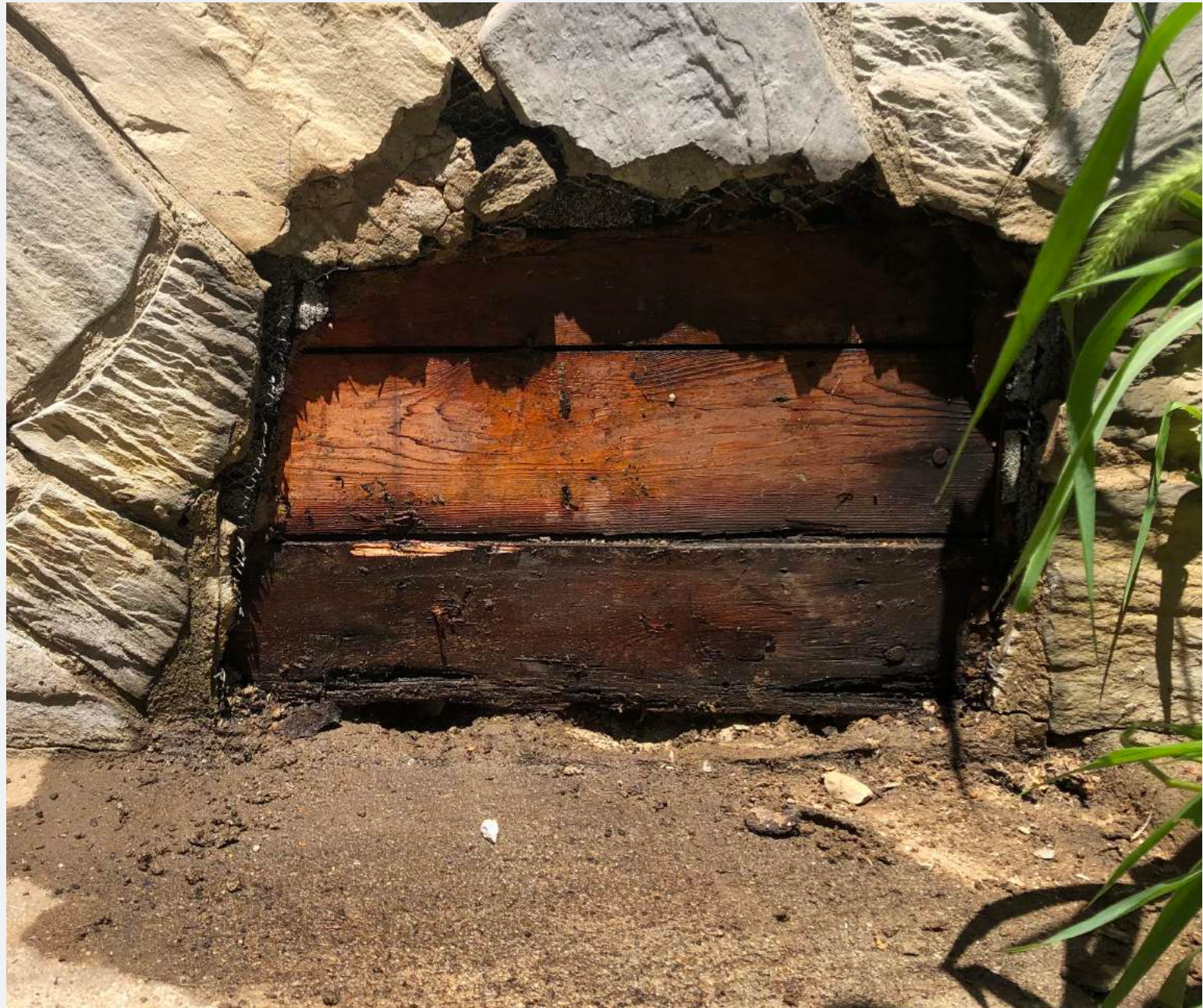
Facade probe below porch - shiplap siding
