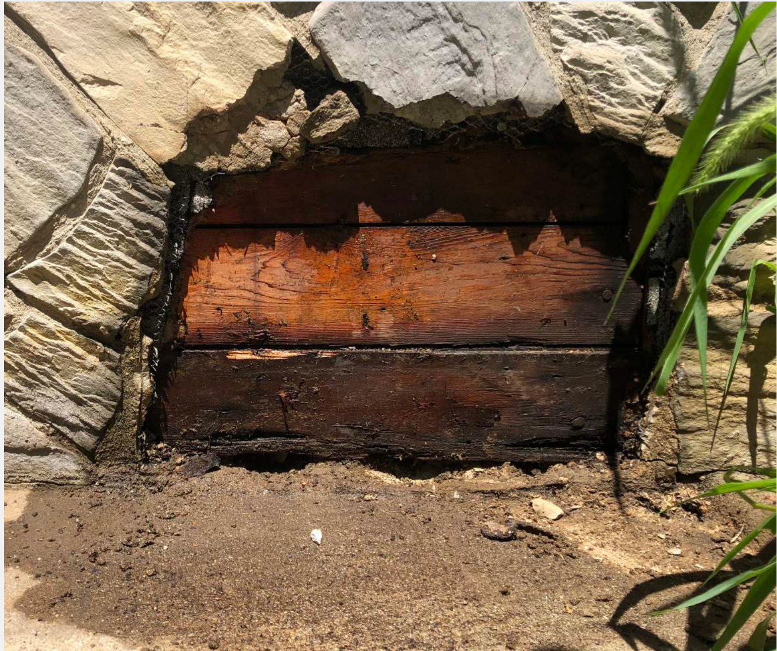
Facade probe below porch - shiplap siding
