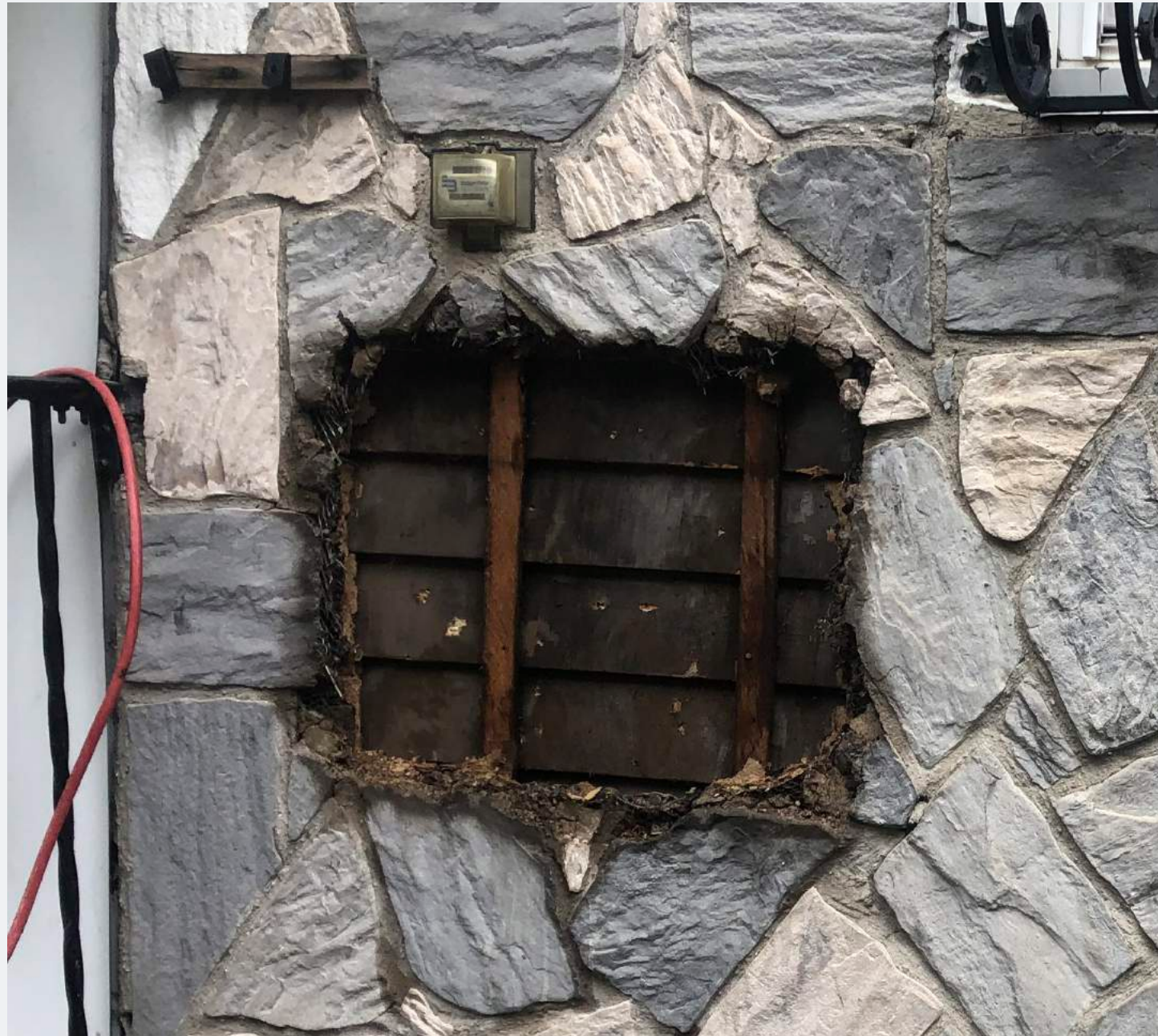
Facade probe above porch - clapboard siding
