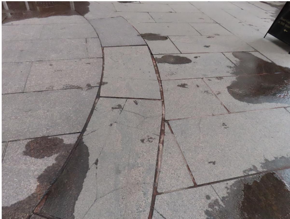
CRACKED FLAGS AT THE EXISTING COURTYARD
