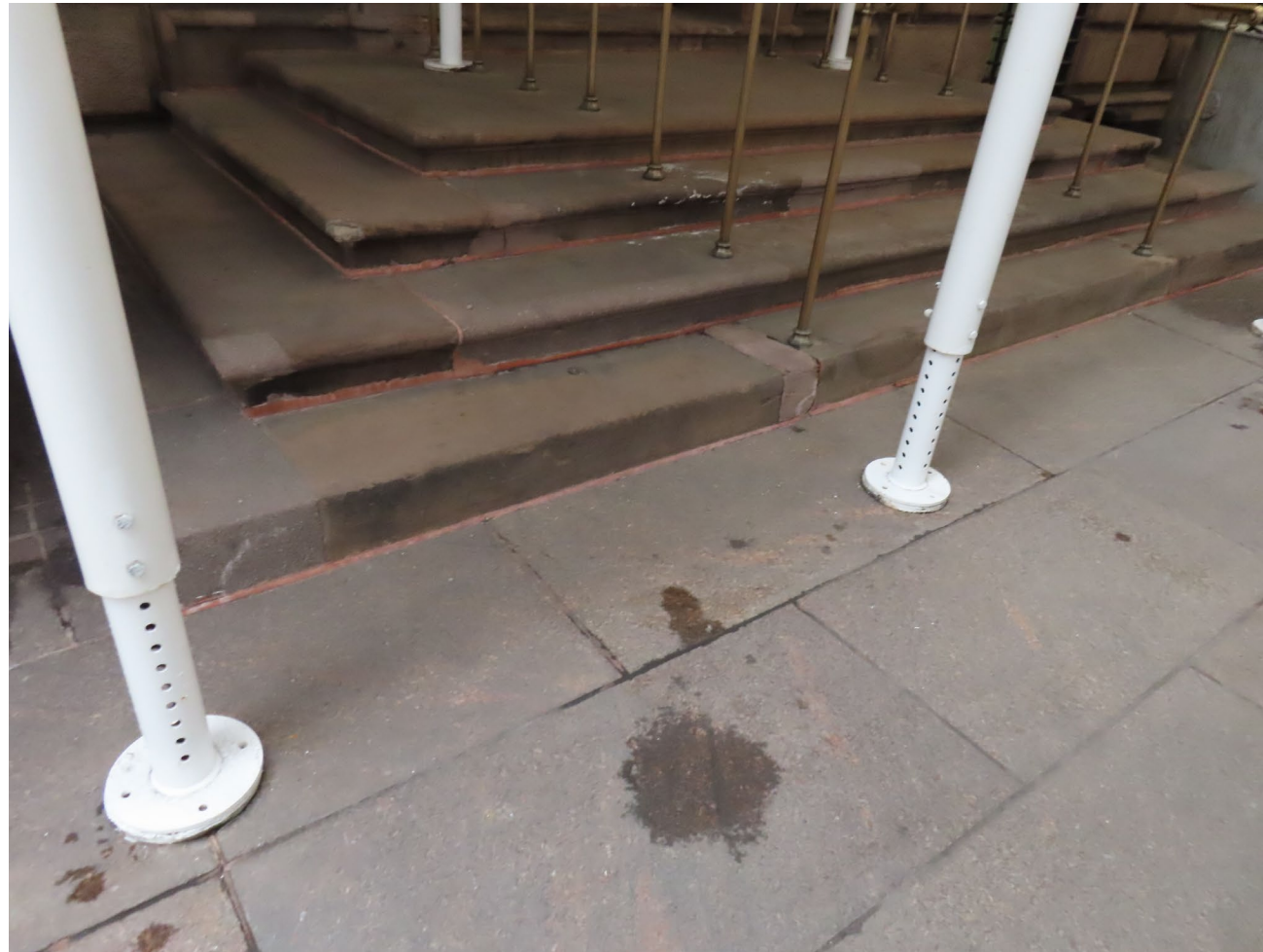
SPALLED BROWNSTONE AND FAILING PATCHES AT THE NORTH COURTYARD ENTRANCE
