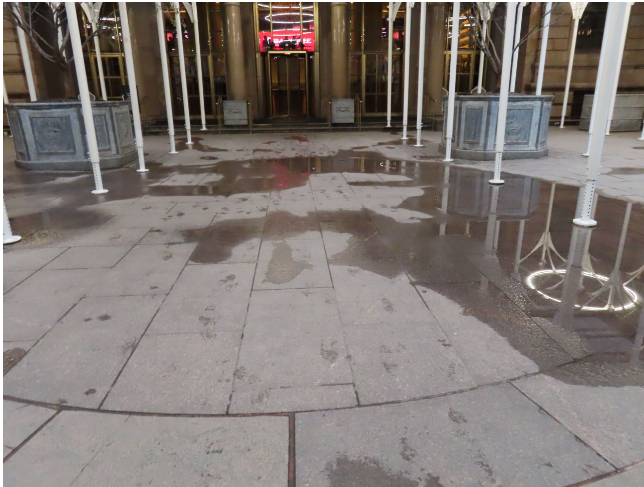
POOLING WATER IN THE COURTYARD FOLLOWING A RAINSTORM
