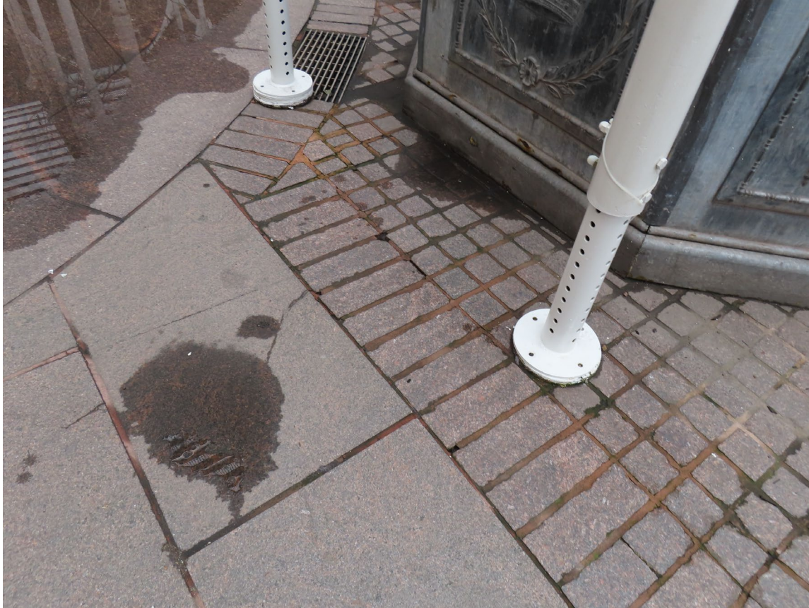
CRACKED GRANITE FLAG AT THE EXISTING COURTYARD
