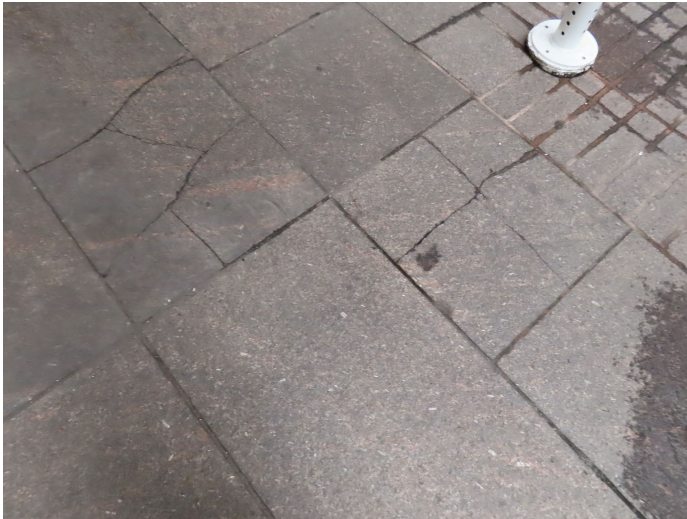
CRACKED GRANITE FLAG AT THE EXISTING COURTYARD
