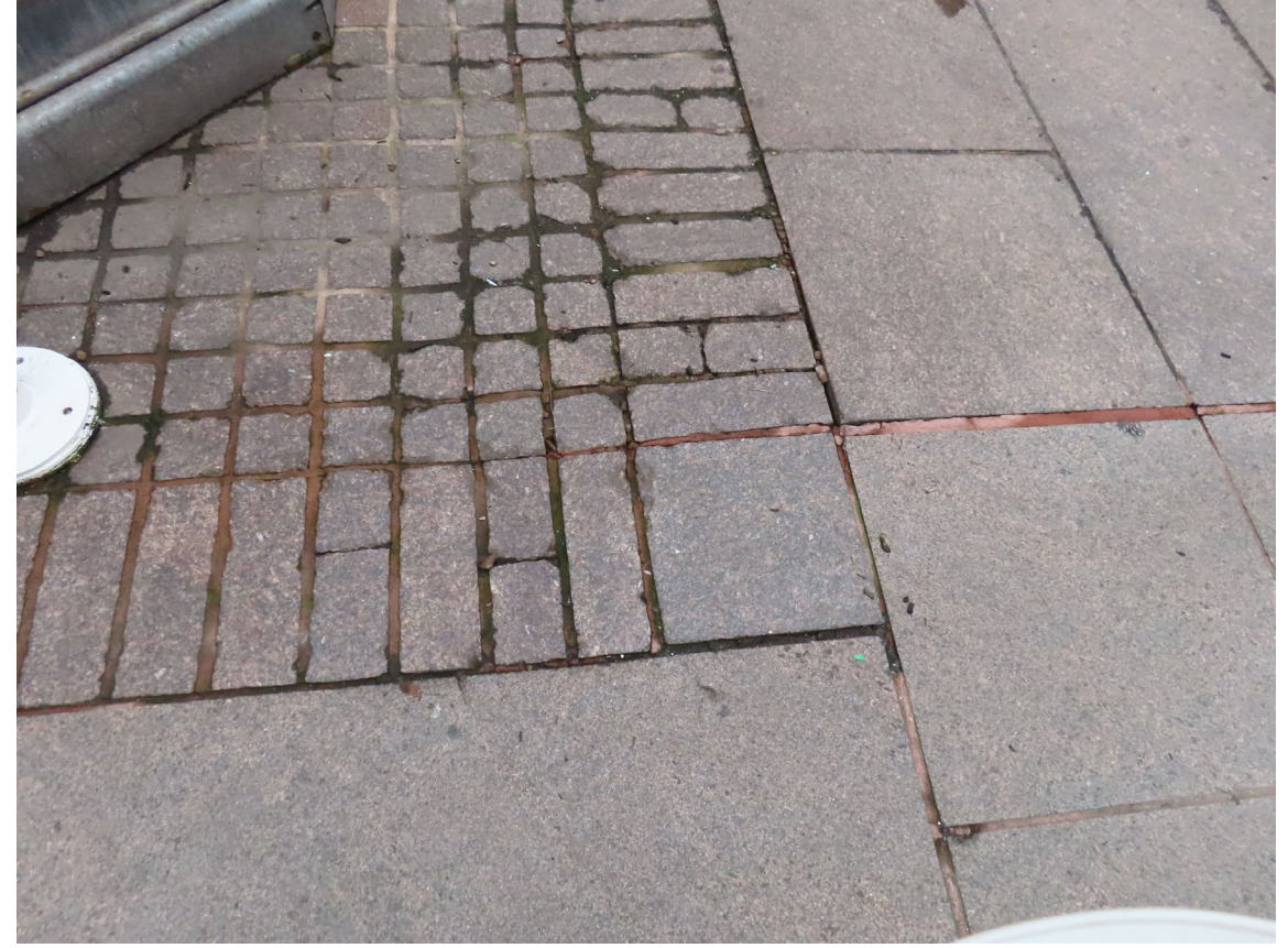
CRACKED GRANITE FLAG AT THE EXISTING COURTYARD
