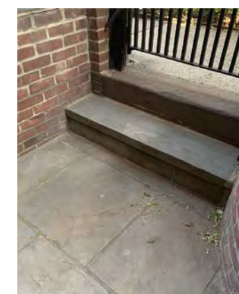
C VIEW OF SERVICE ENTRANCE STAIRS
