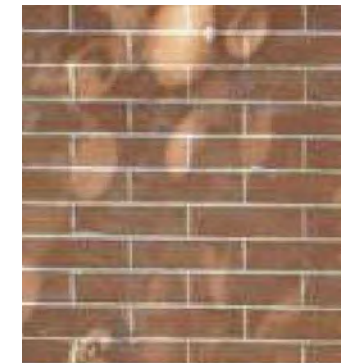
BRICK RETAINING WALLS: RED BRICK TO MATCH TOWNHOUSE FACADE
