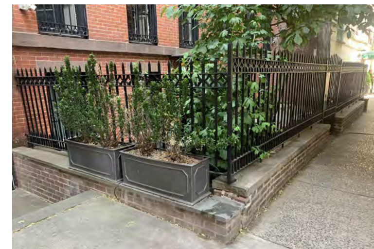
A VIEW OF RETAINING WALL AND PERIMETER FENCE LOOKING NORTHEAST
