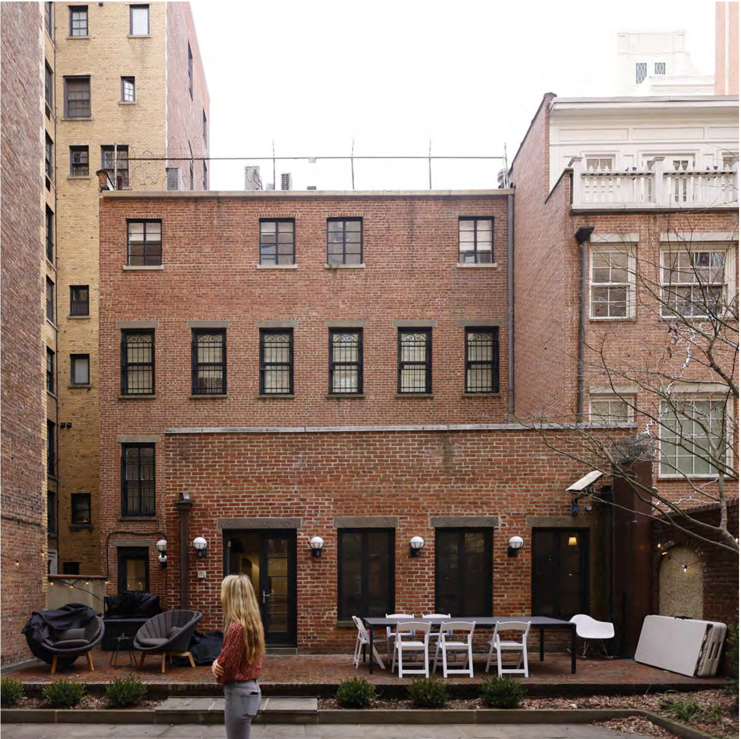
REAR ELEVATION VIEW - EXISTING
