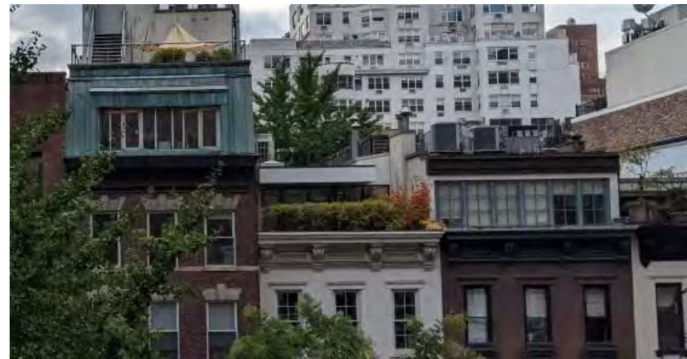
158, 160, 162A East 78 th Street (Non-Landmarked buildings across the street)
