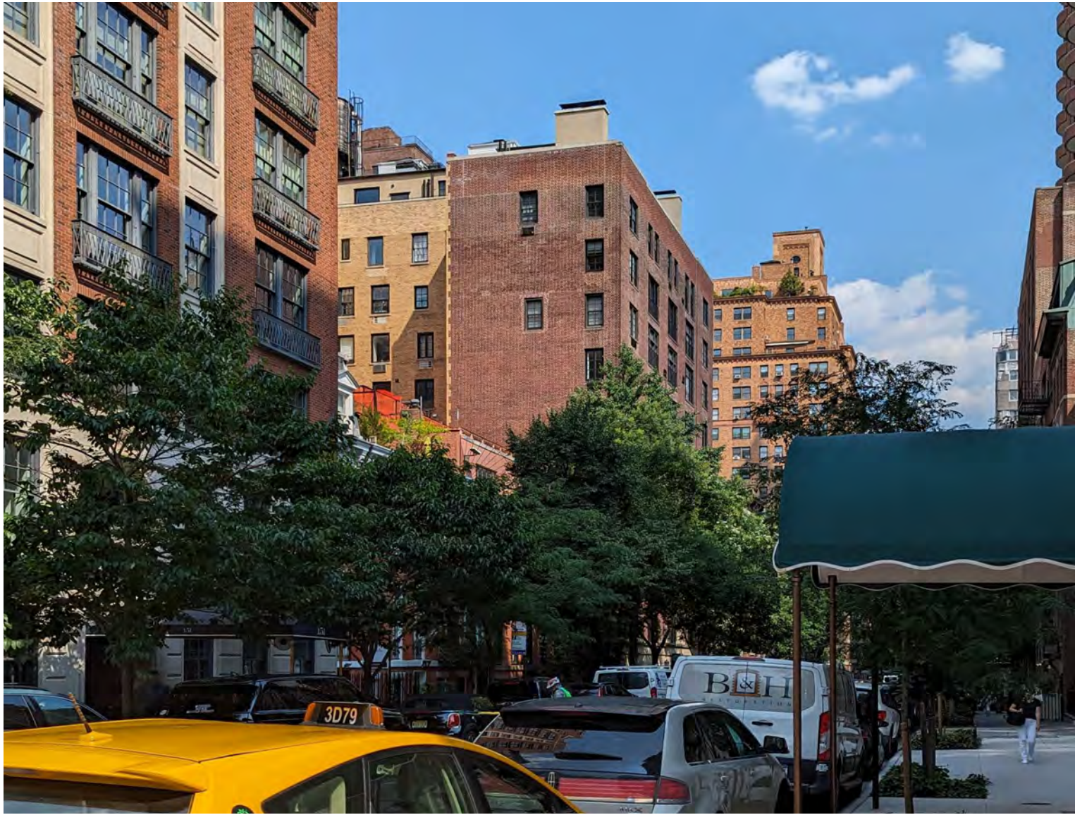
EXISTING CONDITIONS WITH MOCKUP
