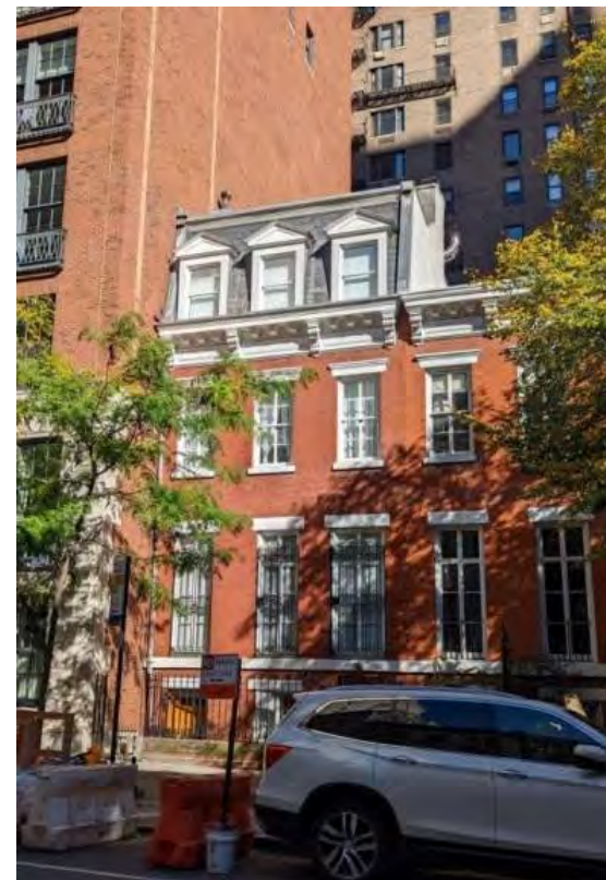
157 East 78 th Street Individual Landmark (Mansard addition in 1877; Rear addition- 1914)
