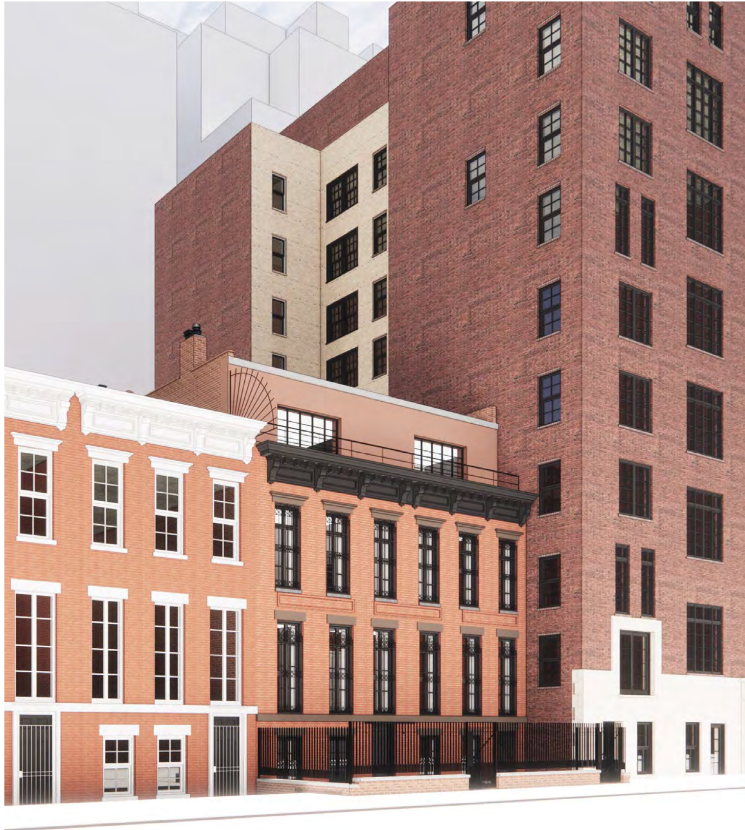
FRONT PERSPECTIVE VIEW - EXISTING CONDITIONS
