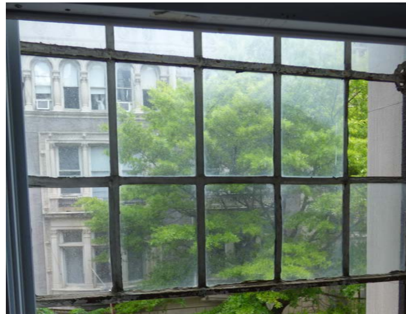
Second floor window detail (from the interior)
