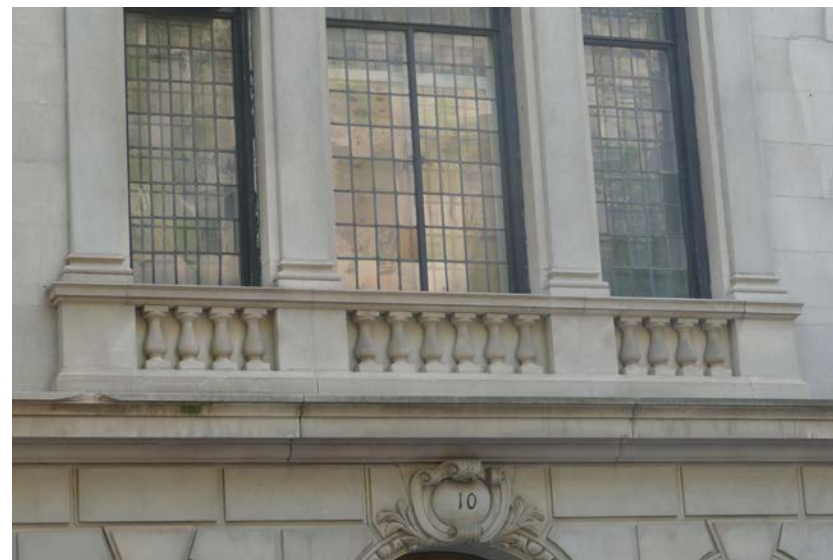
Existing stone balusters at the second floor.
