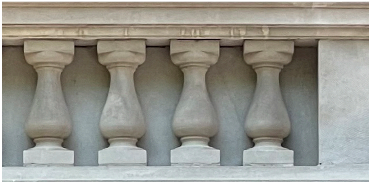
Cast Stone Balustrade
