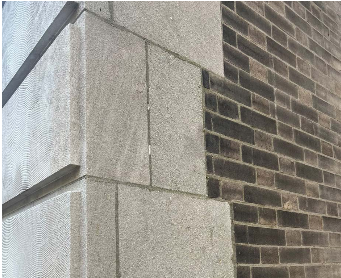
Street Facade Masonry
