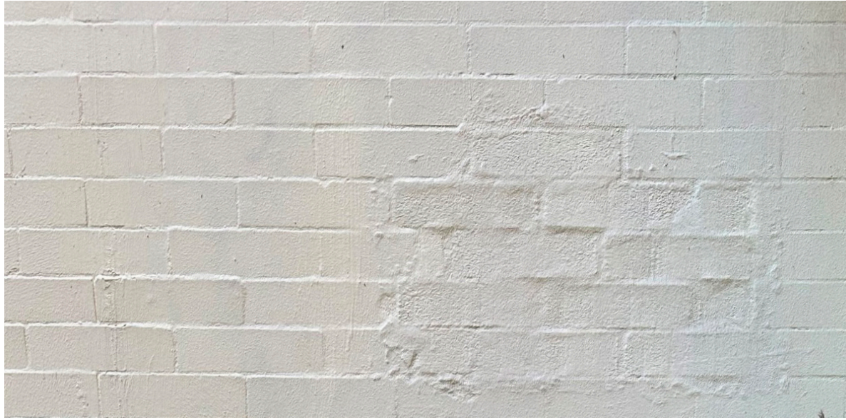
Rear Facade Masonry
