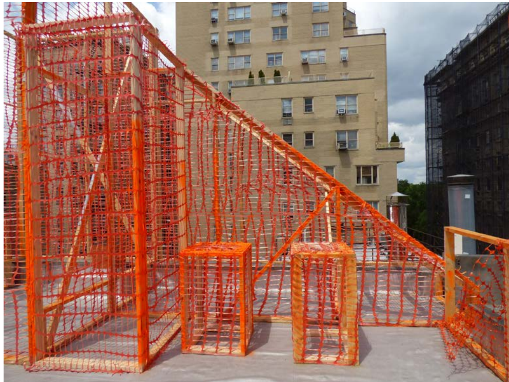
4 | Stair bulkhead, looking west
