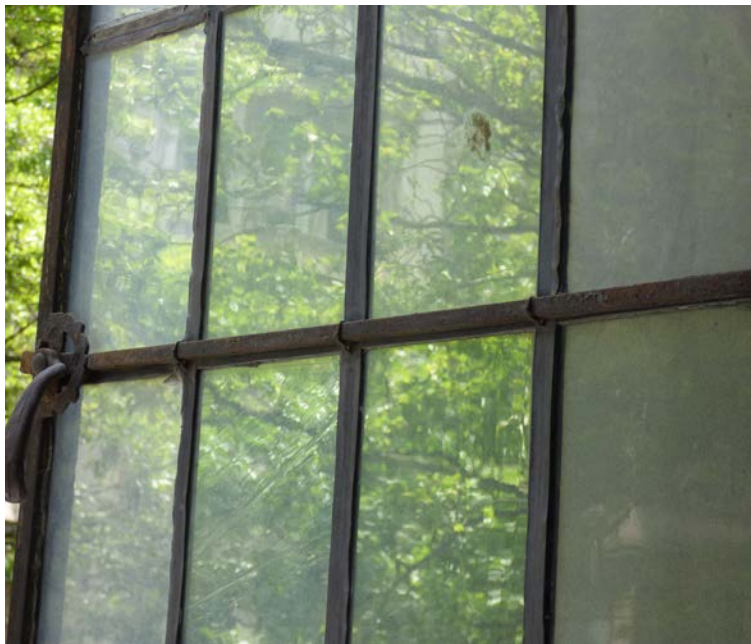
Parlor floor window detail
