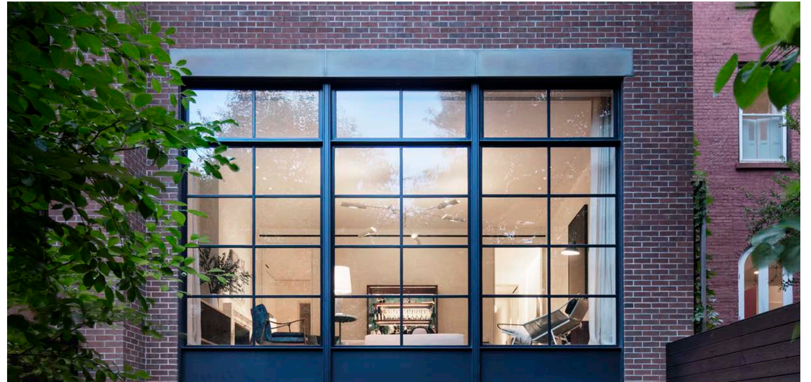
Steel Windows on Rear Penthouse
