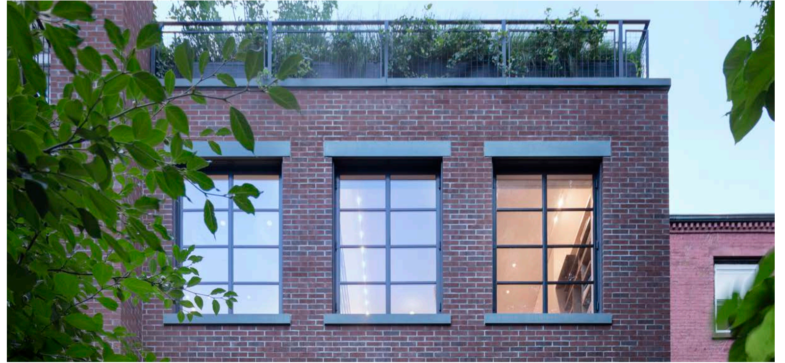
Steel Windows on Rear Facade
