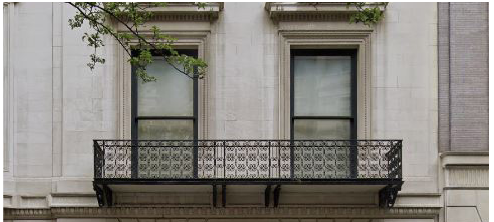
Upper Windows on Front Facade
