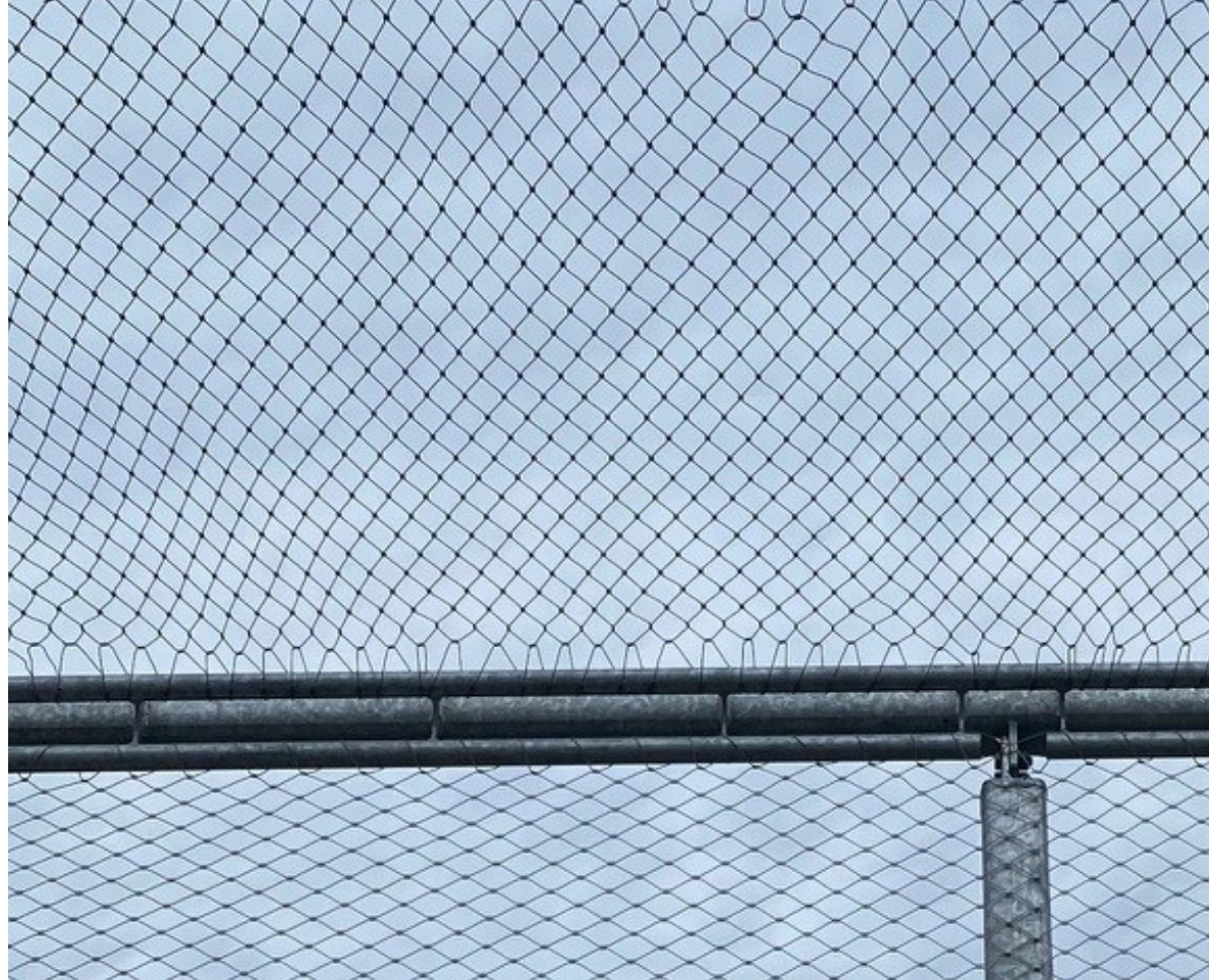
Mesh on Painted Steel Tubes
