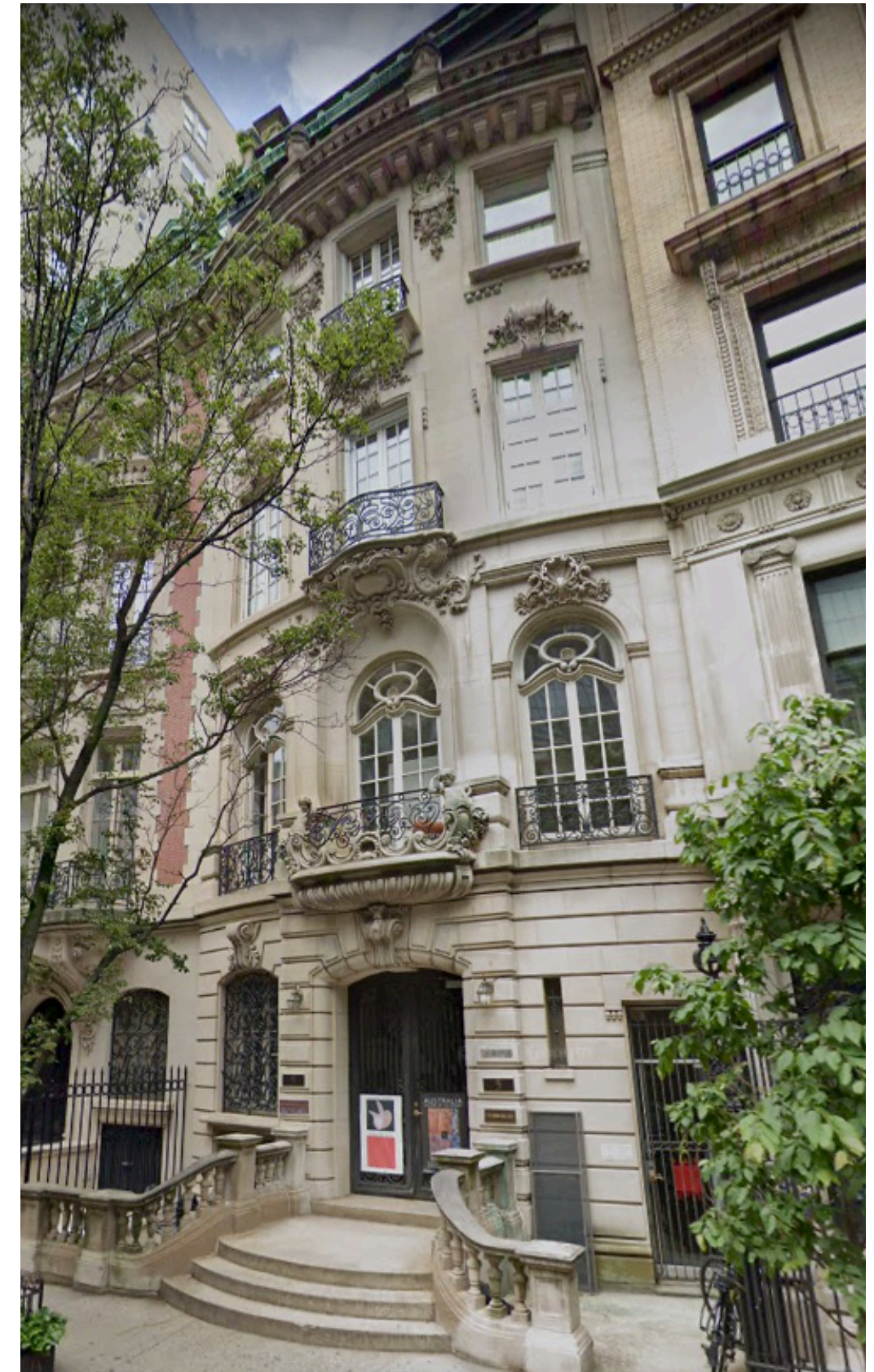
5 East 82nd Street stone balusters (1901, Beaux Arts)
