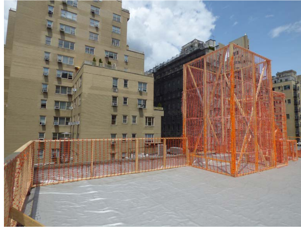
2 | Railing and elevator bulkhead, looking northwest
