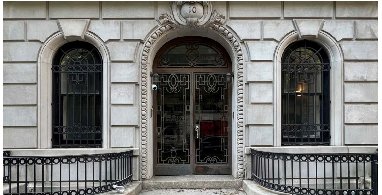
Lower Windows on Front Facade
