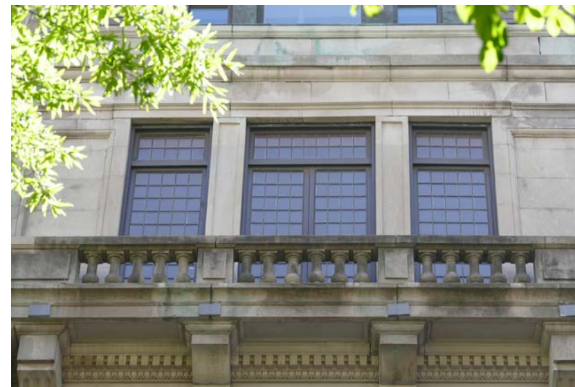
Existing stone balusters at the fourth floor.
