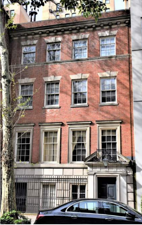
F: 128 - 130 EAST 73RD STREET COMBINED 1928
