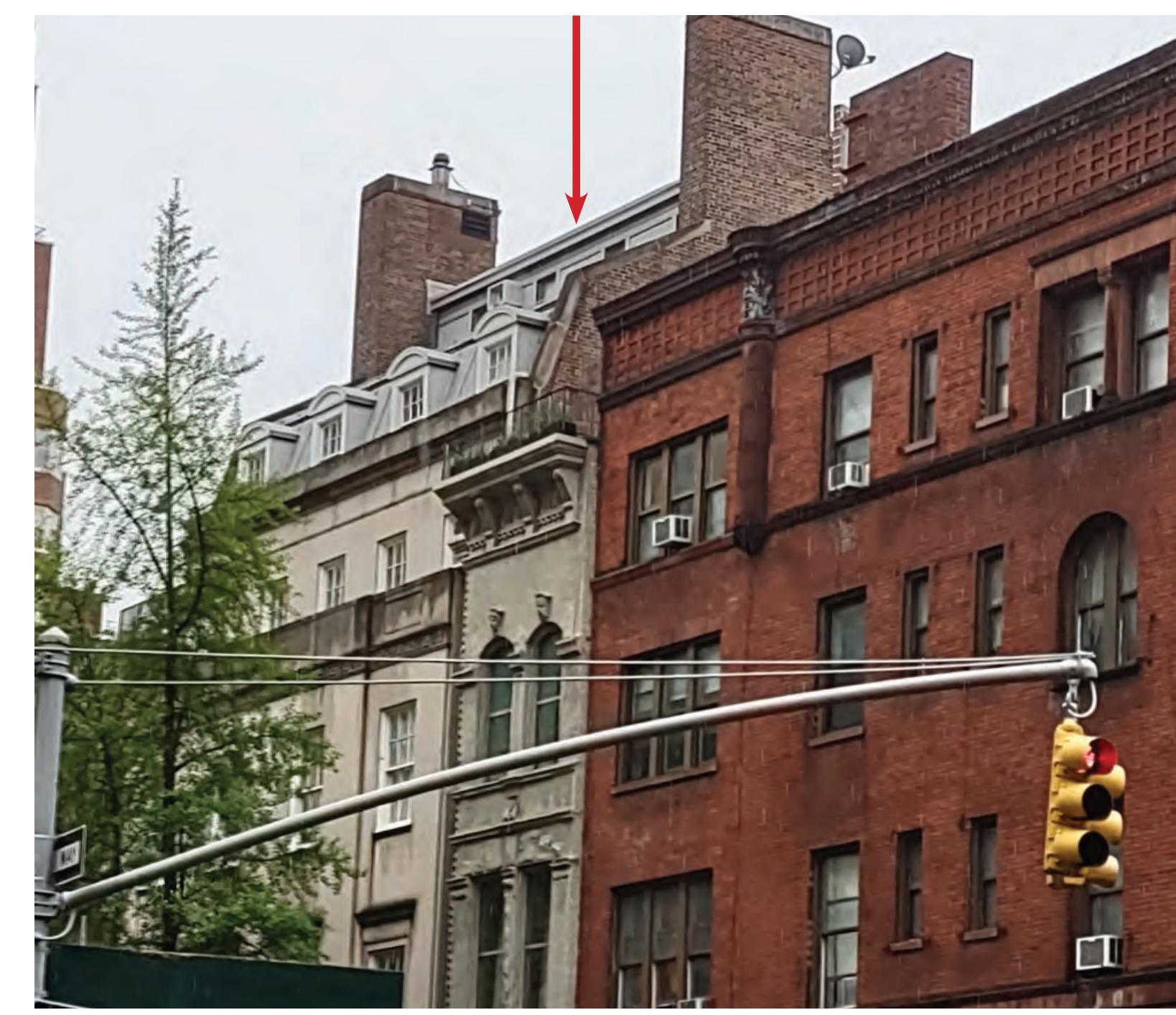
48 EAST 92ND ST. ZOOMED IN VIEW FROM MADISON AVENUE. ROOFTOP ADDITION IS VISIBLE. (MAY 2023)
