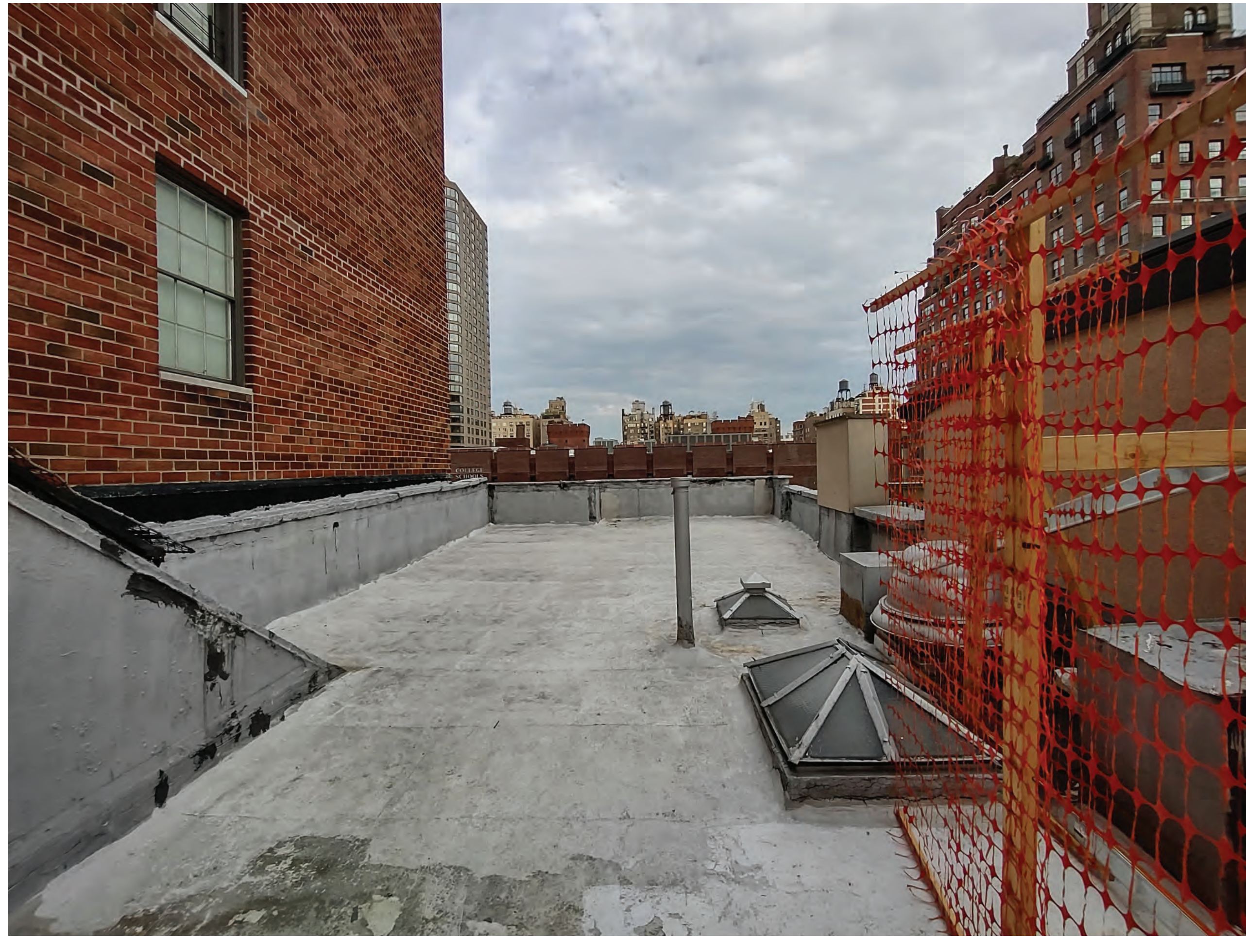
ROOFTOP, LOOKING WEST.
