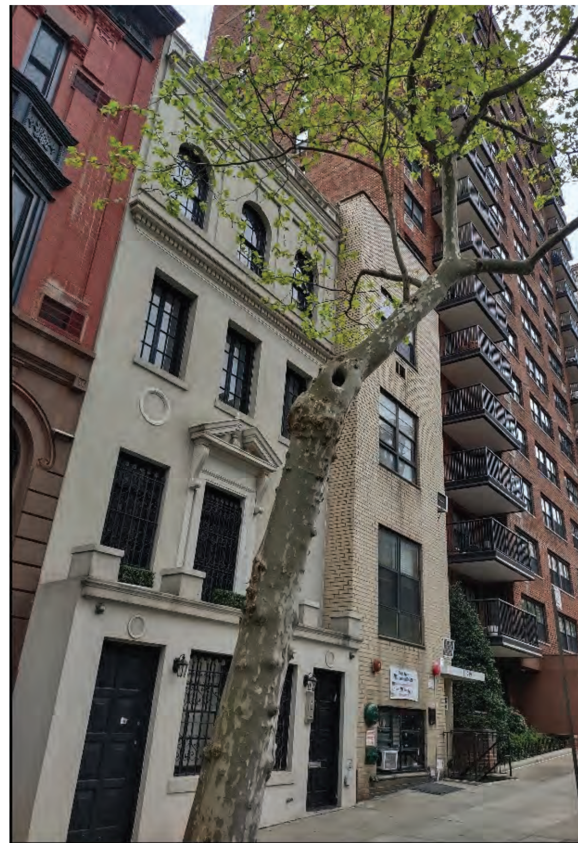
PHOTO 1: 1211 PARK AVENUE CARNEGIE HILL HISTORIC DISTRICT 1-STORY ROOFTOP ADDITION, IN SAME PLANE AS REAR FACADE, APPROVED IN 2009 CofA 10-4613
