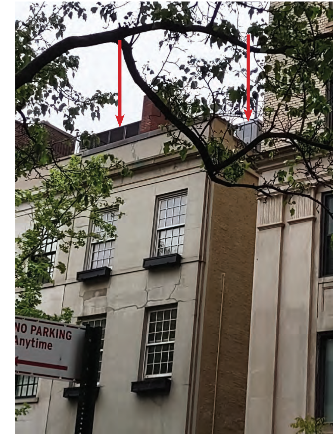
63 AND 65 EAST 92ND ST. ZOOMED IN. VIEWED WALKING EAST. ROOFTOP ADDITIONS ARE VISIBLE (MAY 2023)
