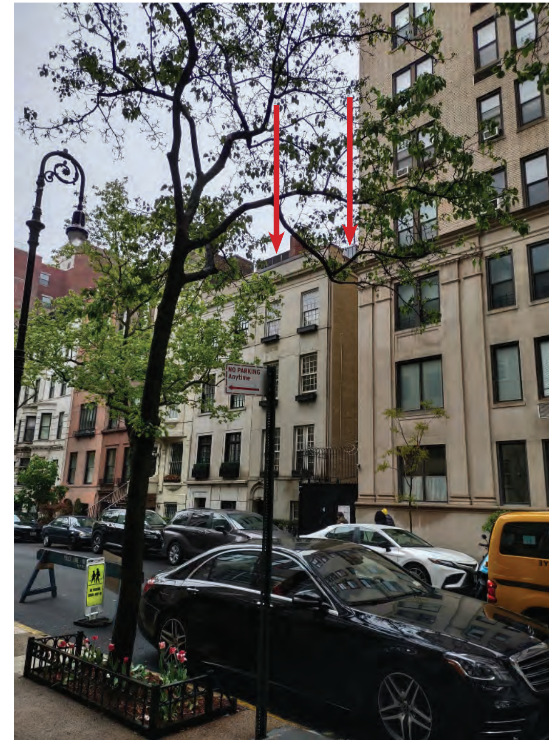
63 AND 65 EAST 92ND ST. VIEWED WALKING EAST. ROOFTOP ADDITIONS ARE VISIBLE (MAY 2023)
