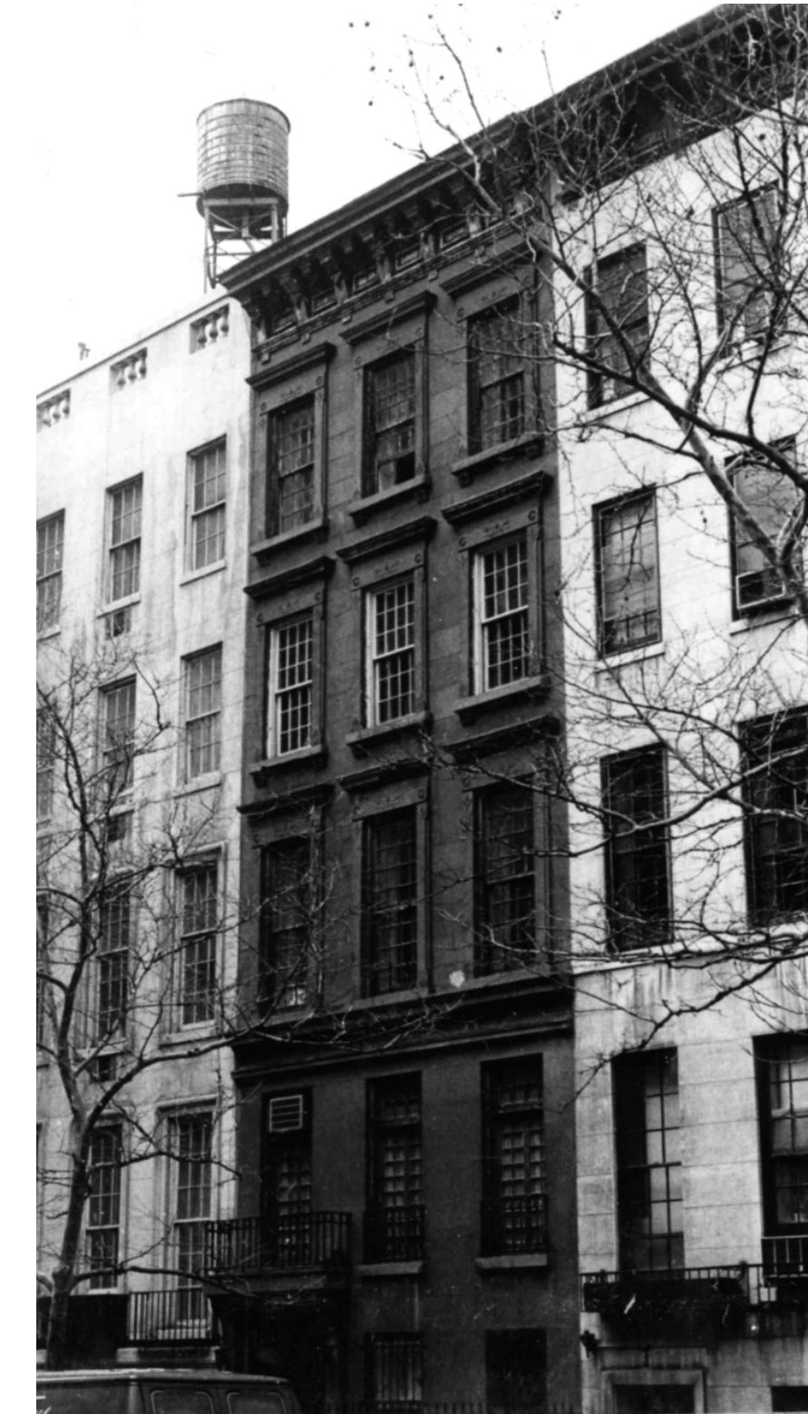
33 EAST 63RD ST. - DESIGNATION PHOTO UPPER EAST SIDE HISTORIC DISTRICT NEO-GREC STYLE
