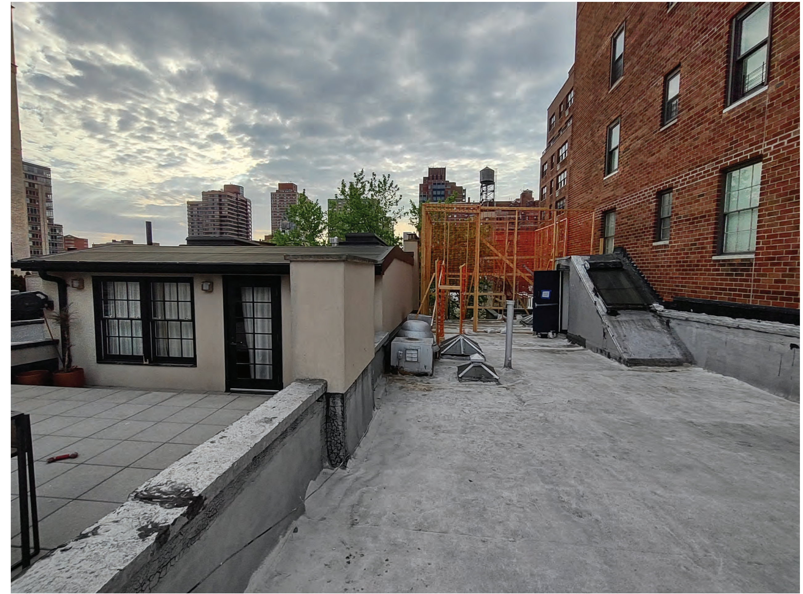
ROOFTOP, LOOKING EAST.
