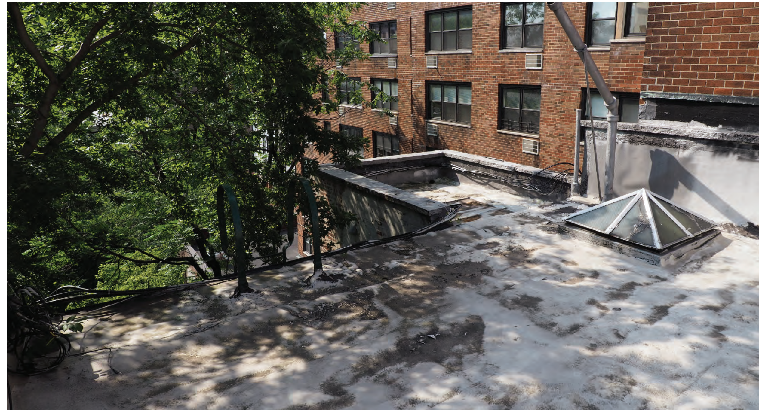
PHOTO 2: LOOKING EAST (REAR EXTENSION)
