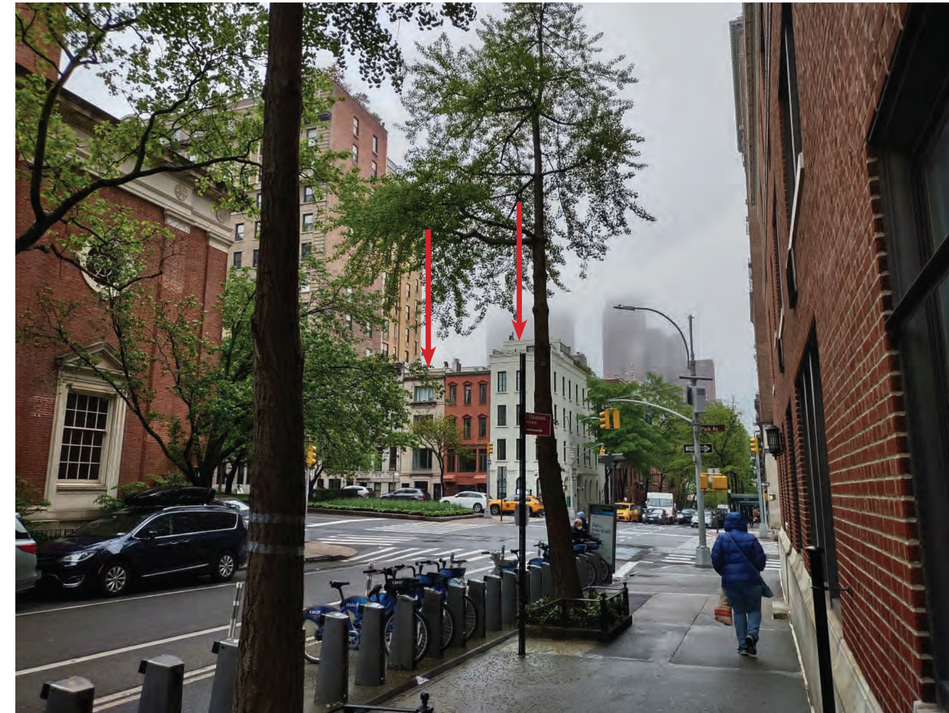
1141 - 1149 PARK AVENUE, VIEWED FROM THE WEST ON EAST 91ST ST. ROOFTOP ADDITIONS AT 1141 AND 1145 ARE VISIBLE (MAY 2023)
