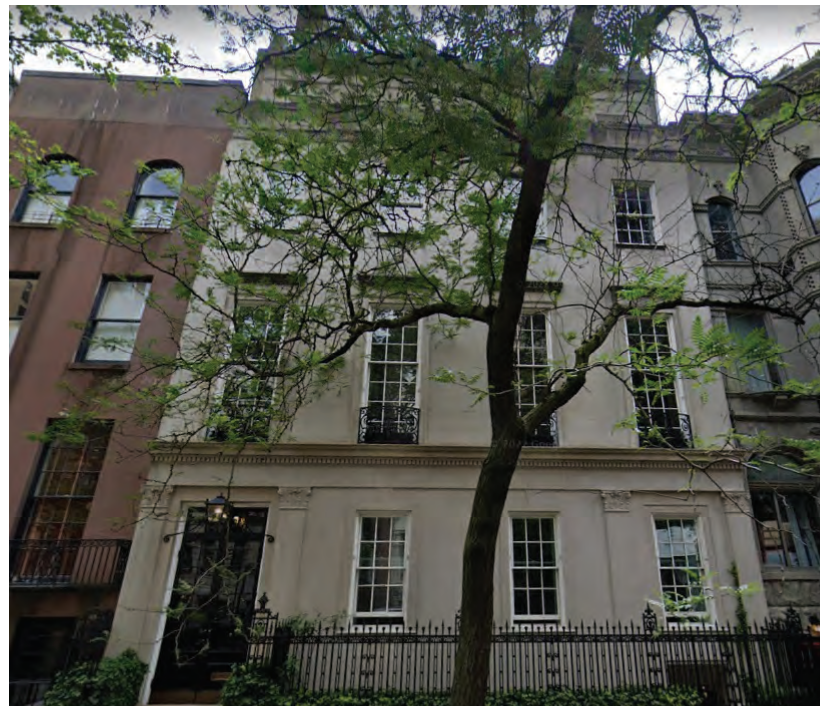
48 EAST 92ND ST. VIEWED FROM ACROSS THE STREET. ROOFTOP ADDITION IS NOT VISIBLE. (MAY 2023)
