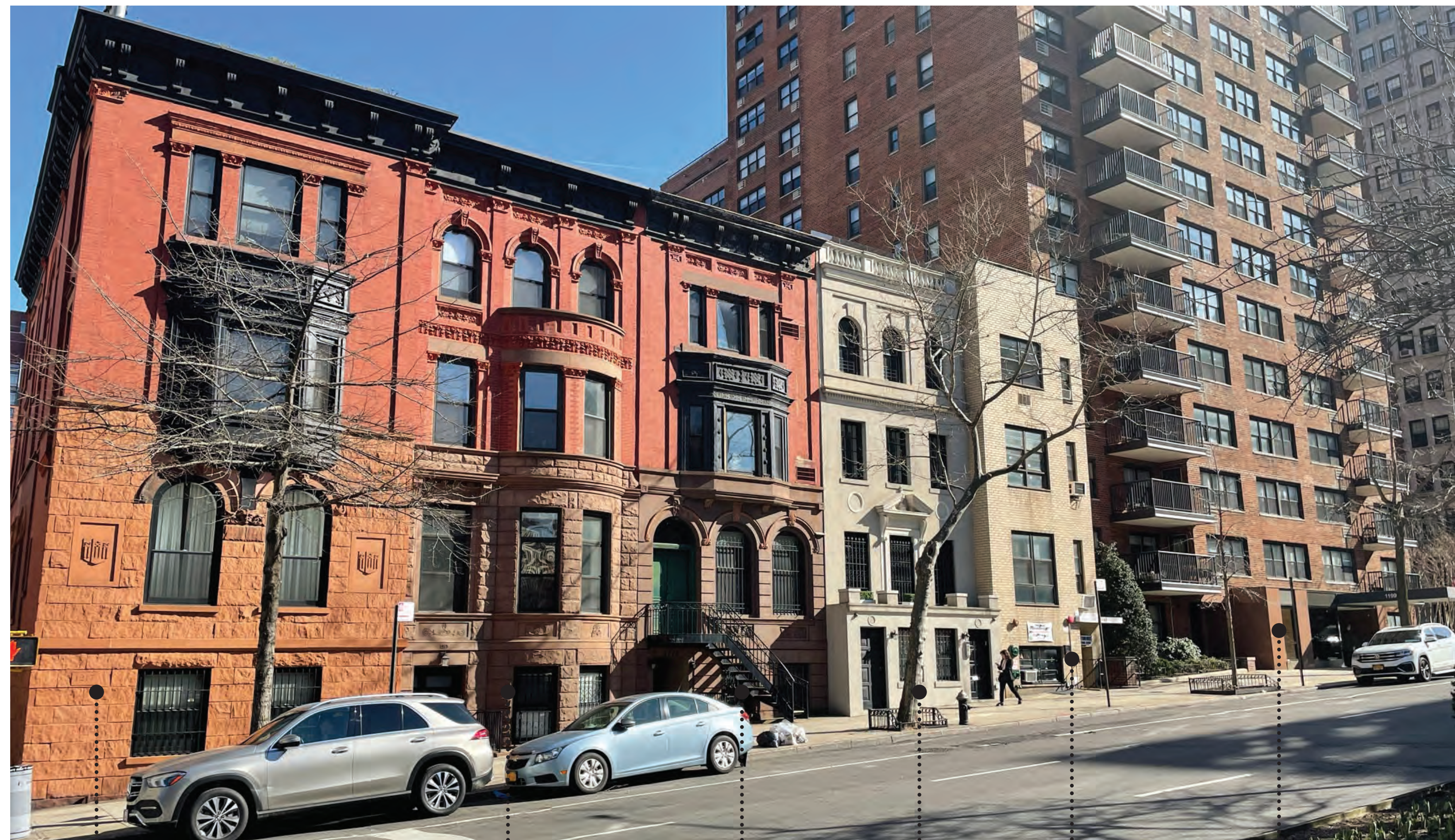
1217 PARK AVE. 1215 PARK AVE. 1213 PARK AVE. 1211 PARK AVE. 1209 PARK AVE. 1199 PARK AVE. VIEW - 1 FROM ACROSS THE 95TH STREET AND PARK AVENUE NOTE: THIS BUILDING IS NOT IN THE CARNEGIE HILL HISTORIC DISTRICT
