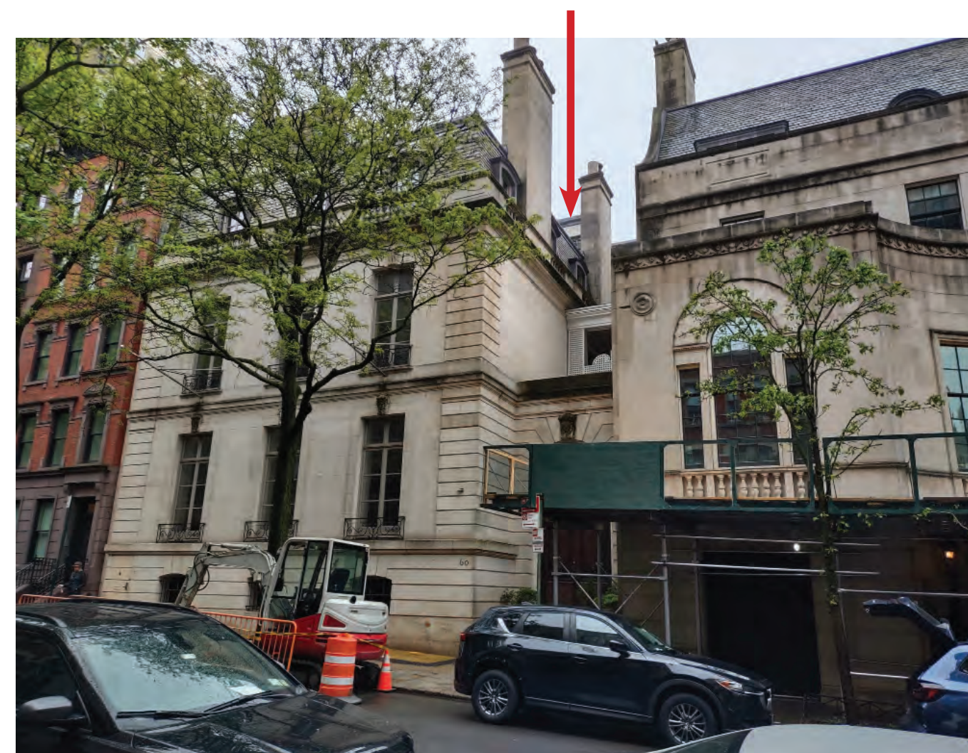
60 EAST 93RD ST. VIEWED FROM ACROSS THE STREET. ROOFTOP ADDITIONS ARE VISIBLE (MAY 2023)
