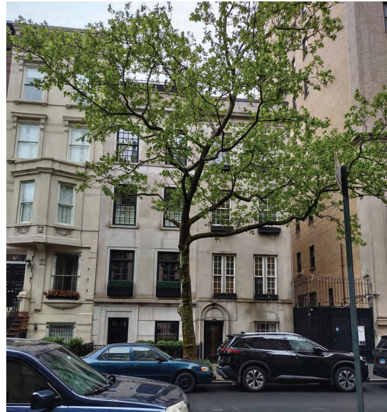
63 AND 65 EAST 92ND ST. VIEWED FROM ACROSS THE STREET. ROOFTOP ADDITIONS ARE NOT VISIBLE (MAY 2023)
