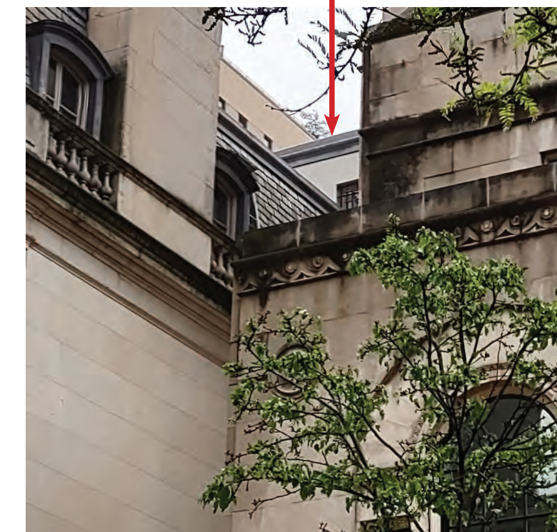
60 EAST 93RD ST. ZOOMED IN. VIEWED FROM ACROSS THE STREET AND WALKING WEST. ROOFTOP ADDITIONS ARE VISIBLE (MAY 2023)
