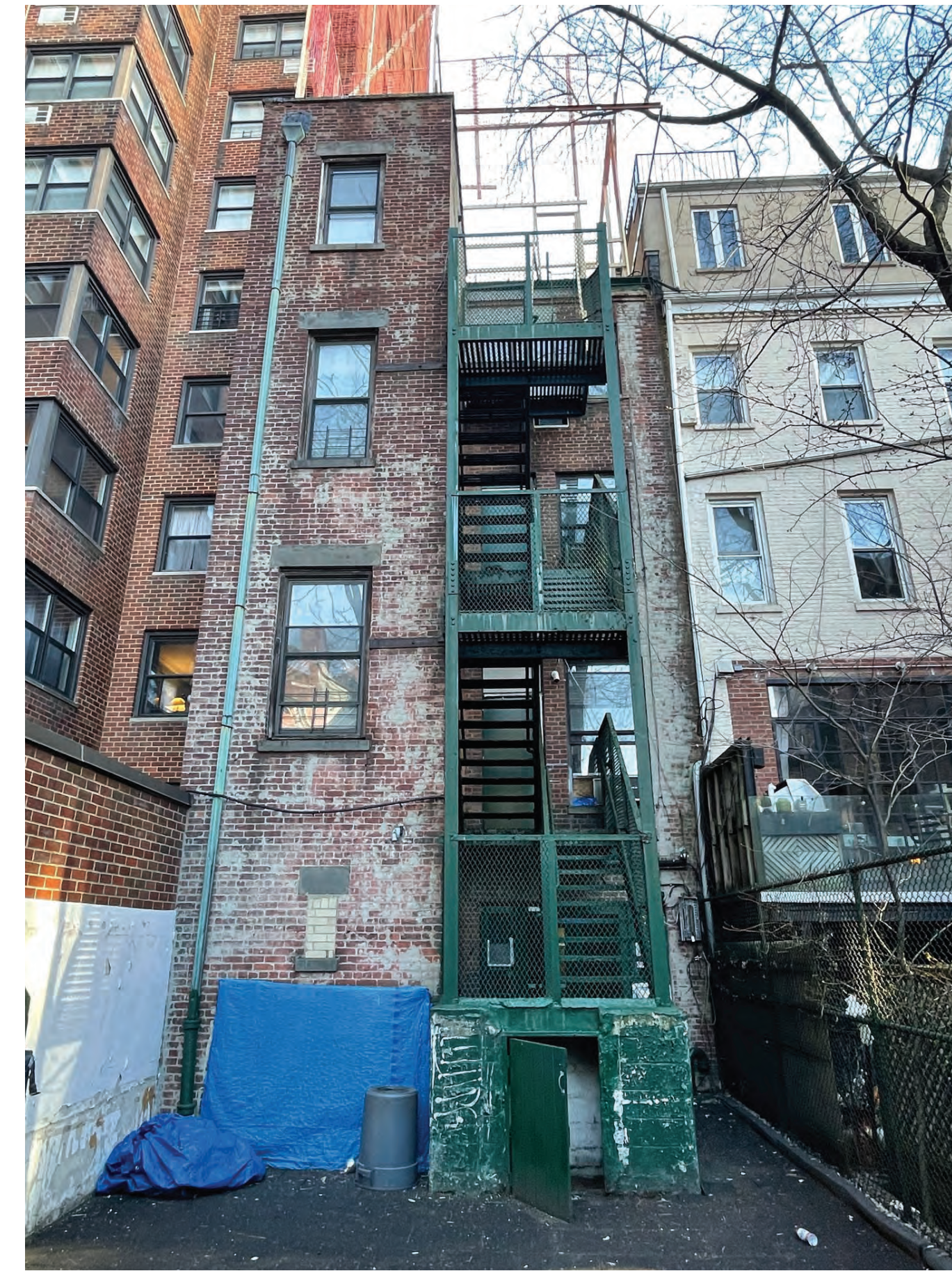
EXISTING REAR FACADE
