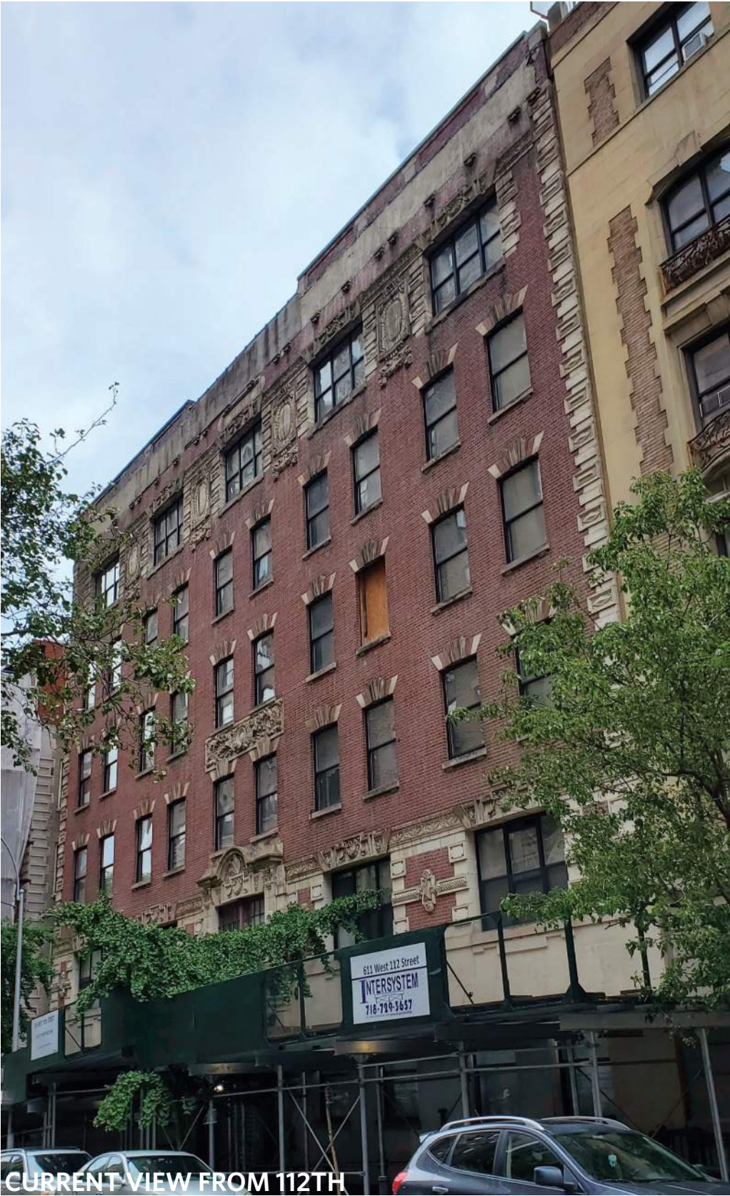
REMOVED CORNICE & RECONFIGURED WINDOWS
