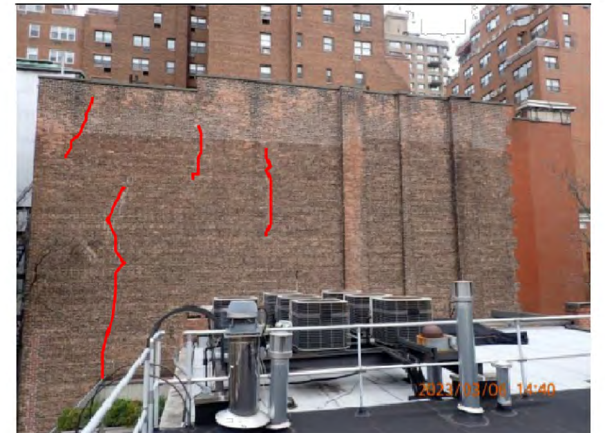
Typical Vertical Cracks in Existing Masonry Wall
