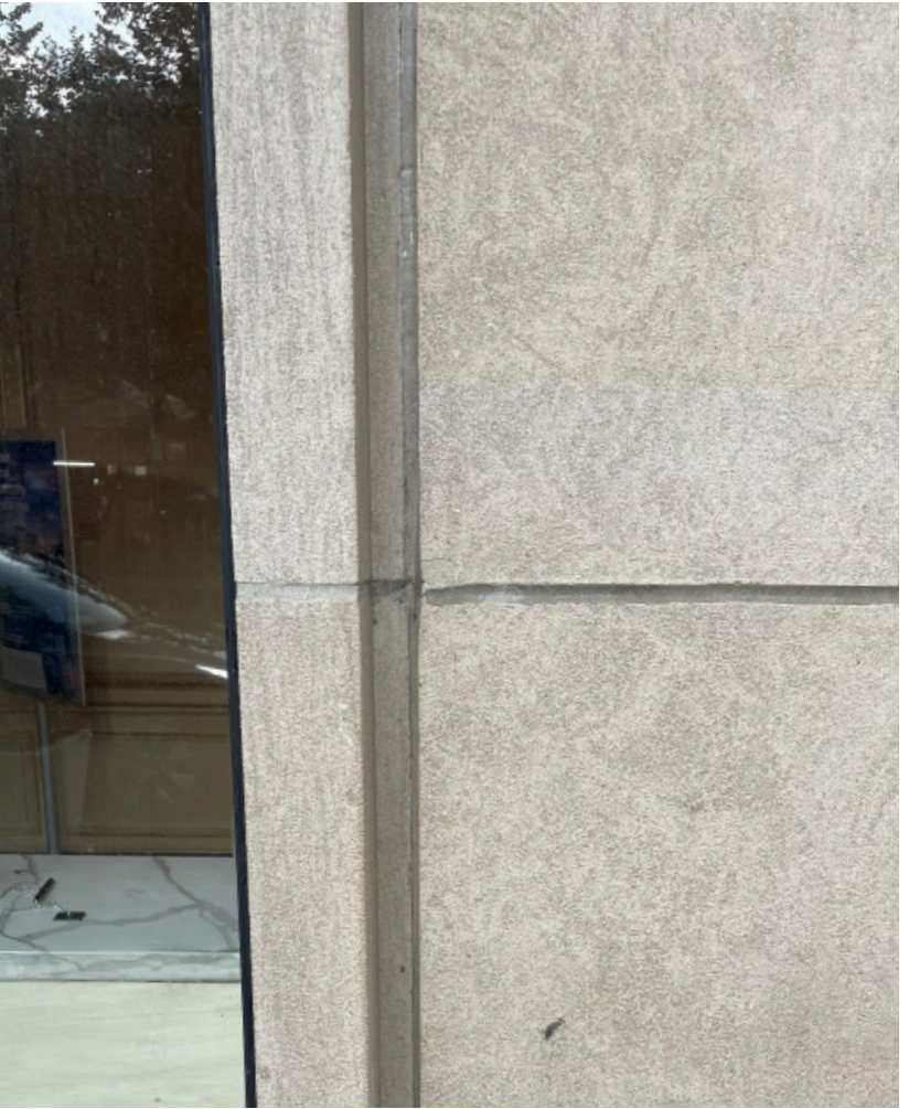
Rough-honed limestone window detail
