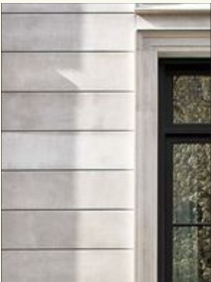
3/8" W x 1/4" D RECESSED SEAMS ON GROUND LEVEL. PHOTO: 48 E 82ND STREET
