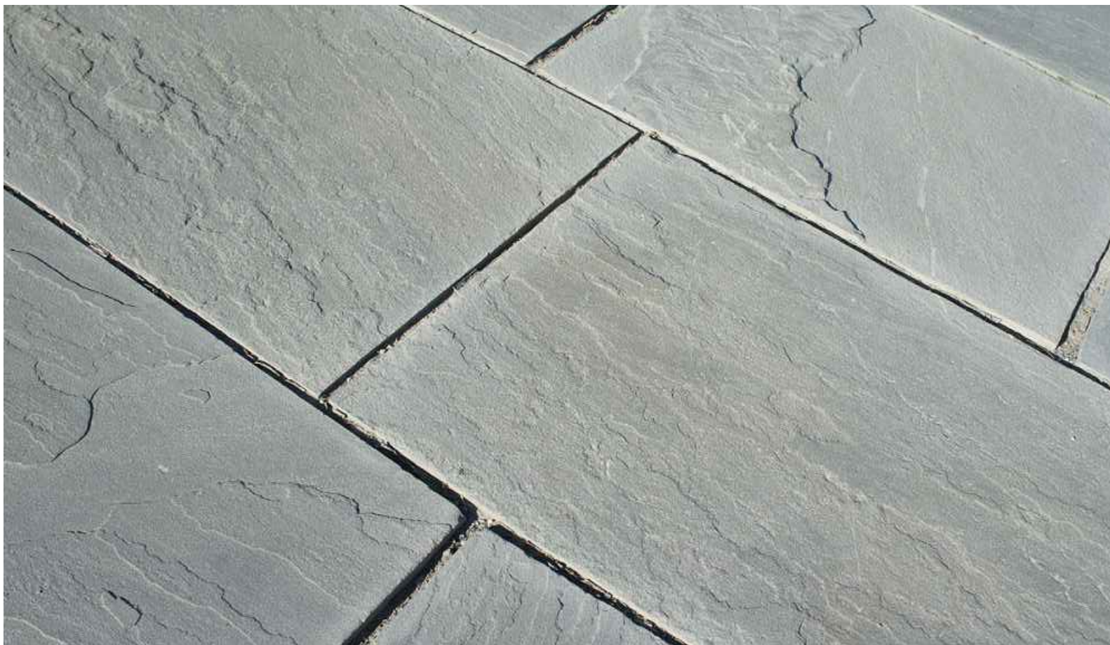
PROPOSED PAVERS: MAKE: NATURAL BLUESTONE SIZE 24X18 COLOR: BLUE SELECT MIX GROUT: BEIGE FINISH: NATURAL CLEFT PATTERN: RUNNING BOND
