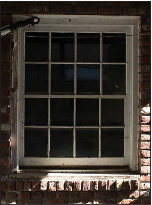
FIRST FLOOR DOUBLE-HUNG WINDOWS
