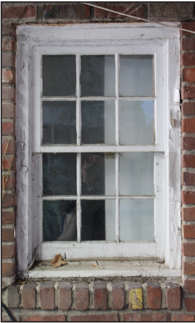
FIRST FLOOR DOUBLE-HUNG WINDOWS
