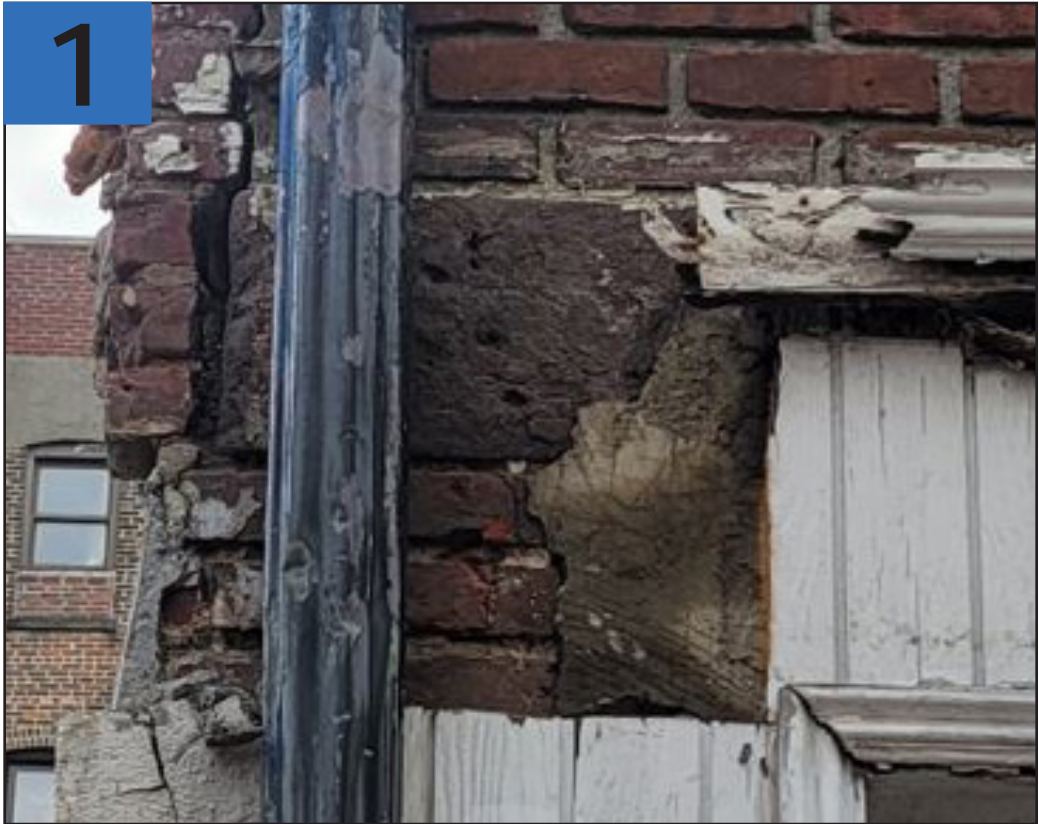
PROBE AT GROUND FLOOR FRONT FACADE LINTEL
