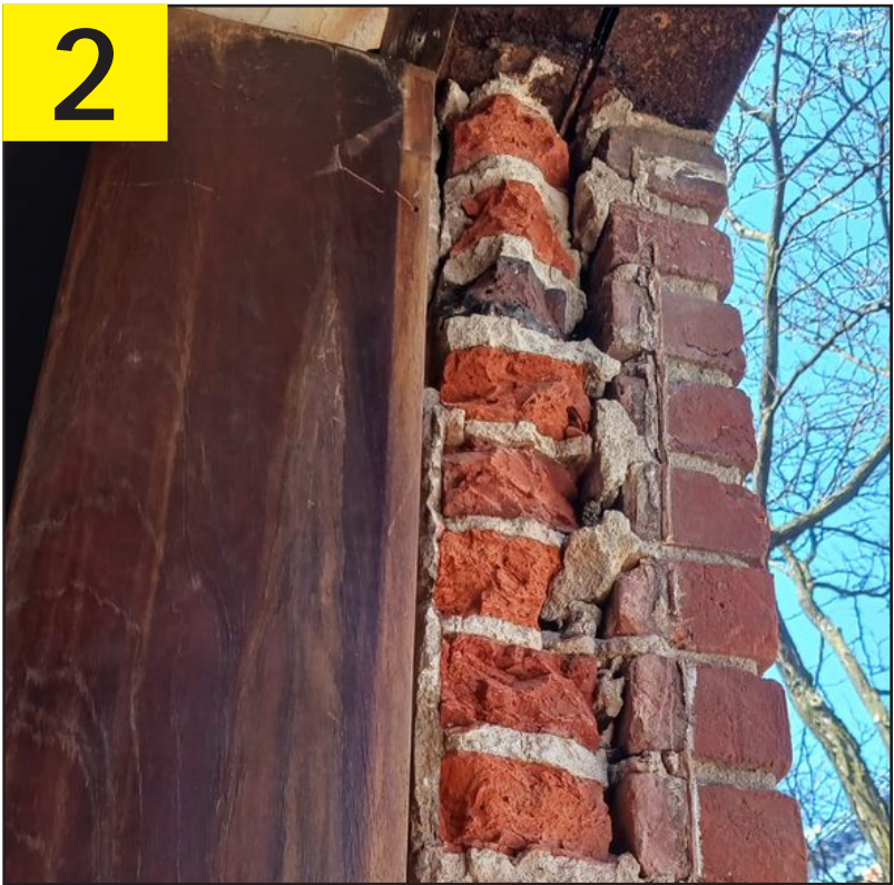
PROBE AT 2ND FLOOR WINDOW SHOWING REPLACED BRICK FACADE
