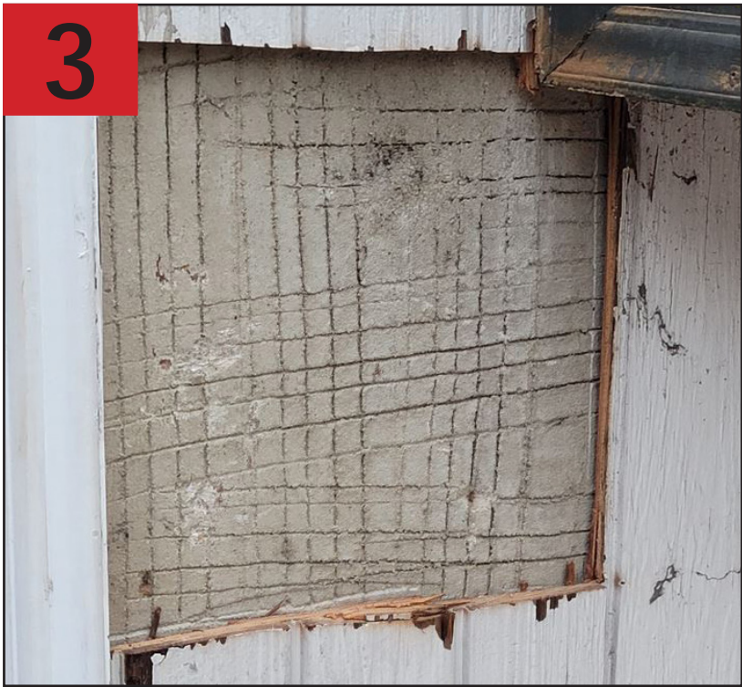
PROBE AT GROUND FLOOR BASE REMOVING WOOD PANELING
