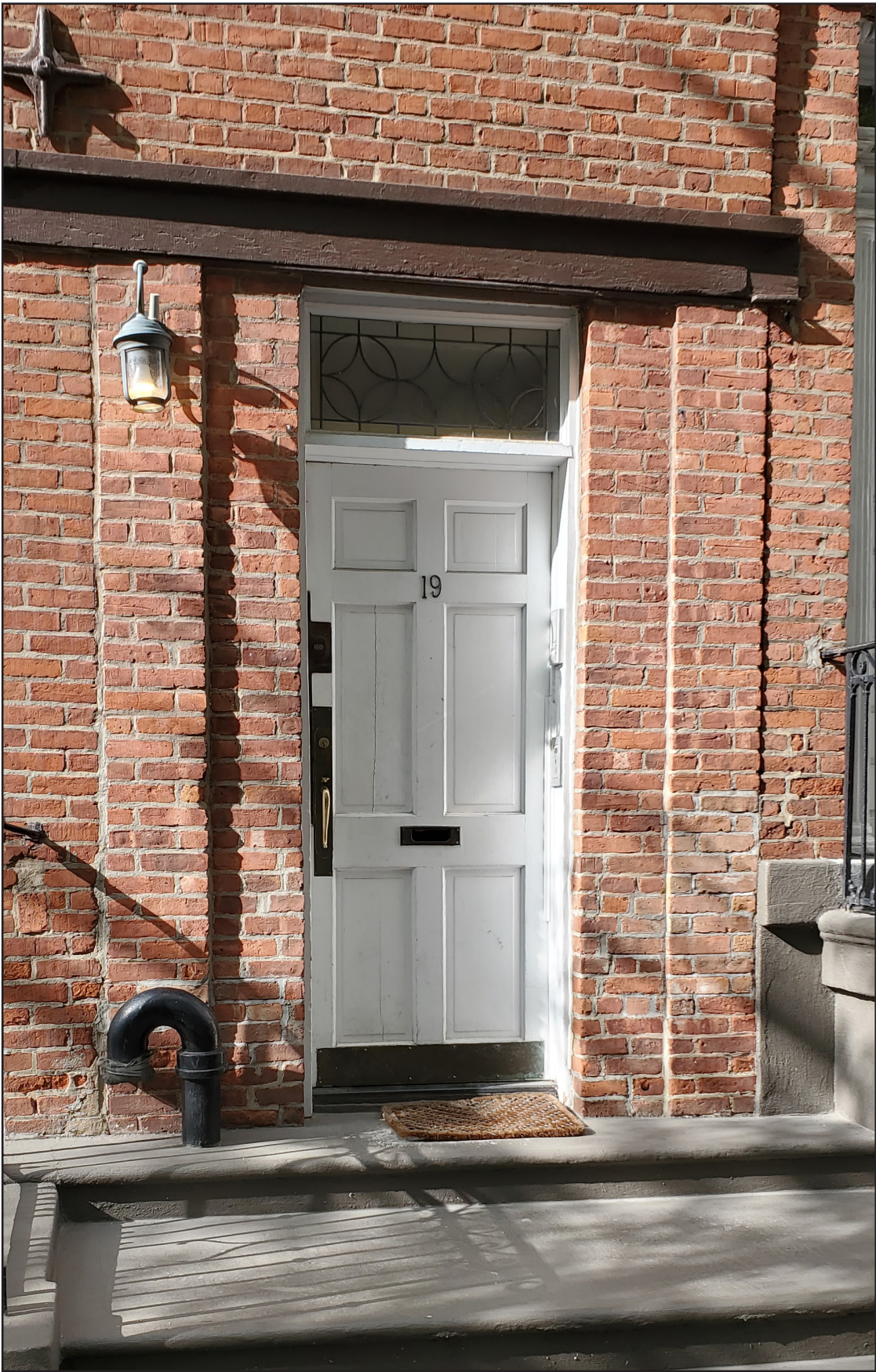
ALTERED FENESTRATION W/ RECESSED BRICK
