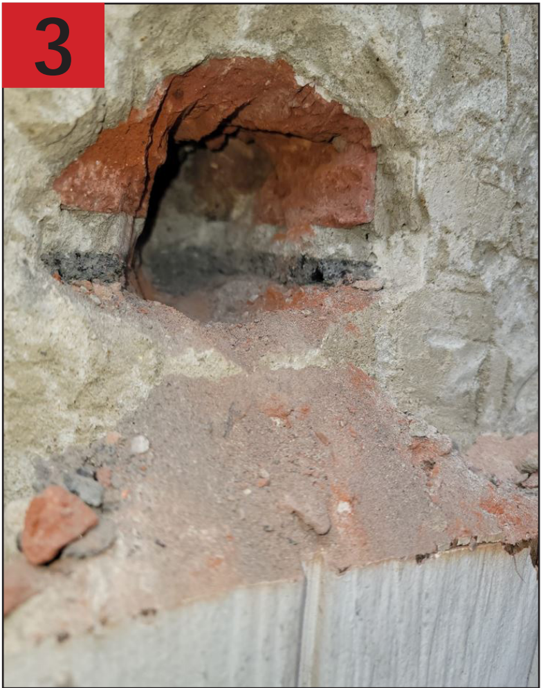
PROBE AT GROUND FLOOR BASE REMOVING SECOND LAYER OF CEMENT PARGING
