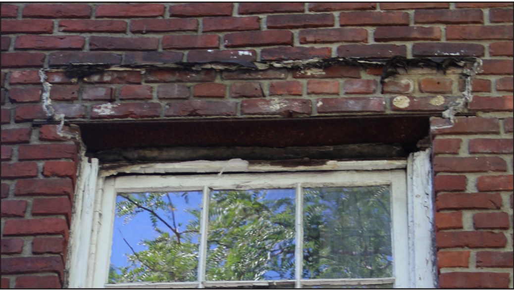
REMOVED NON-HISTORIC 2ND & 3RD FLOOR WOOD LINTEL
