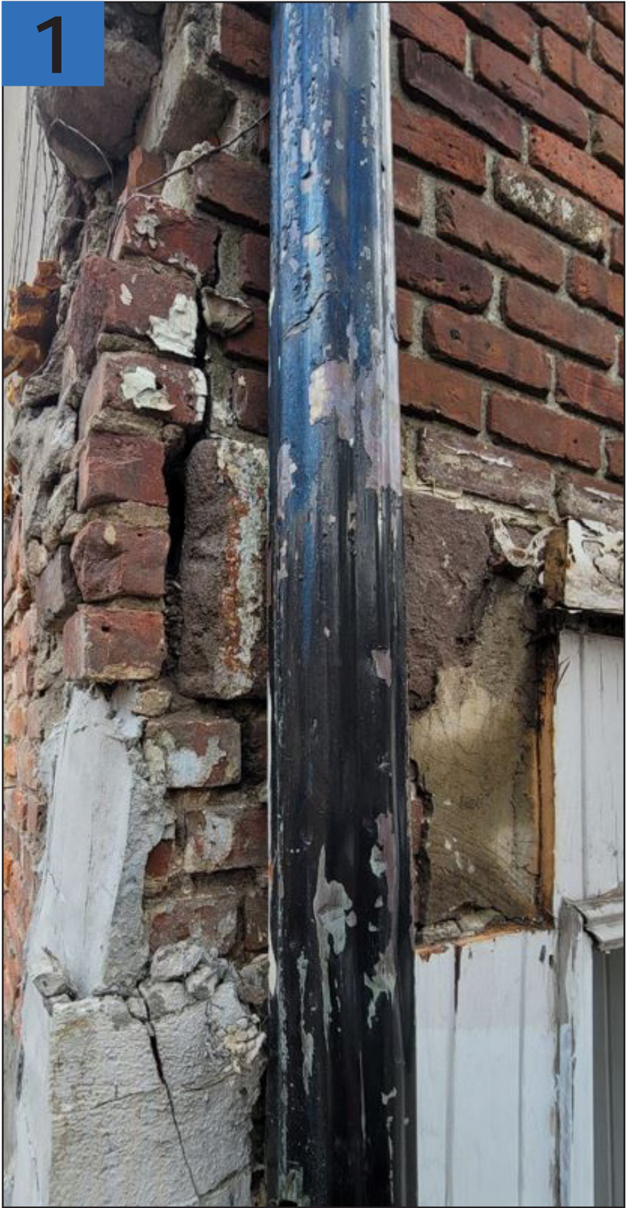
PROBE AT GROUND FLOOR FRONT FACADE LINTEL
