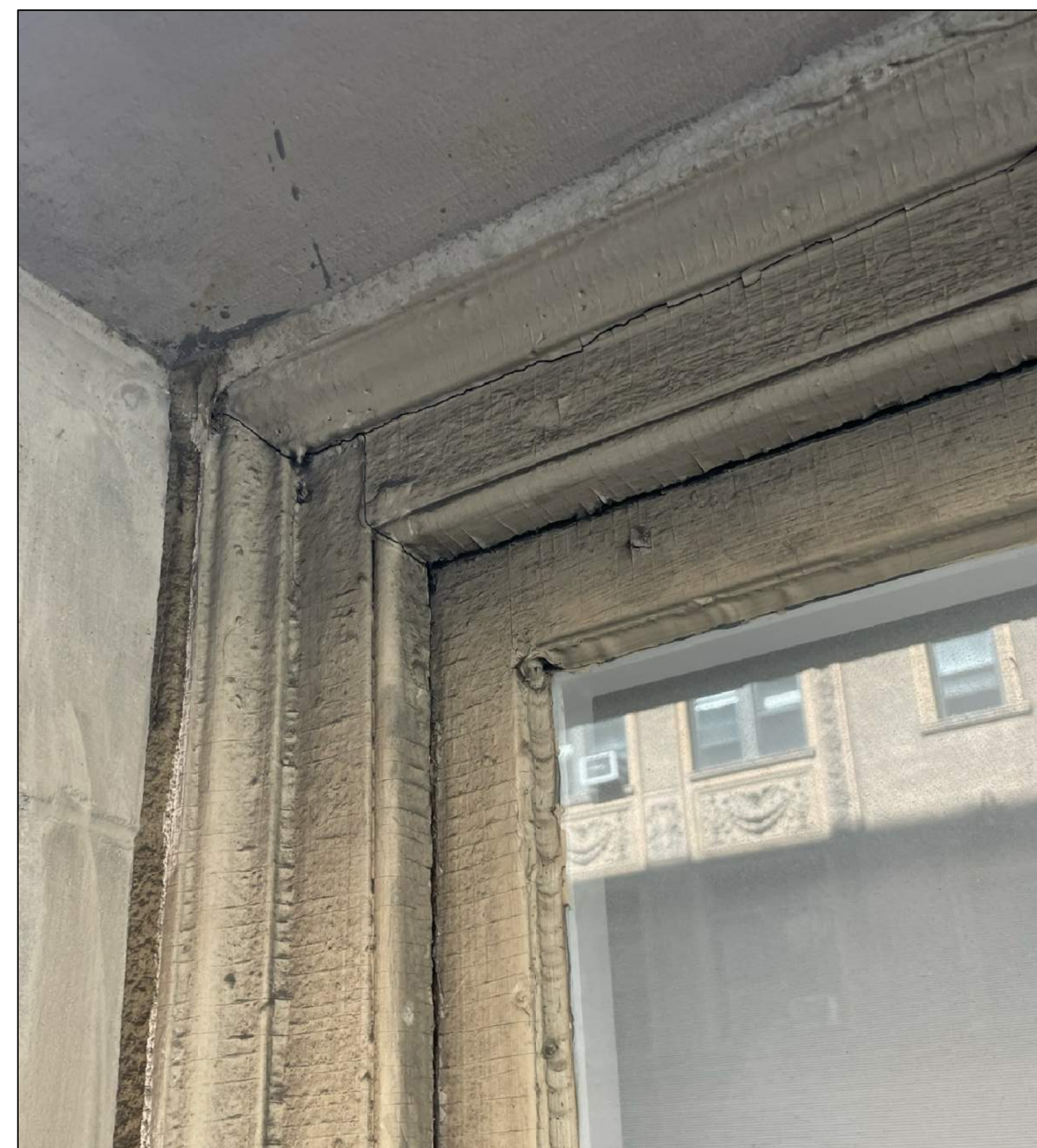
1 EXISTING WOOD BRICKMOLD NTS
