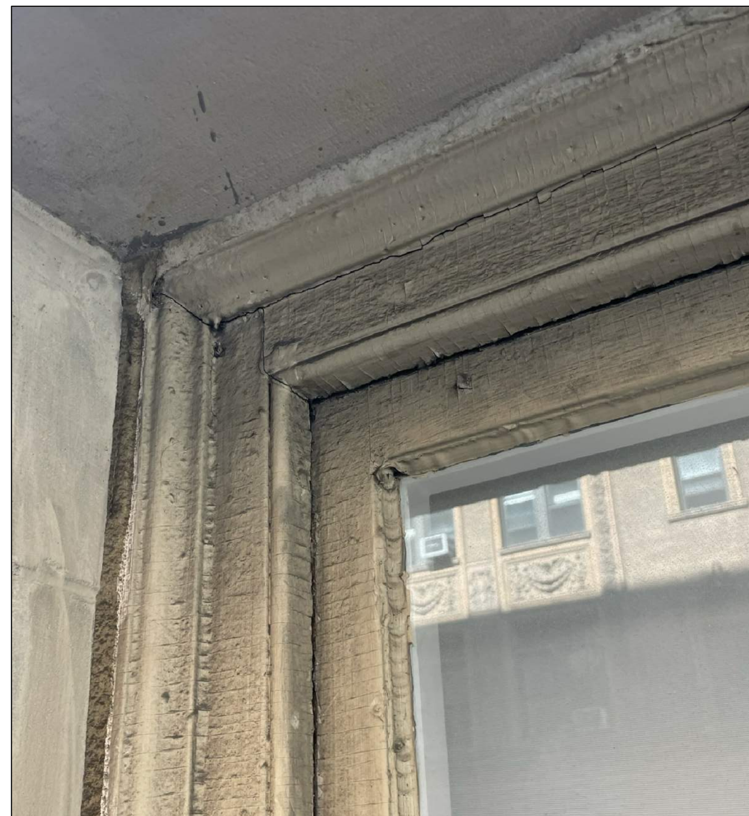
4 EXISTING WOOD BRICKMOLD NTS
