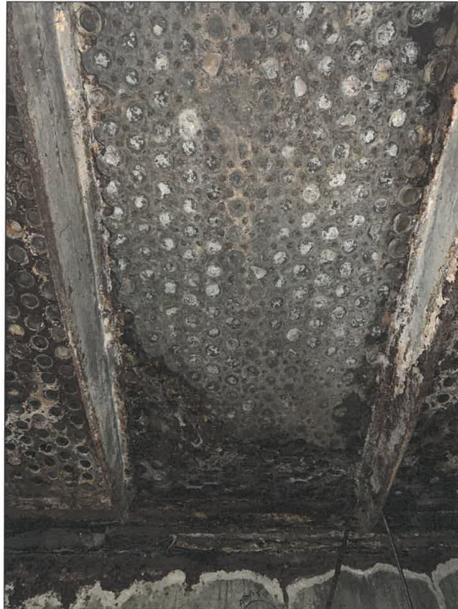
CELLAR VAULT LIGHT PANEL IS CORRODED AND EXTENSIVELY DAMAGE WITH MISSING PORTION OF THE PANEL
