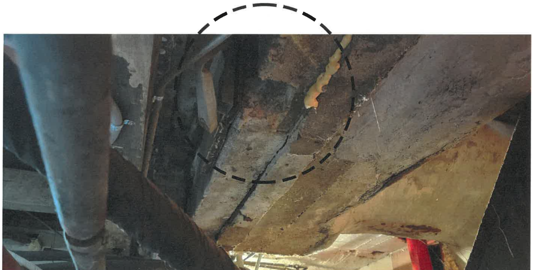
DAMAGE CONCRETE BEAM COMPROMISES THE STRUCTURAL INTEGRITY OF THE BEAM
