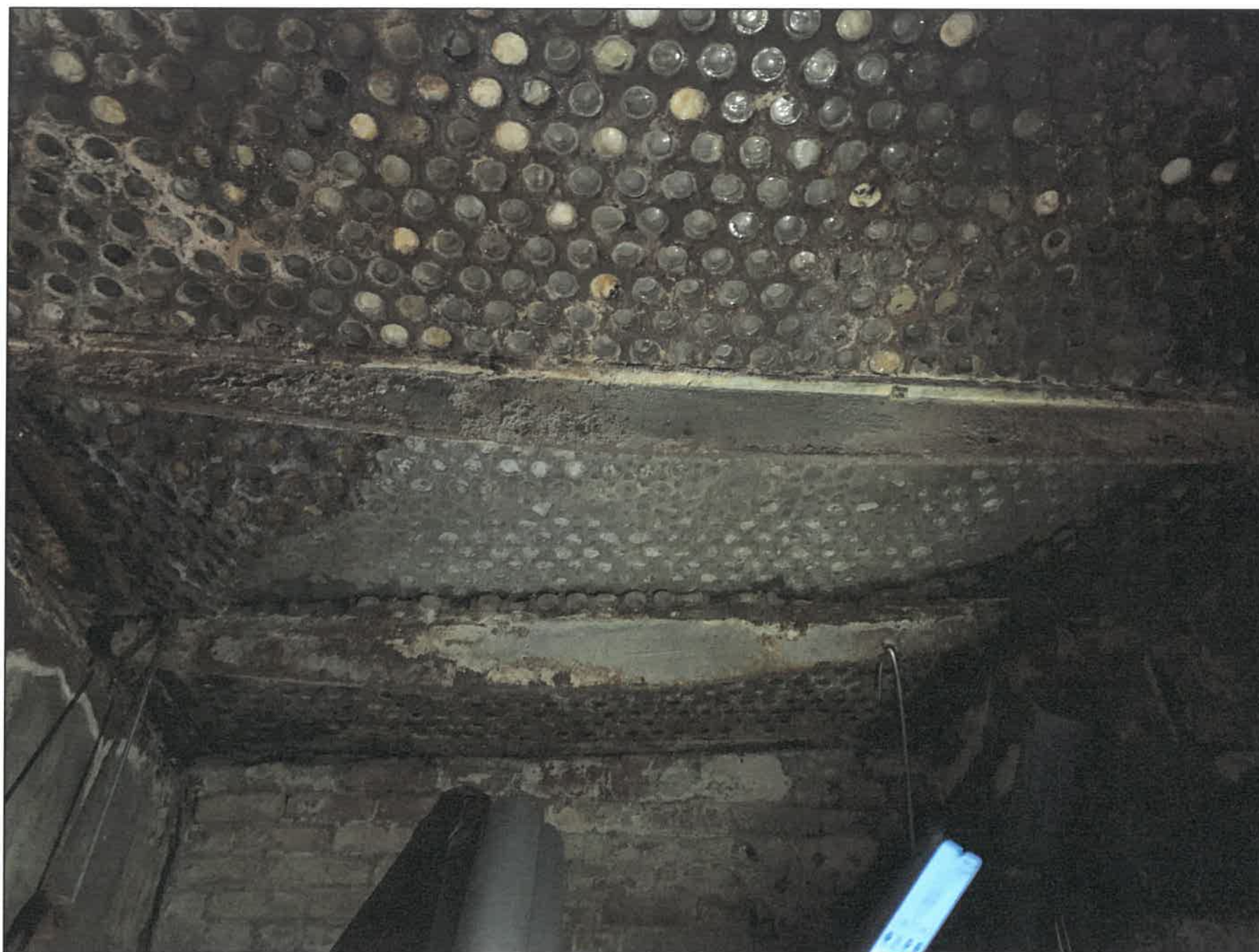
CELLAR VAULT LIGHT PANEL IS CORRODED AND EXTENSIVELY DAMAGE WITH MISSING PORTION OF THE PANEL
