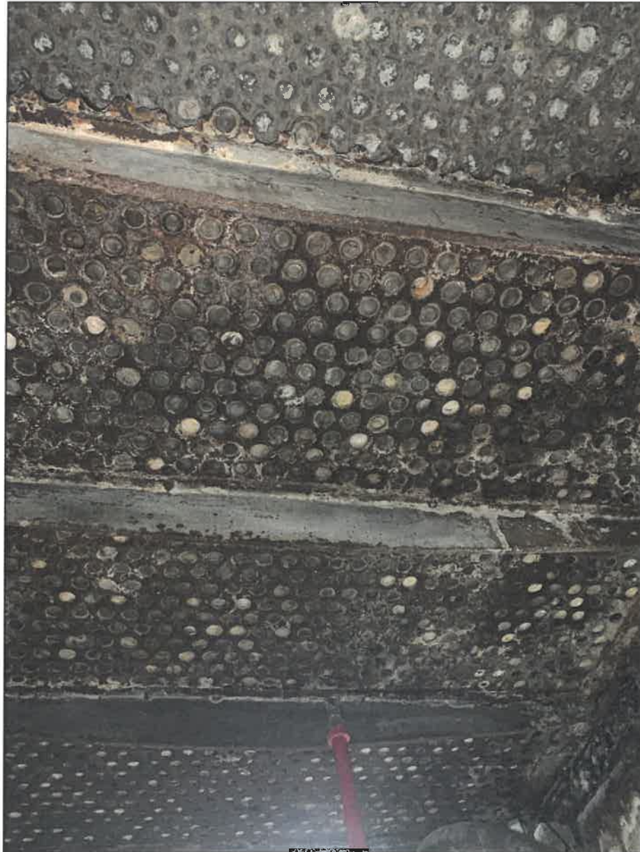
CELLAR VAULT LIGHT PANEL IS CORRODED AND EXTENSIVELY DAMAGE WITH MISSING PORTION OF THE PANEL
