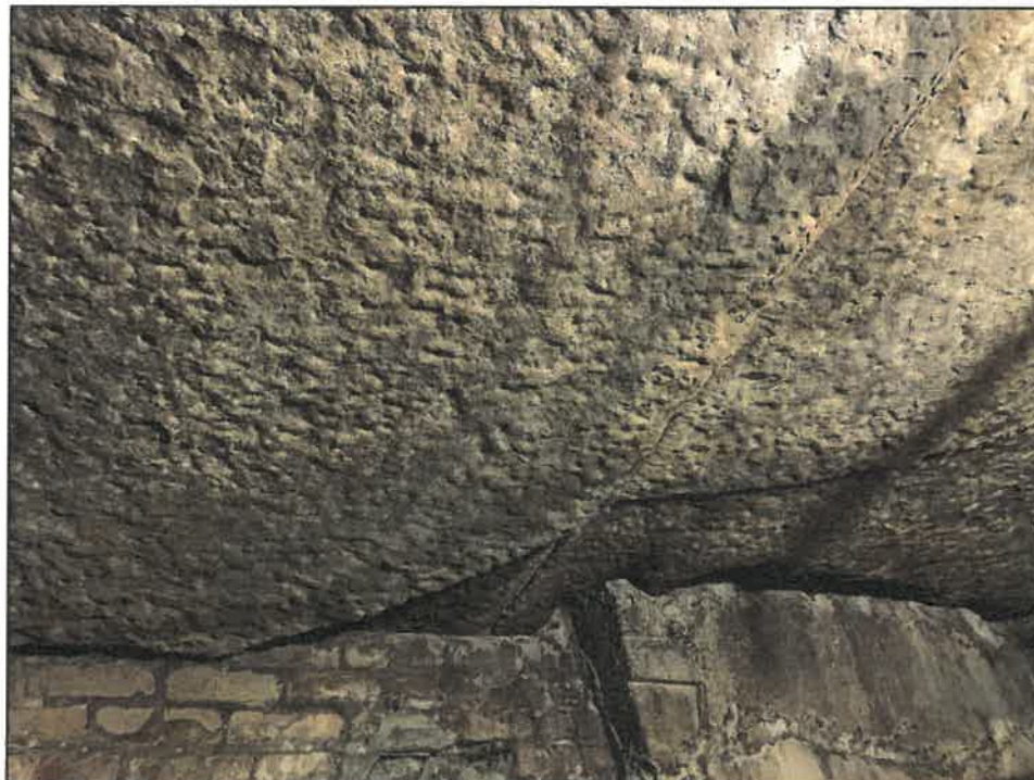
NOTABLE WATER LEAK DAMAGE, EROSION OF JOINTS AND SIGNS OF STRESS AND MATERIAL FATIGUE AT THE SLAB (GRANITE)
