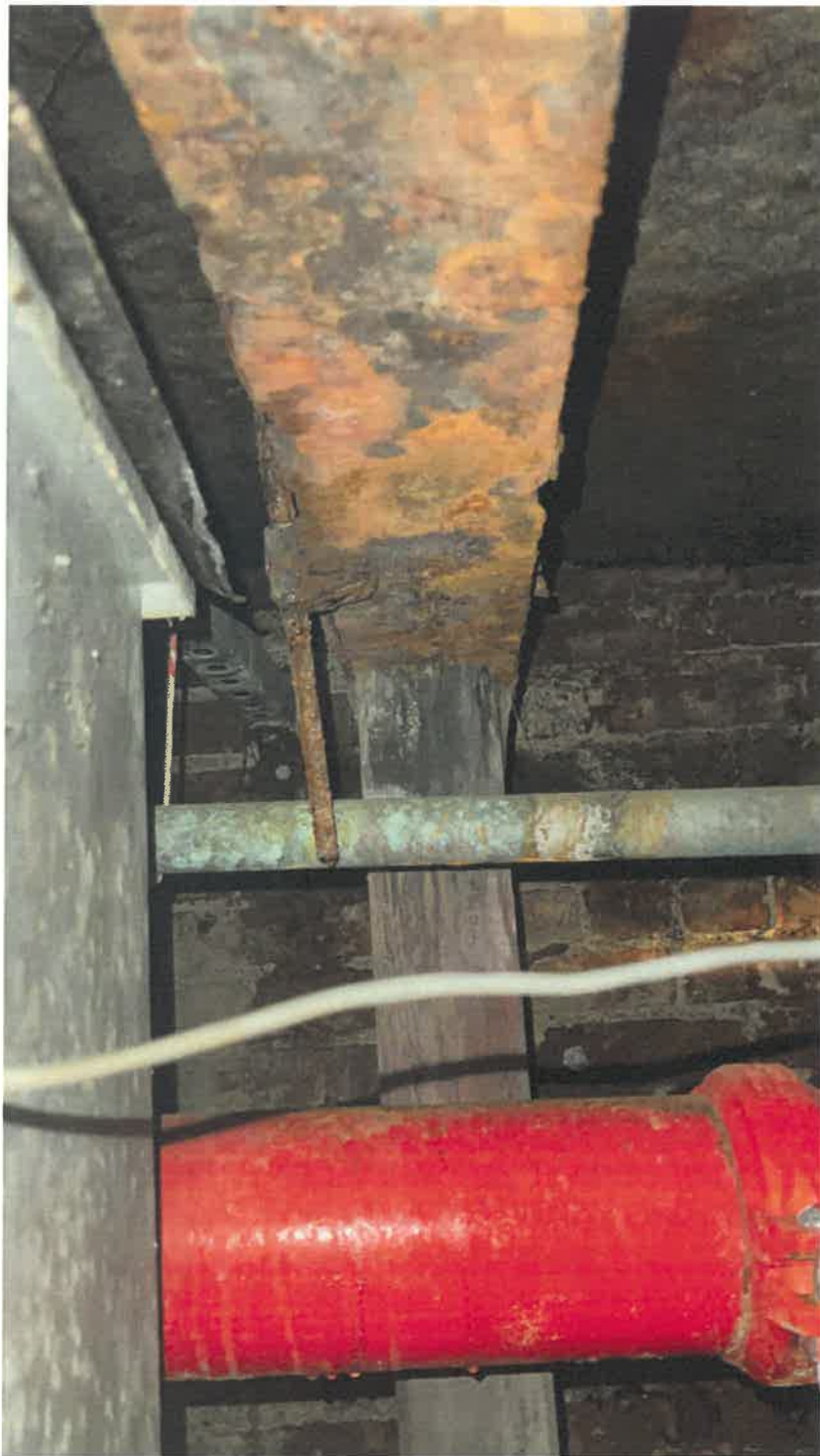
DETERIORATED STEEL BEAM BRACING WITH WOOD COLUMN SUPPORTING THE DILAPIDATED SLAB ABOVE.
