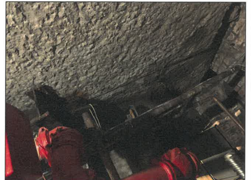
NOTABLE WATER LEAK DAMAGE, EROSION OF JOINTS AND SIGNS OF STRESS AND MATERIAL FATIGUE AT THE SLAB (GRANITE)
