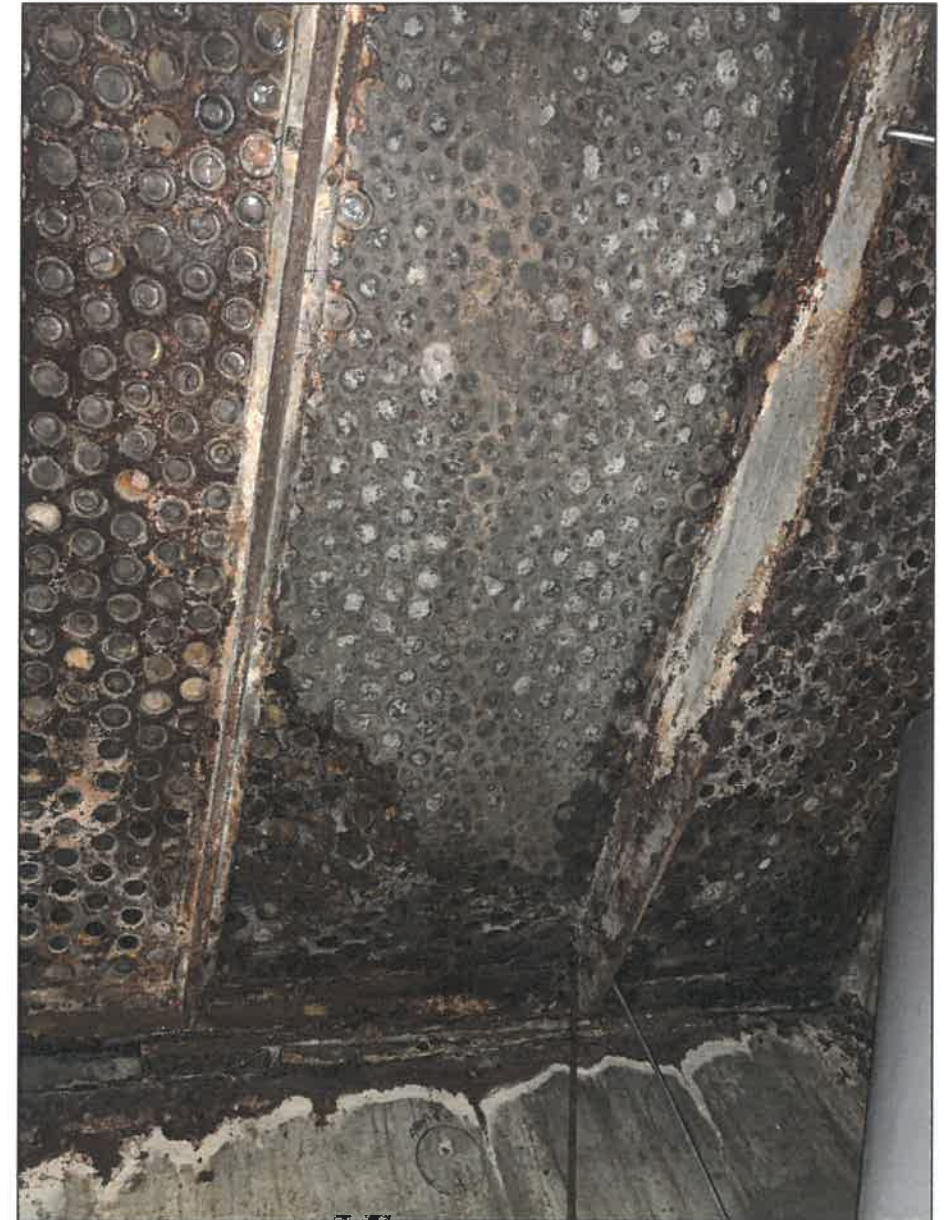
CELLAR VAULT LIGHT PANEL IS CORRODED AND EXTENSIVELY DAMAGE WITH MISSING PORTION OF THE PANEL
