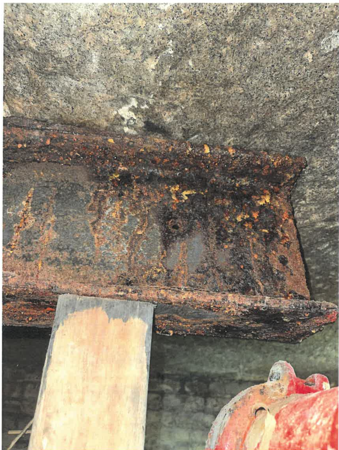
WOOD COLUMN SUPPORTING THE STEEL BEAM
