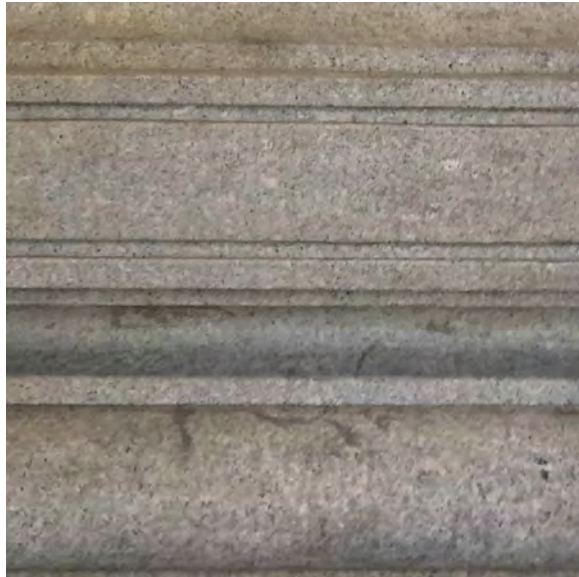
GRANITE PLINTH BASE: STONE SELECTED TO MATCH EXISTING GRANITE
