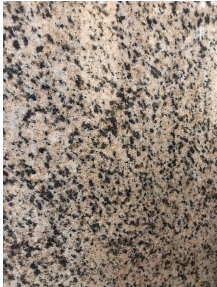
EXISTING GRANITE STONE AT MAIN ENTRY FLOOR FINISH
