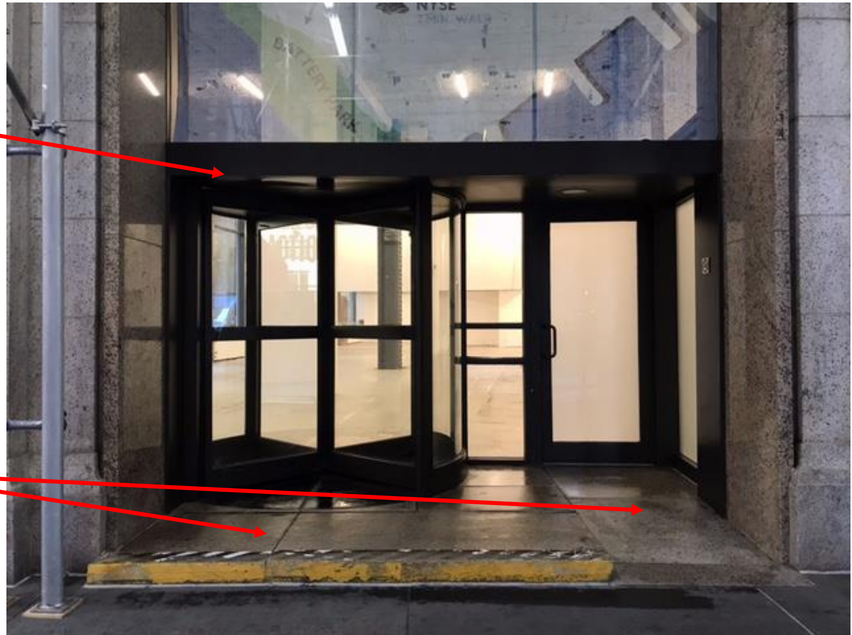
EXISTING ENTRY – REVOLVING DOOR AND SINGLE SWINGING DOOR – DARK BRONZE FINISH
