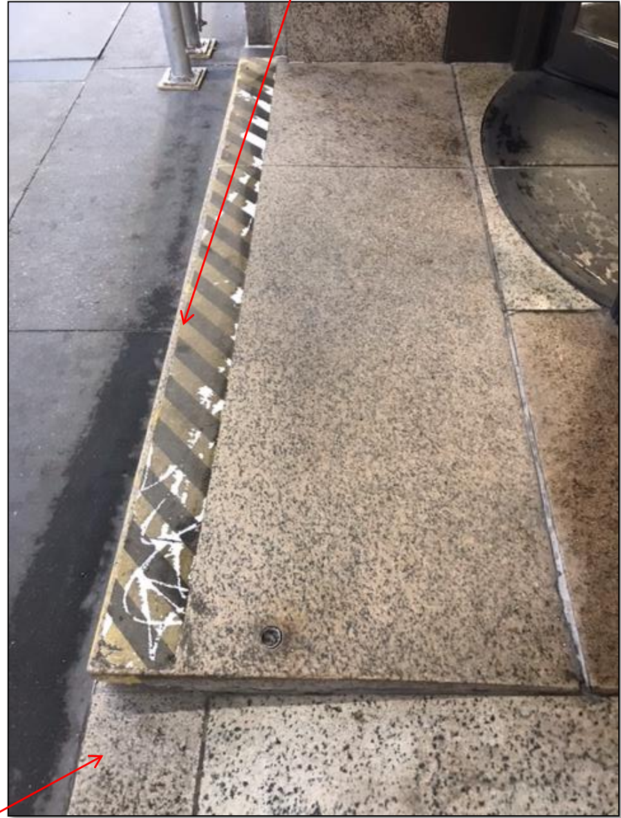
C NORTHEAST FAÇADE ENTRANCE – EXISTING RAMP AND STEP
