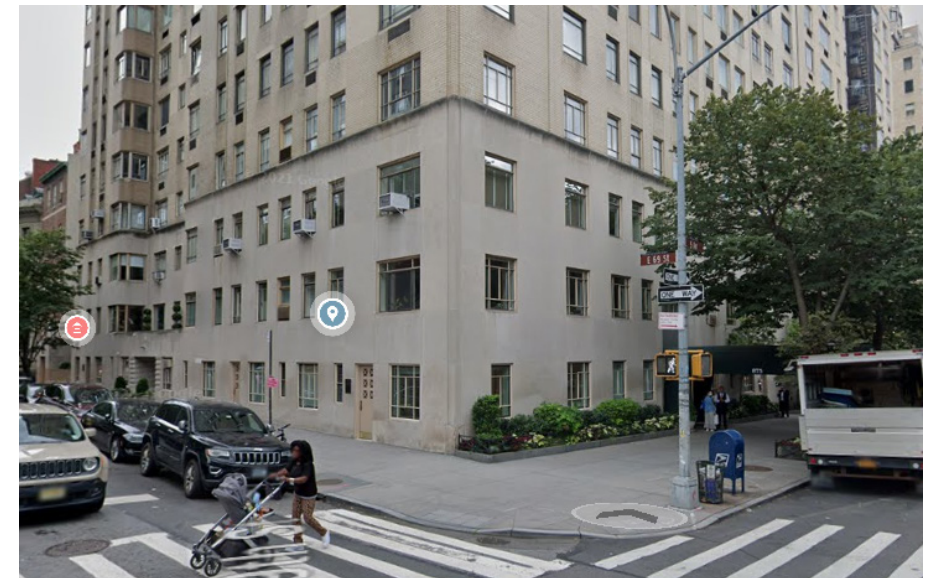
5th Avenue and 69th Street (875 5th Avenue) Three story base expression; entry on 5th Ave.
