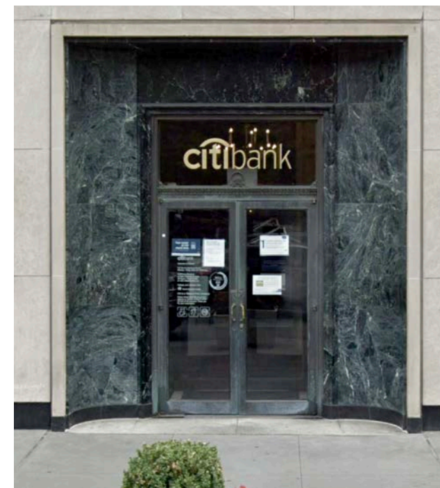
Existing Citibank entry
