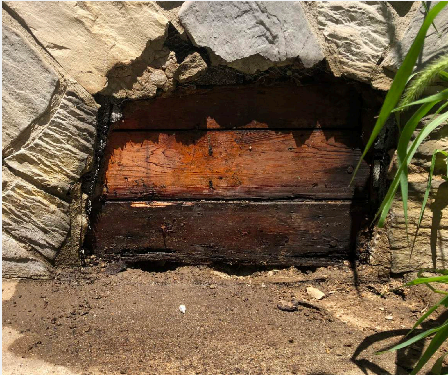
Facade probe below porch - shiplap siding
