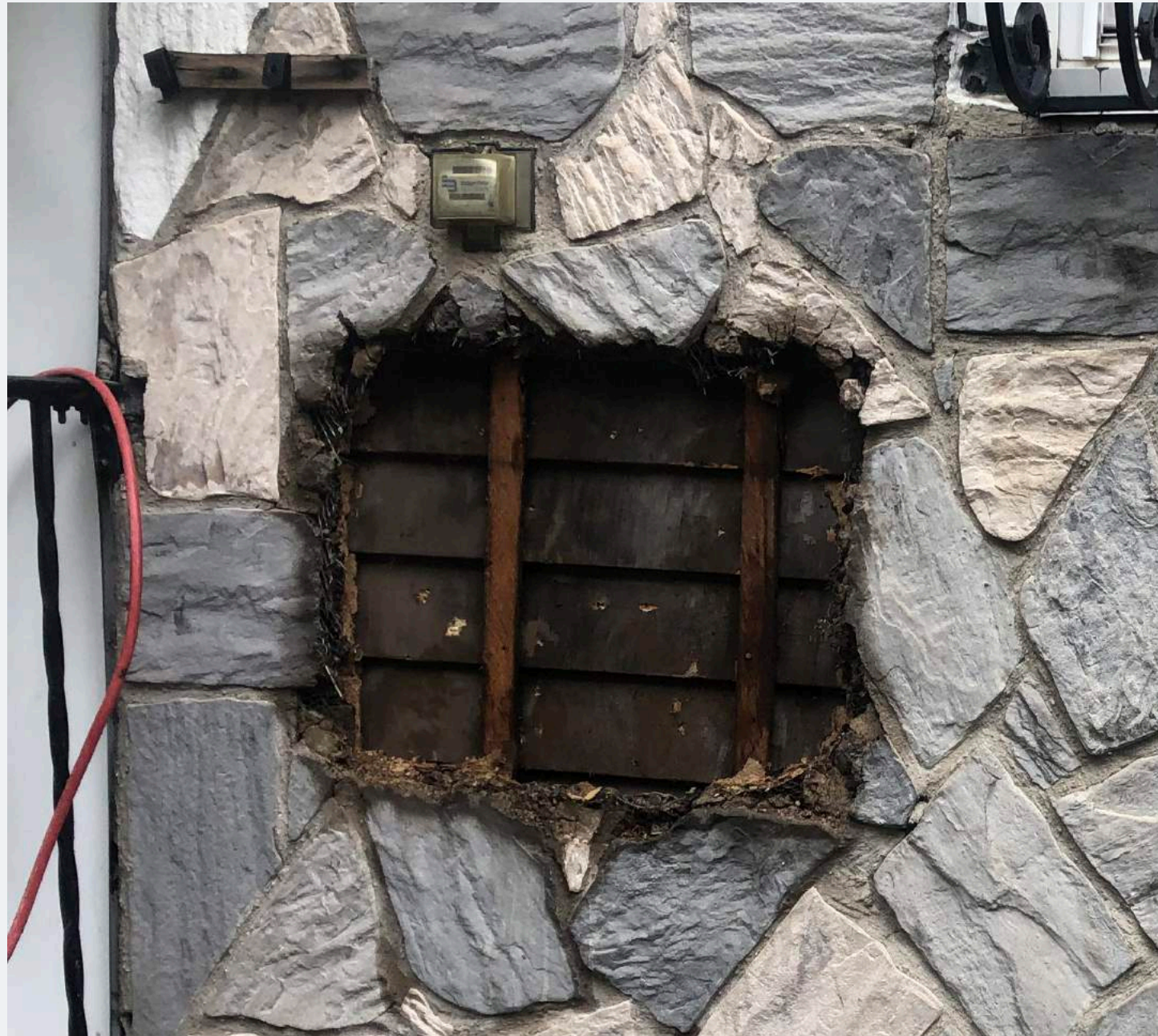
Facade probe above porch - clapboard siding
