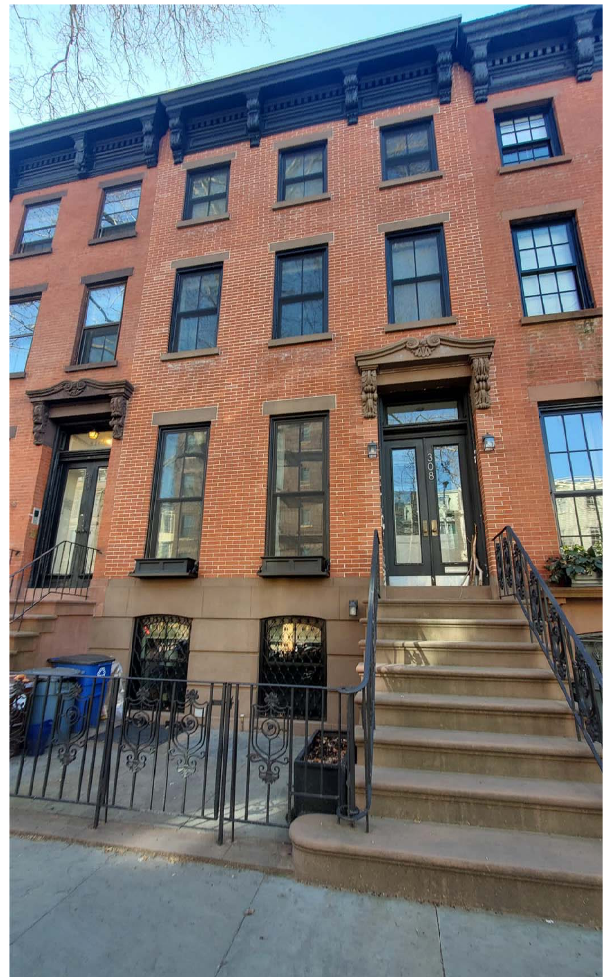
308 Cumberland Installed approved 2 over 2 aluminum clad windows
