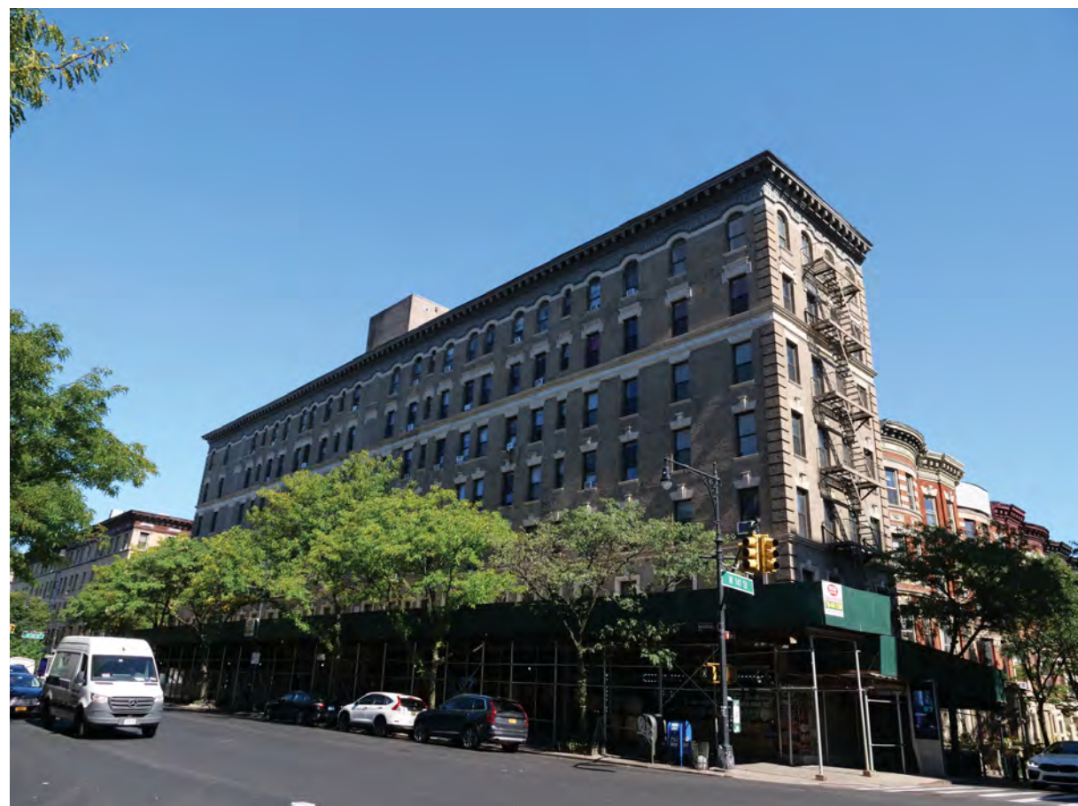
WEST ELEVATION AND CONTEXT FROM AMSTERDAM AVENUE LOOKING NORTH EXISTING
