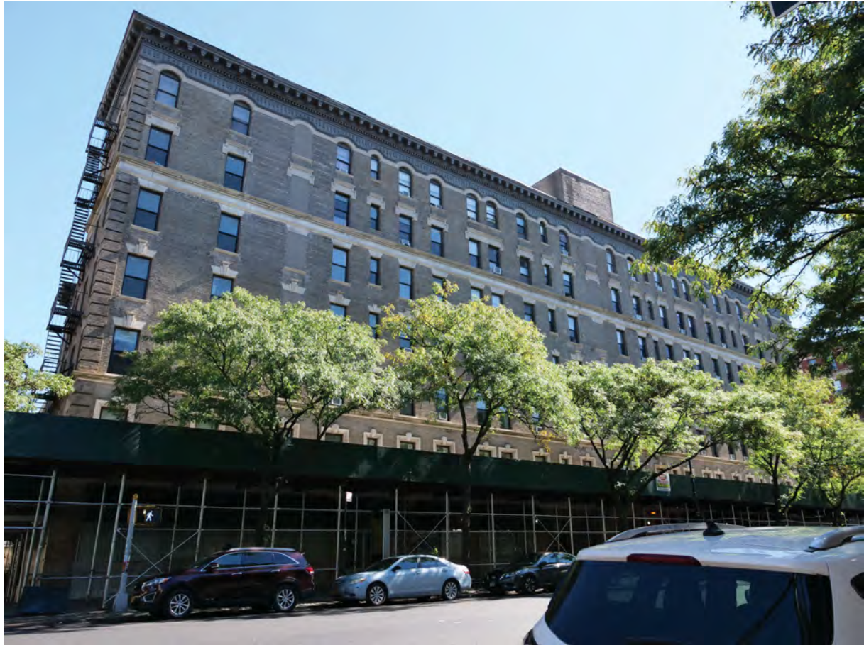
WEST ELEVATION AND CONTEXT FROM AMSTERDAM AVENUE LOOKING SOUTH
