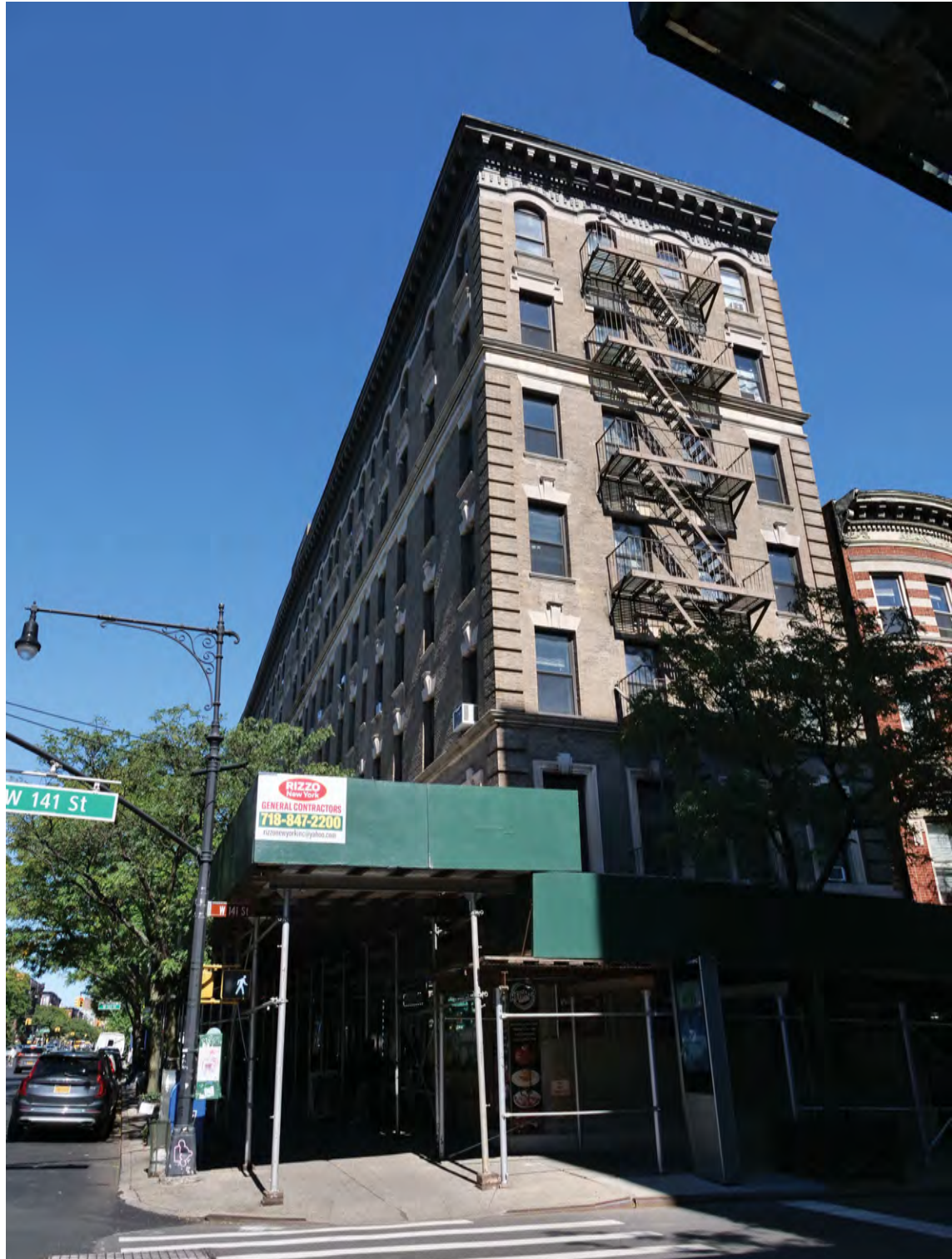
SOUTH ELEVATION FROM 141ST STREET
