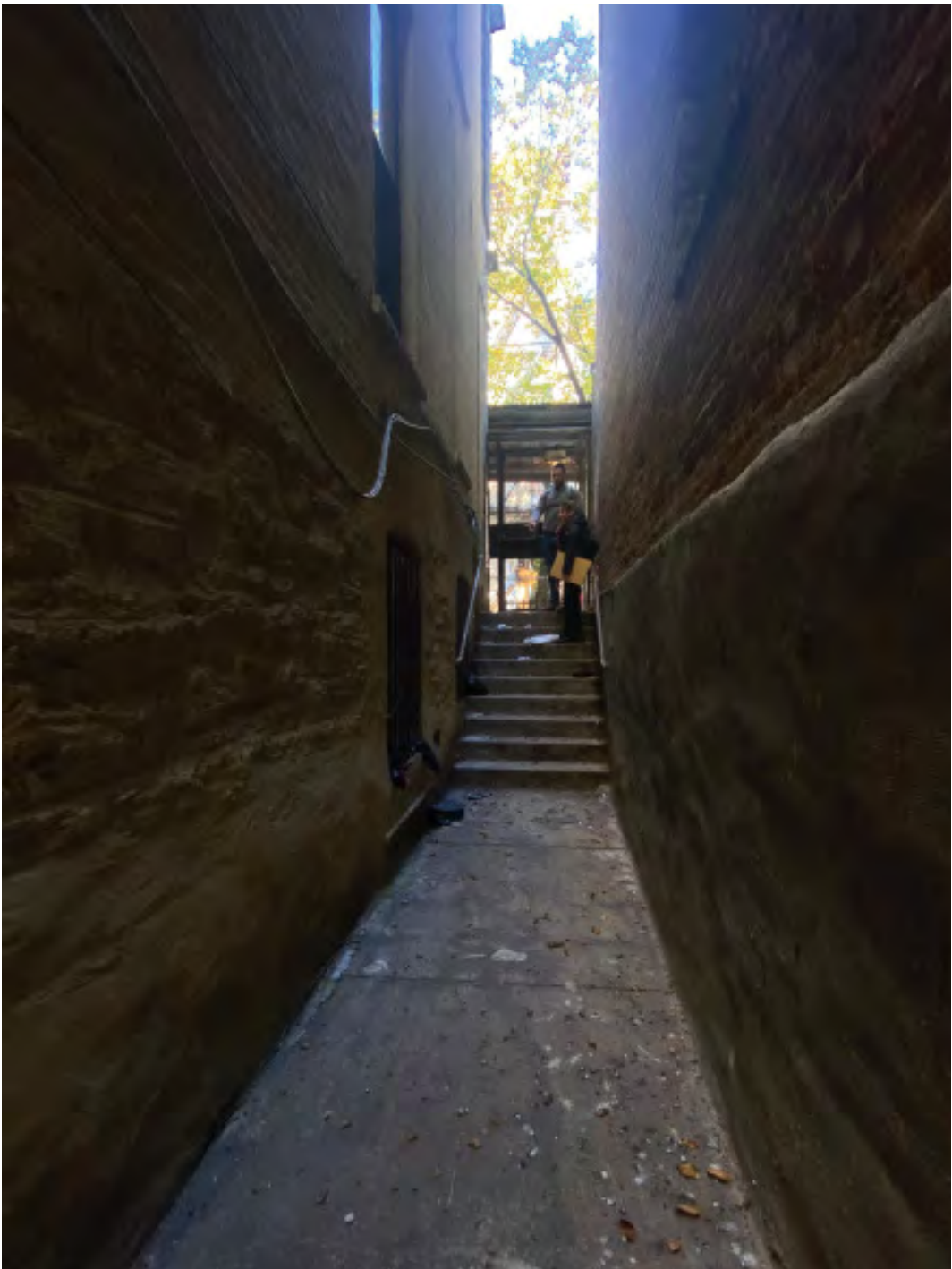
NORTH WING REAR ELEVATION/YARD
