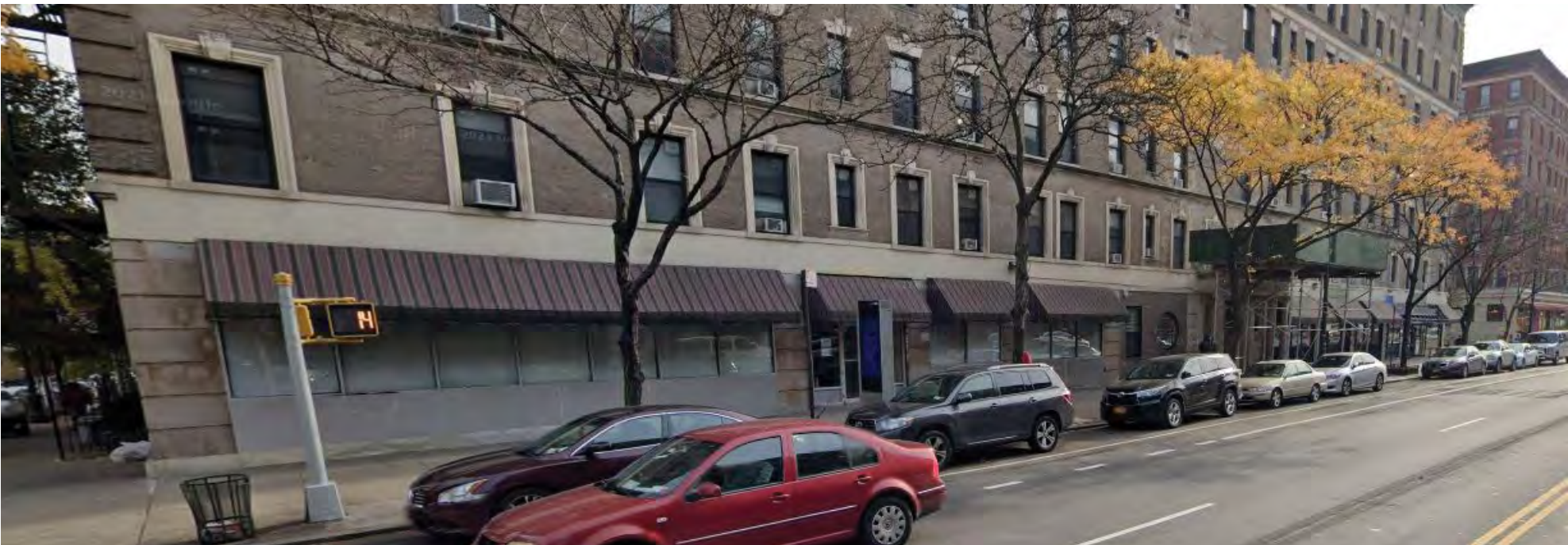
WEST ELEVATION AND CONTEXT FROM AMSTERDAM AVENUE LOOKING SOUTH
