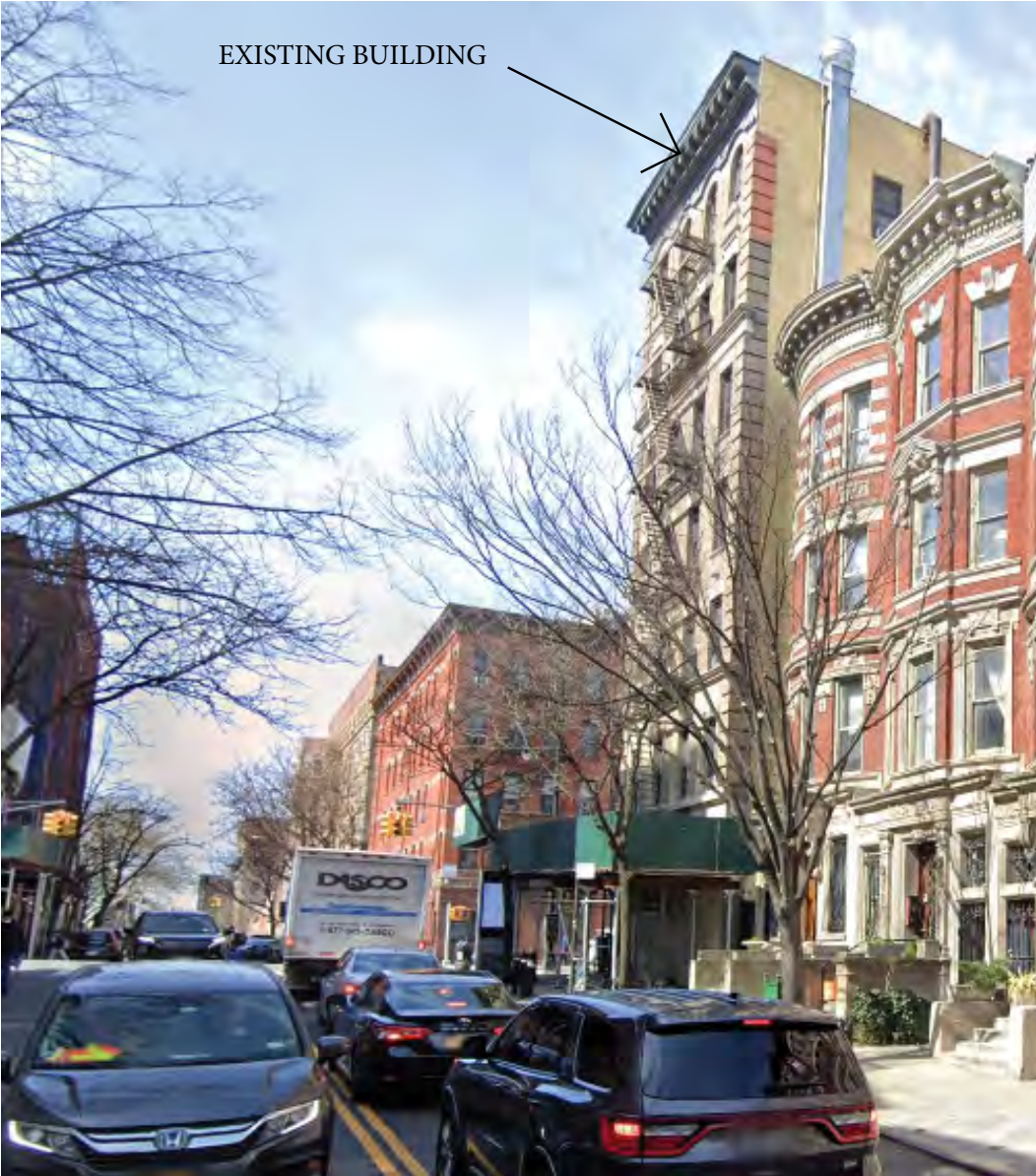
NORTH WING REAR FACADE FROM 141ST STREET LOOKING WEST
