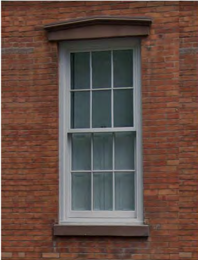
LIGHT GREY DOUBLE HUNG WINDOWS WITH CAST STONE HEADERS TO MATCH HISTORICAL PROFILE.
