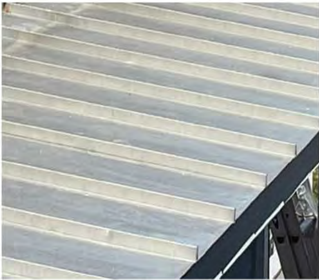
ZINC COATED COPPER STANDING SEAM ROOF.
