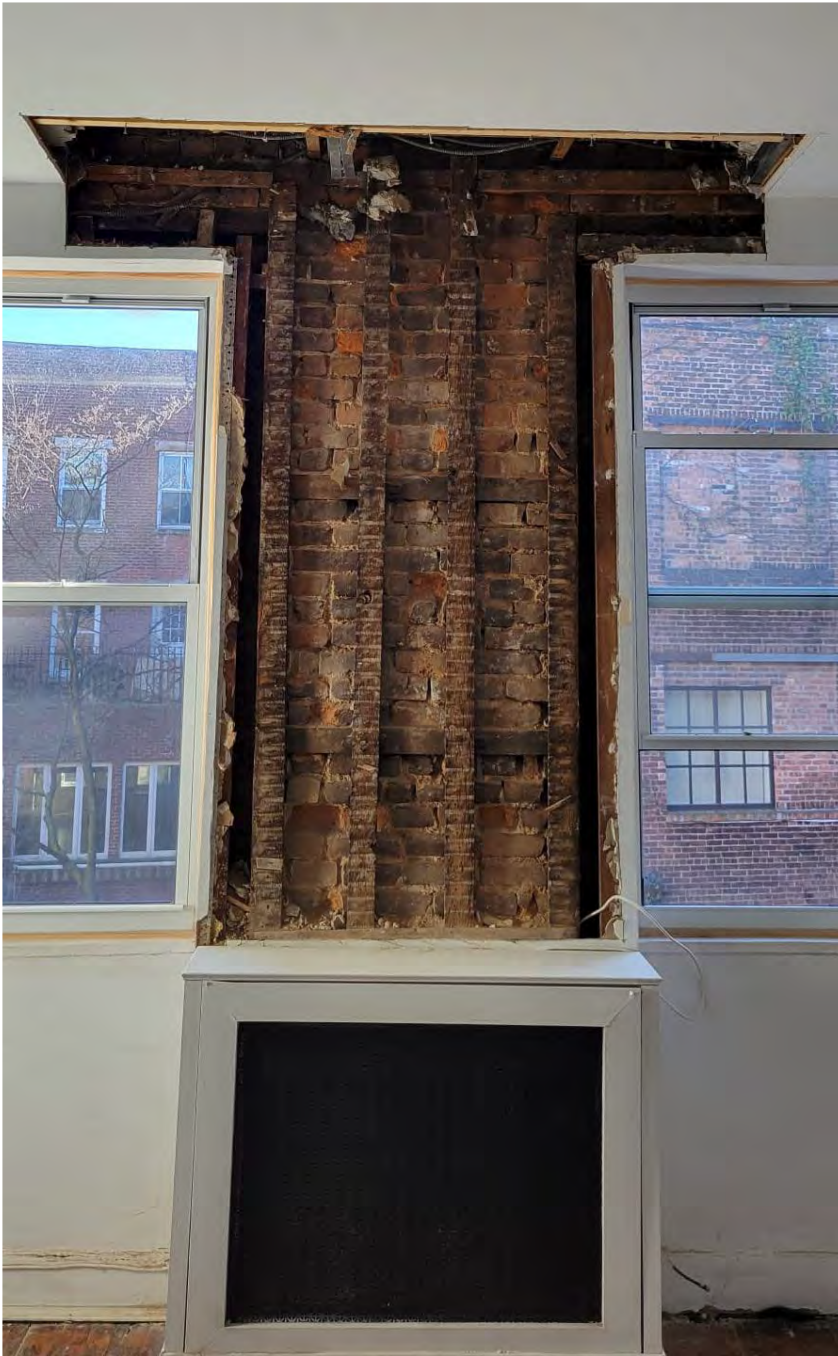
2 PROBE AT REAR WALL ON SECOND FLOOR NTS
