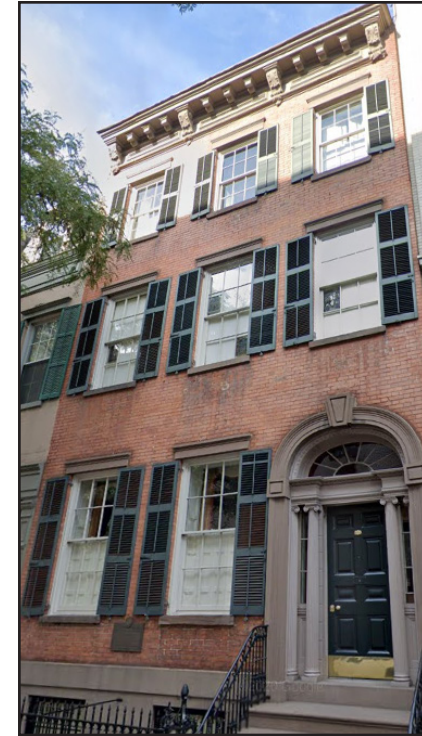
205 PRINCE ST TRANSITIONAL FEDERAL/GREEK REVIVAL
