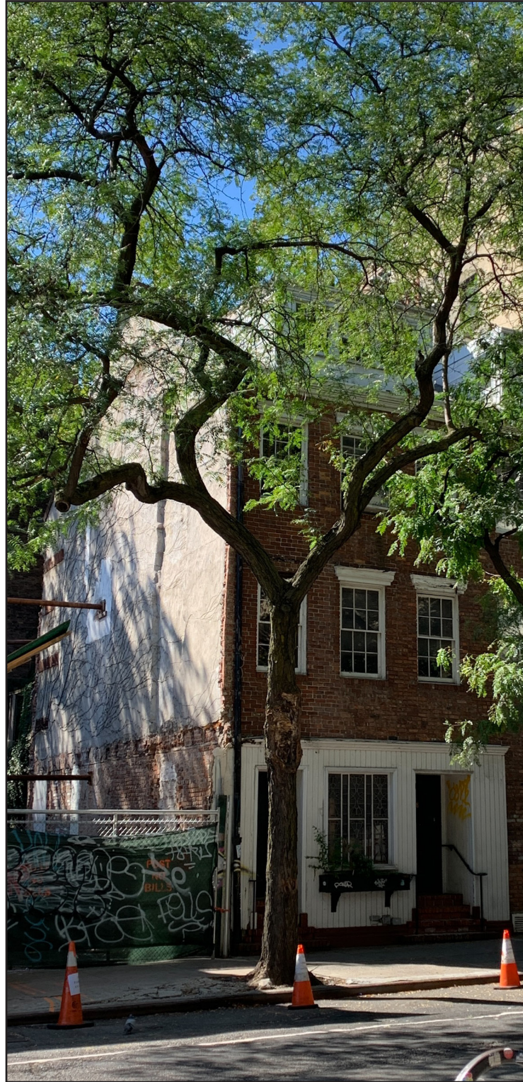
PHOTO 1 FRONT VIEW LOOKING SOUTHWEST
