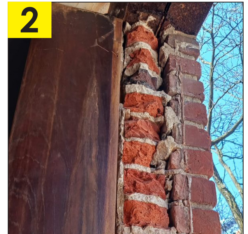
PROBE AT 2ND FLOOR WINDOW SHOWING REPLACED BRICK FACADE
