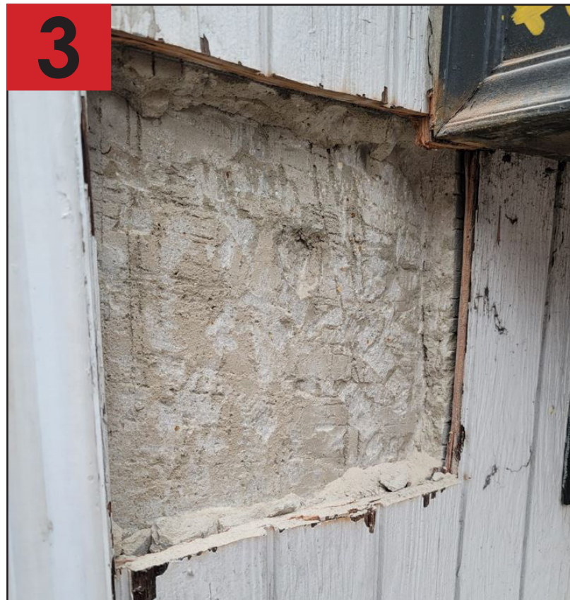
PROBE AT GROUND FLOOR BASE REMOVING FIRST LAYER OF CEMENT PARGING
