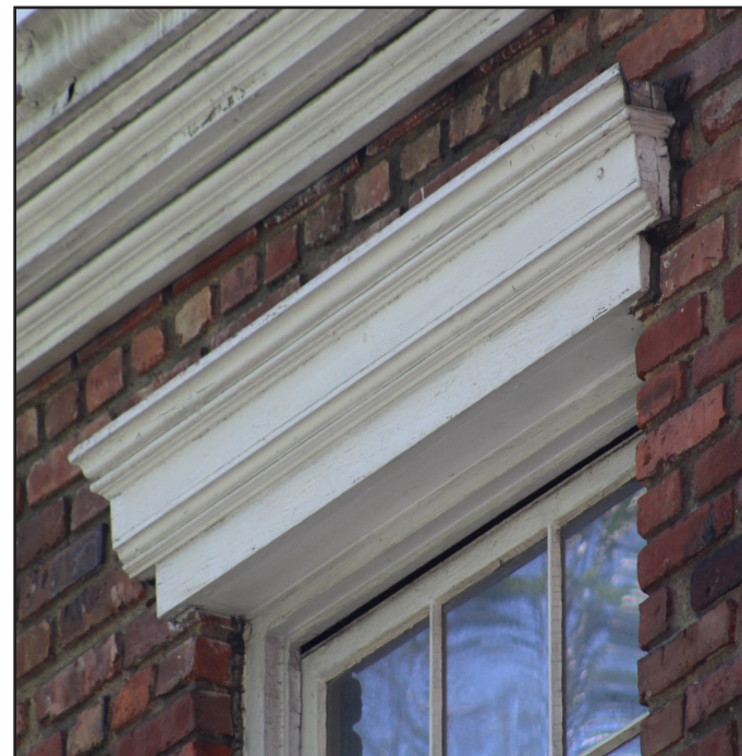
NON-HISTORIC 2ND & 3RD FLOOR WOOD LINTEL
