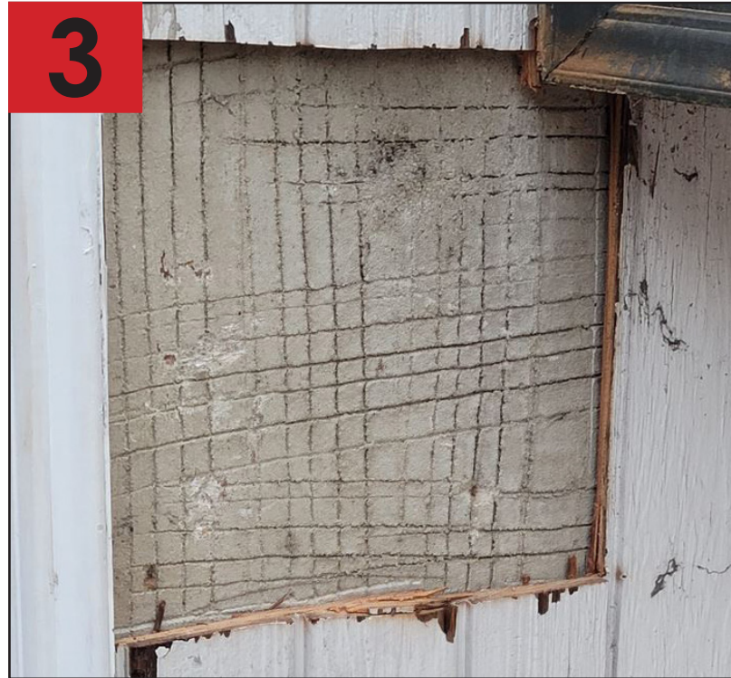
PROBE AT GROUND FLOOR BASE REMOVING WOOD PANELING
