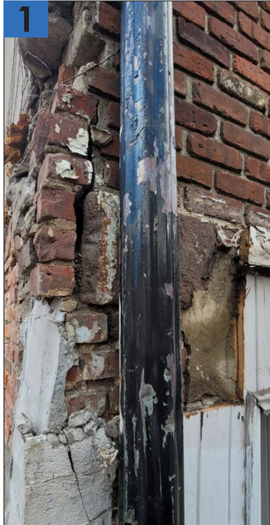
PROBE AT GROUND FLOOR FRONT FACADE LINTEL
