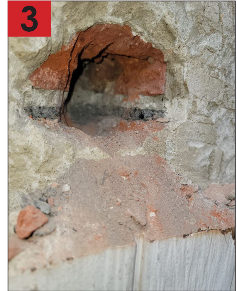
PROBE AT GROUND FLOOR BASE REMOVING SECOND LAYER OF CEMENT PARGING
