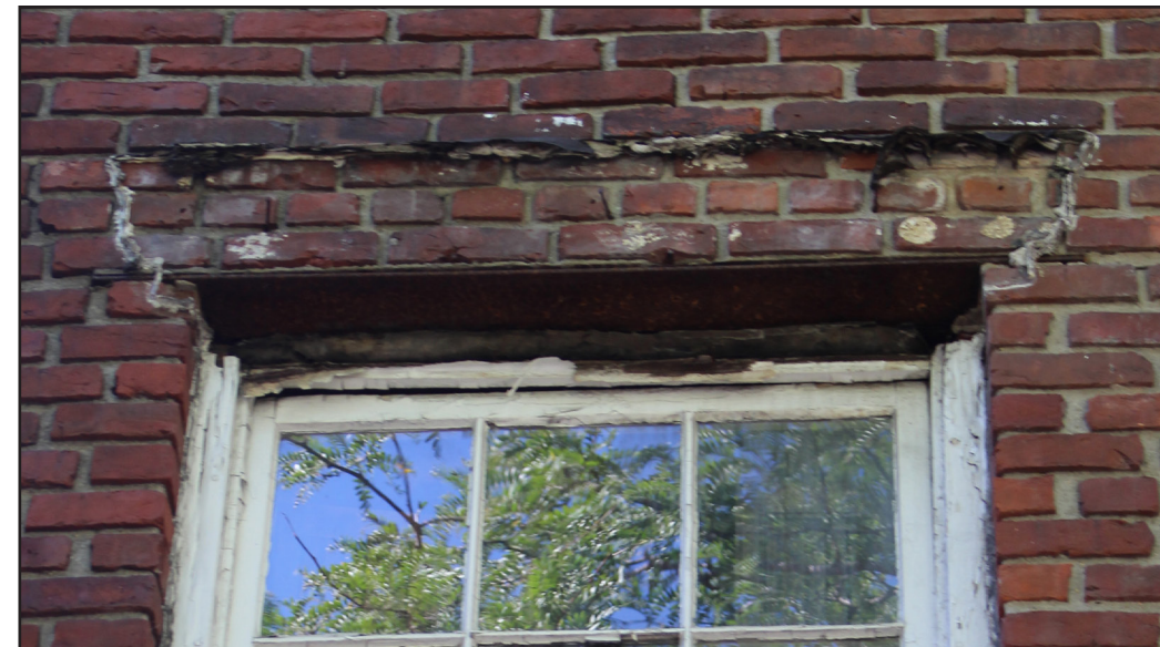
REMOVED NON-HISTORIC 2ND & 3RD FLOOR WOOD LINTEL
