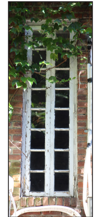
THIRD FLOOR DOUBLE CASEMENT WINDOWS
