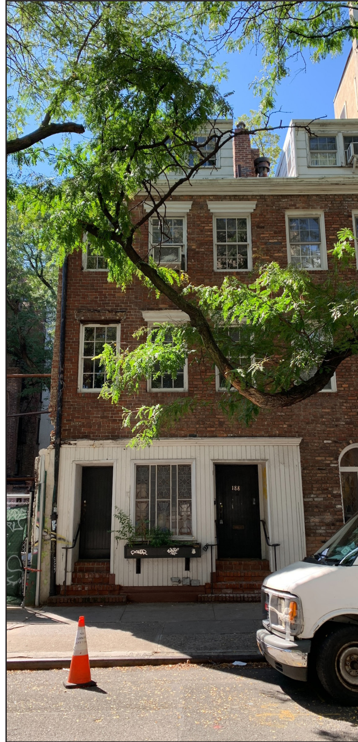
PHOTO 2 FRONT VIEW LOOKING SOUTH
