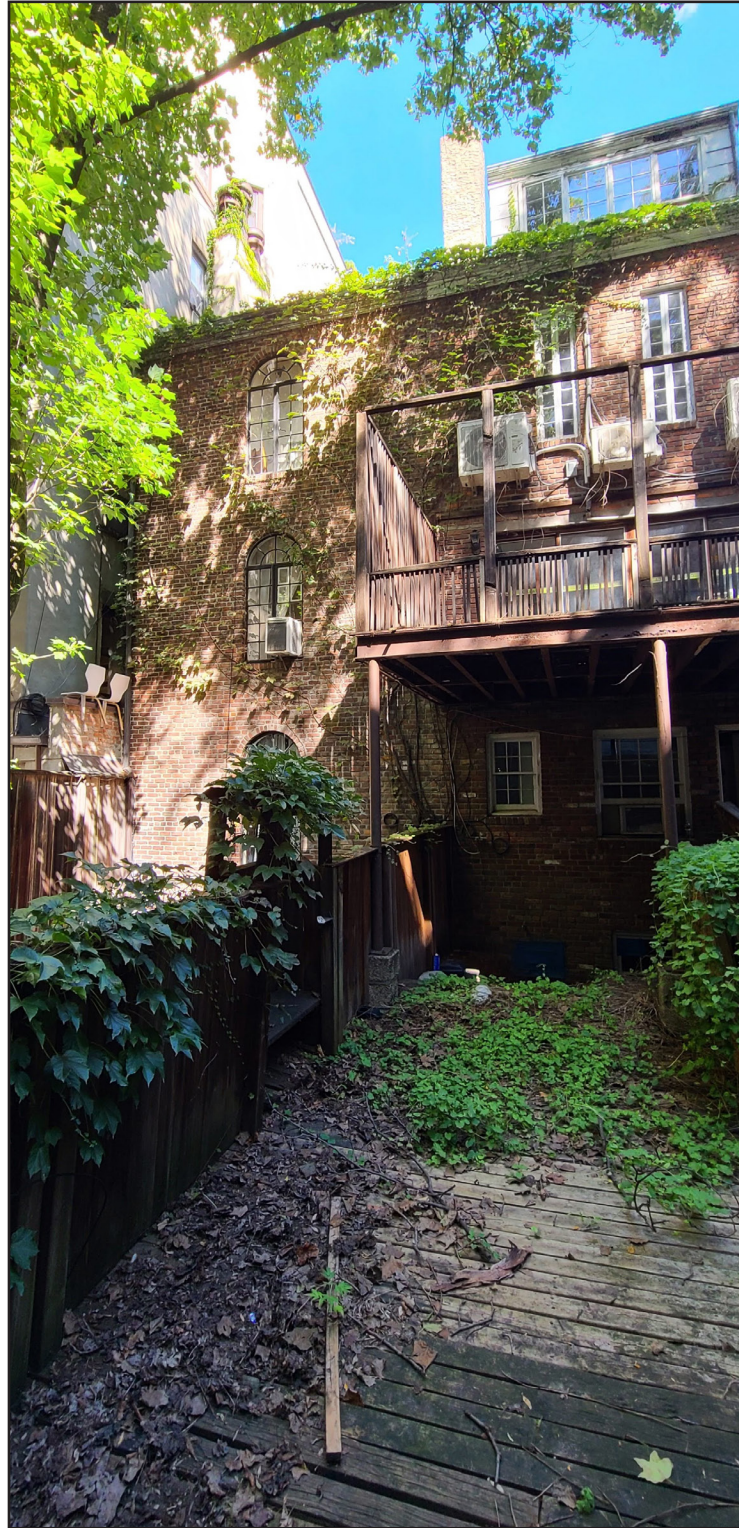
PHOTO 1 REAR VIEW LOOKING NORTHWEST
