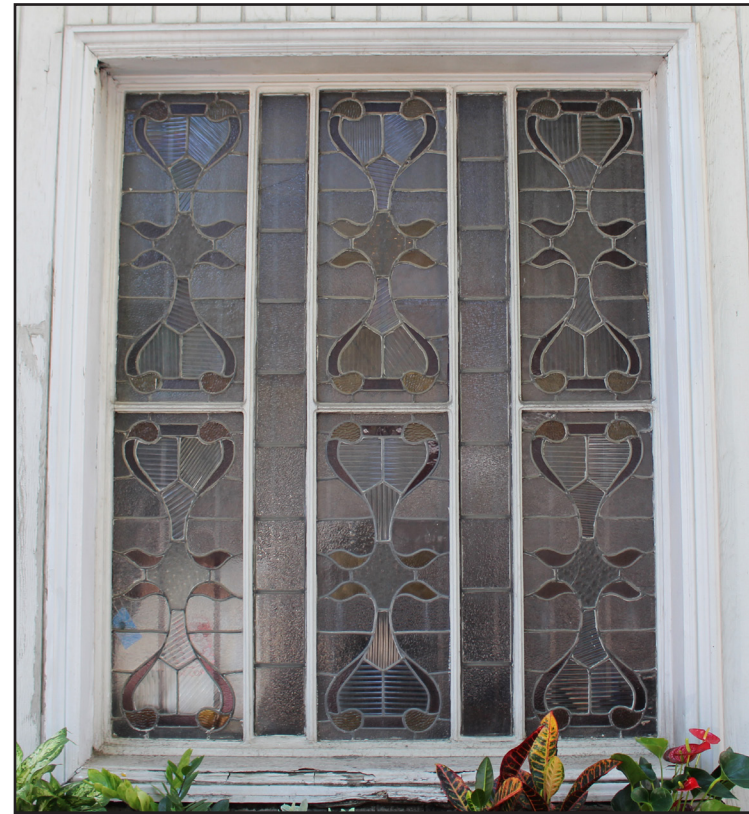
1960s FIRST FLOOR FIXED STAINED GLASS WINDOW
