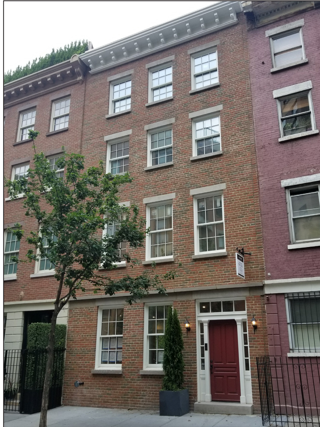
4 BEDFORD ST | LPC 16-3137 ALTERED FEDERAL
