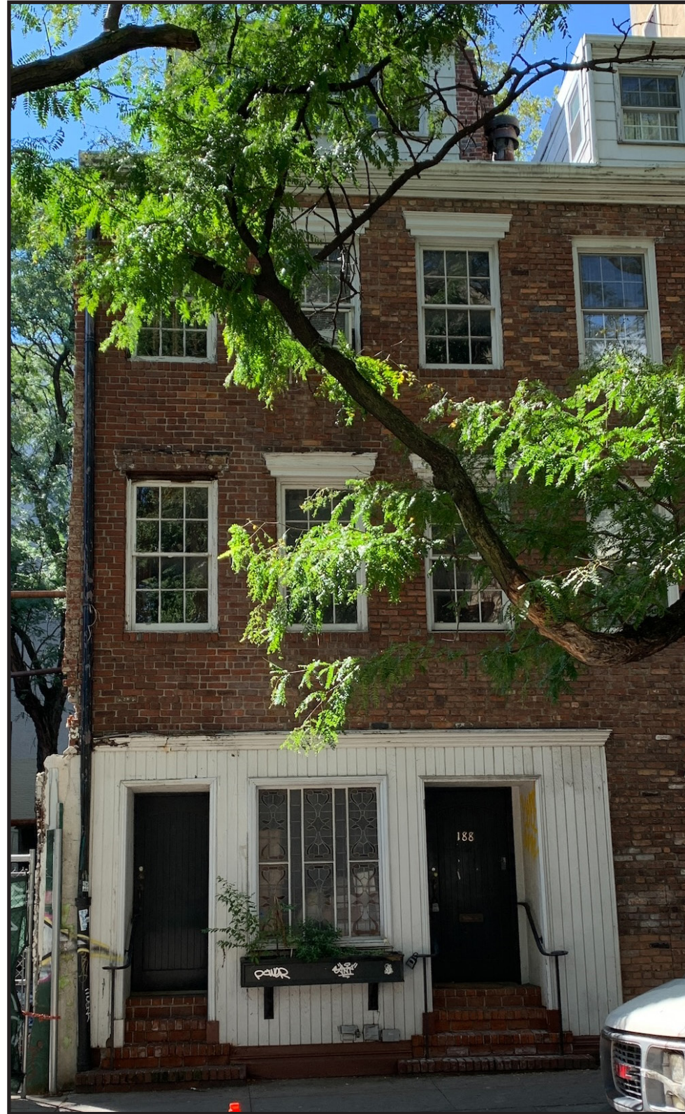
188 SPRING ST EXISTING FRONT FACADE
