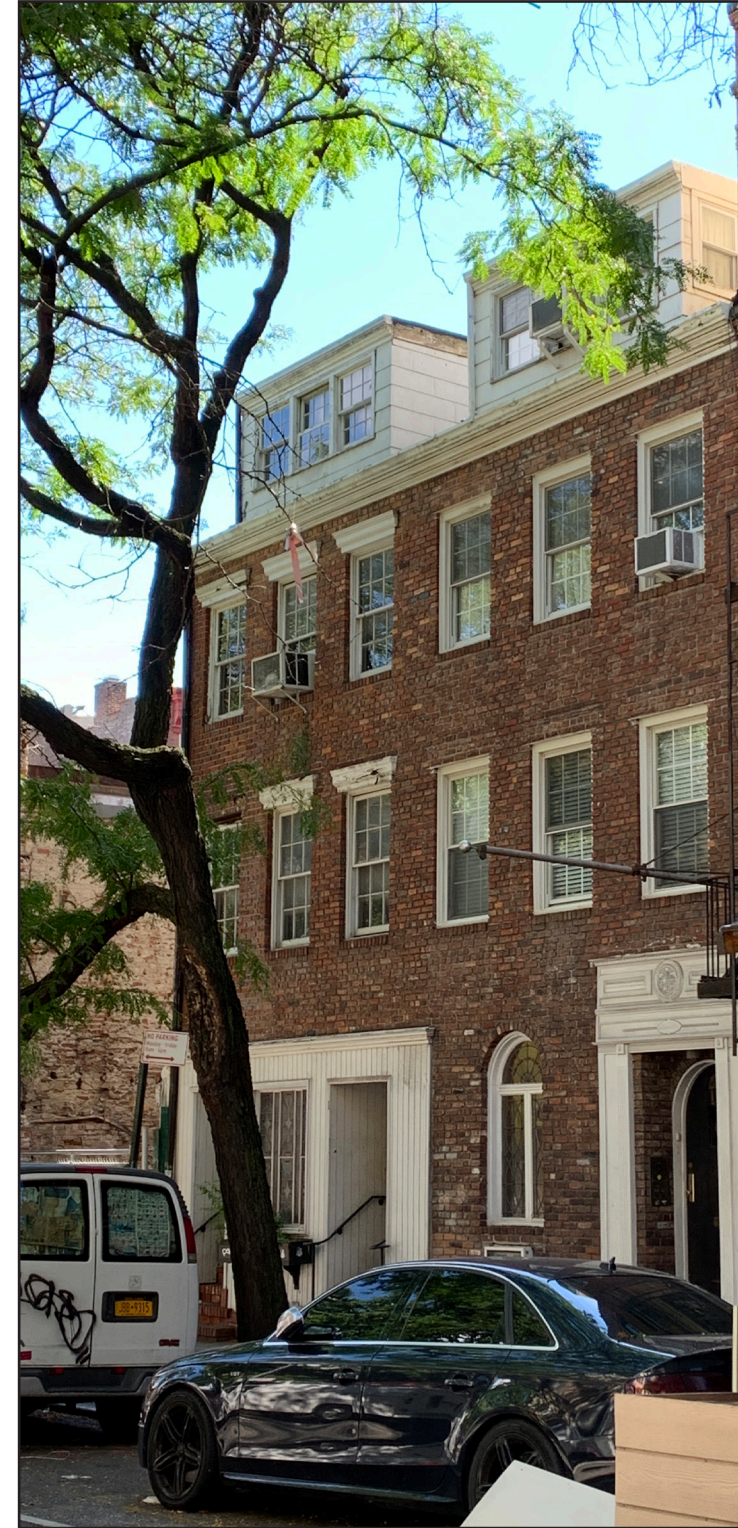
PHOTO 3 FRONT VIEW LOOKING SOUTHEAST
