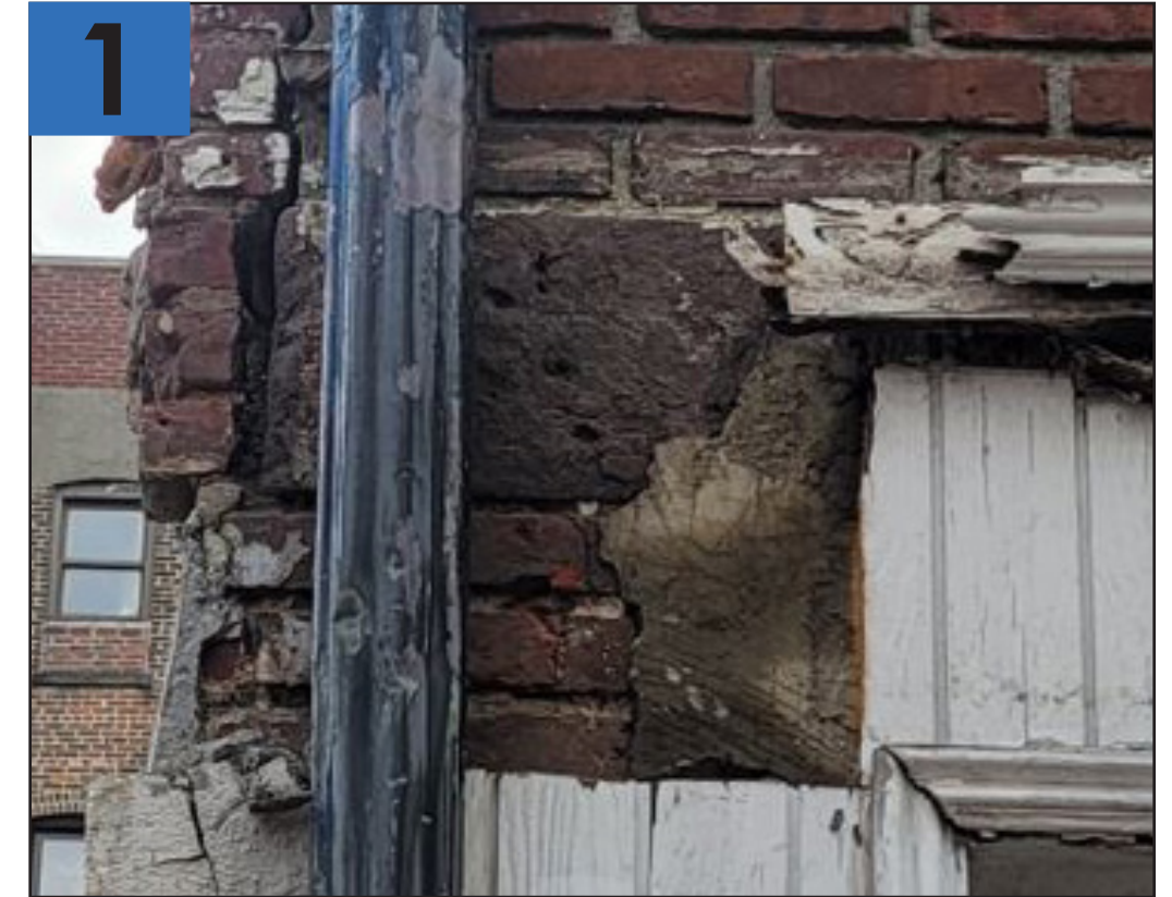
PROBE AT GROUND FLOOR FRONT FACADE LINTEL
