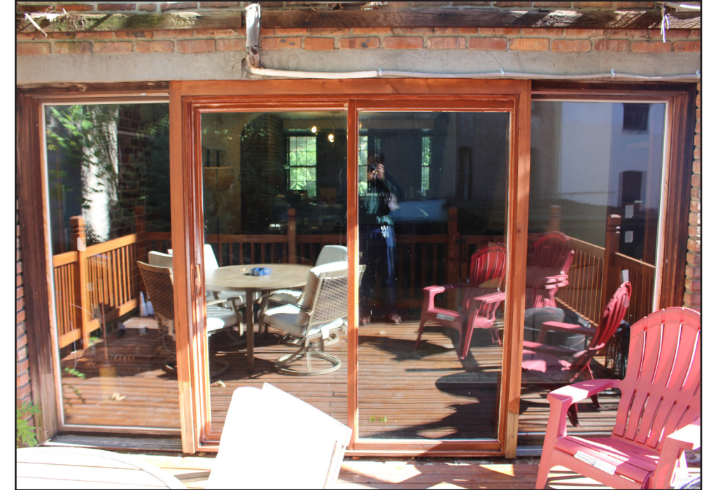
SECOND FLOOR GLAZING
