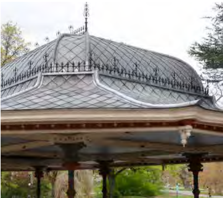
Concert Grove and Pavilion - Metal flashing and roof details, wood molding
