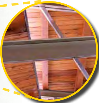
Matte finish metal structure, flashing and coping, with wood auxiliary structure
