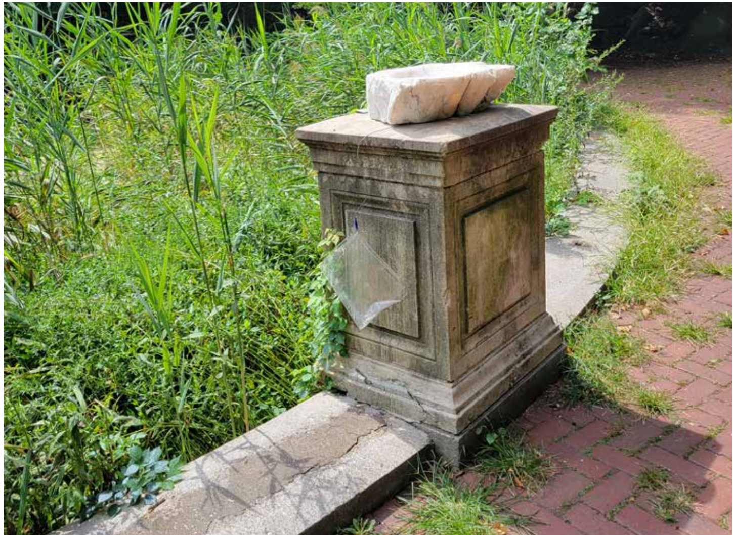
4 - Missing balustrade, damaged piers and invasive plant material in pond
