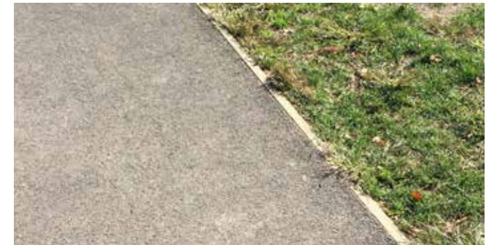
Full Depth Asphalt Pavement and Timber Edge
