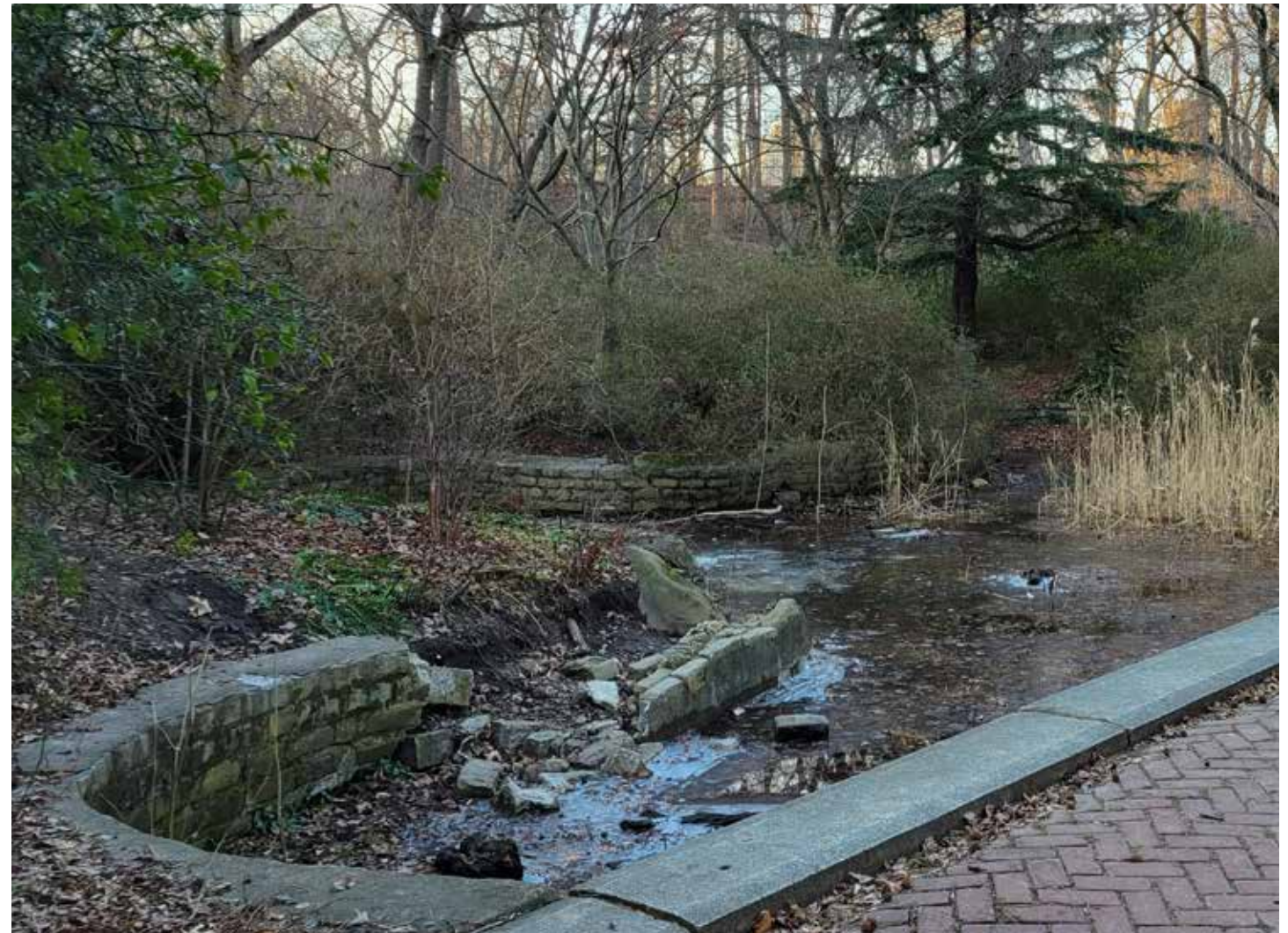
2 - Failing cobble wall
