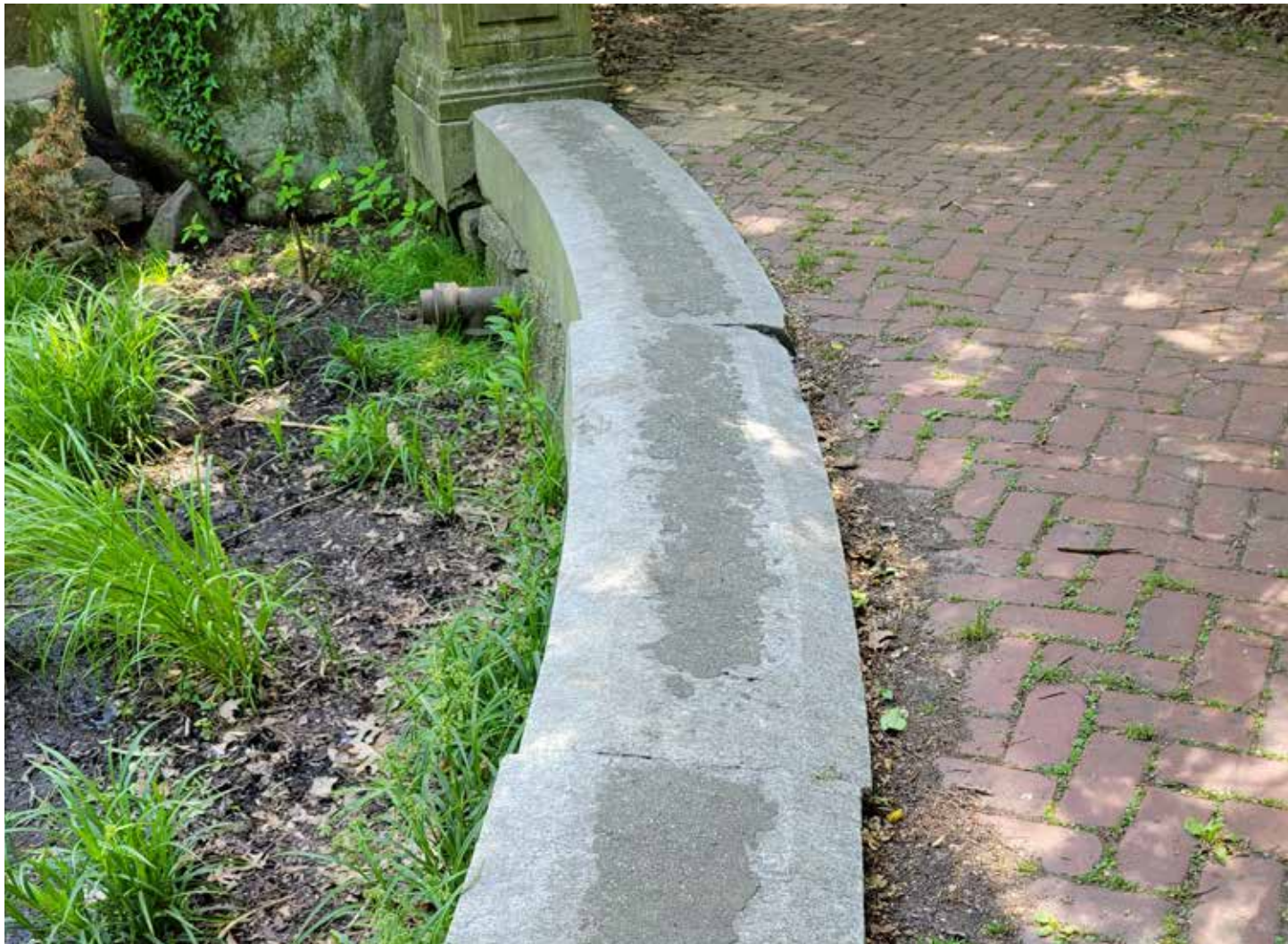
3 - Granite edge damaged & shifting
