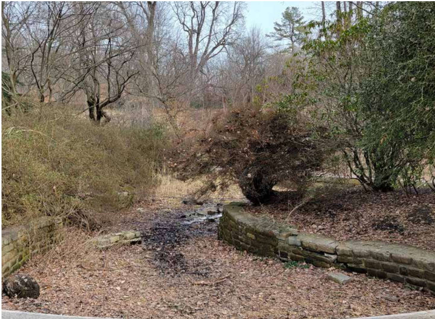
1 - Leaning / failing cobble wall
