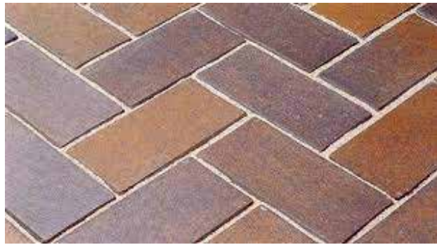
Restored Existing Brick Pavement with Permeable Joints
