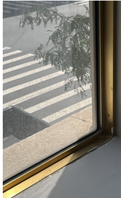
EXISTING BRONZE DISPLAY WINDOW FINISH (INTERIOR & EXTERIOR) Typical @ 2nd Fl building corners Color to be used as reference for new double hung windows
