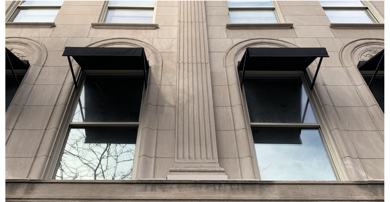
EXISTING DOUBLE HUNG WINDOW Typical @ 2nd and 3rd Fl To be replaced with new bronze type at 2nd Floor - 21 total units
