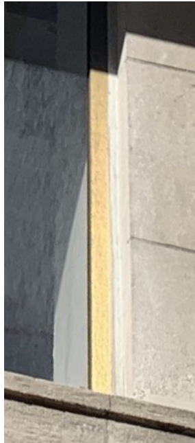
EXISTING BRONZE DISPLAY WINDOW FINISH (INTERIOR & EXTERIOR) Typical @ 2nd Fl building corners Color to be used as reference for new double hung windows
