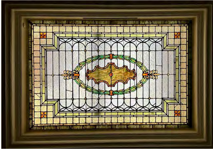
EXISTING HISTORIC LAYLIGHT AT ATTIC CEILING
