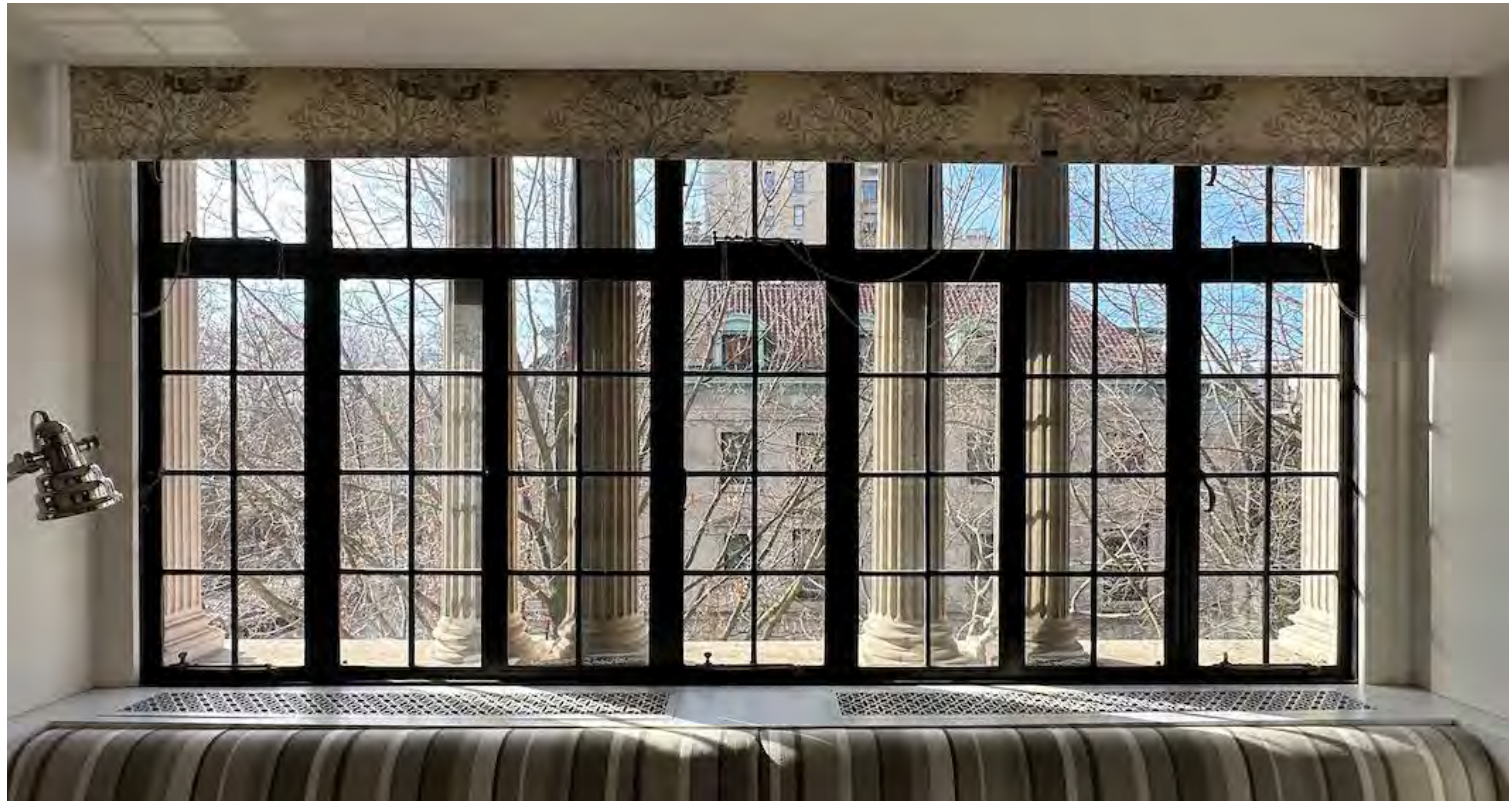
PHOTO OF EXISTING 3RD FL STEEL WINDOWS
