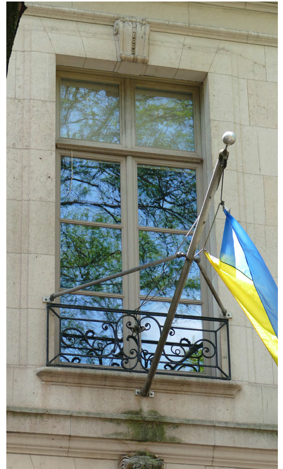
The existing windows at the front facade are retrofitted historic sash with new glazing. The flagpoles will be removed and masonry patched. Biological growth and soiling will be removed.
