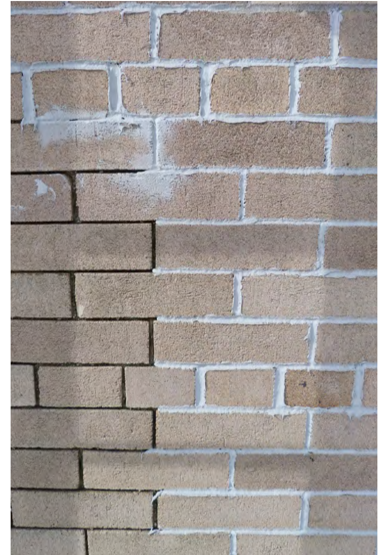
Detail view of poorly done repointing at penthouse elevation.
