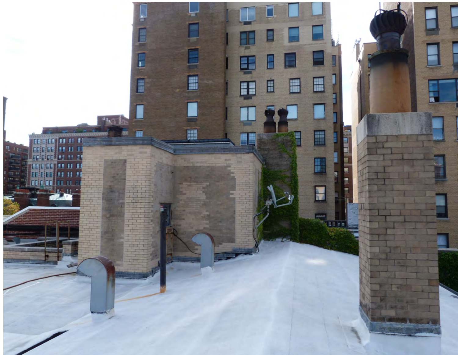
Upper roof, looking east
