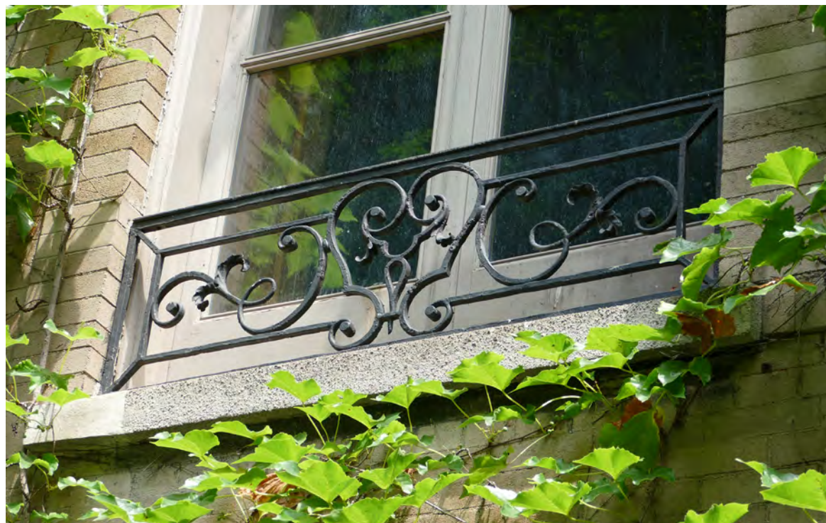
Detail of coated sill and historic ironwork. Historic masonry and metal will be inspected and repaired as necessary.
