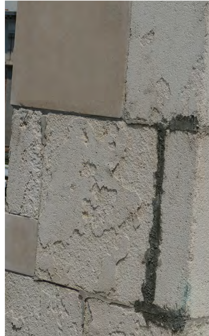
Detail view of stone deterioration at chimney.
