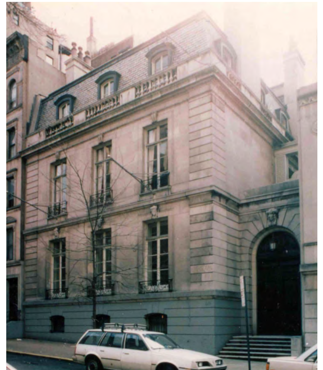
ca. 1993 LPC designation photo
