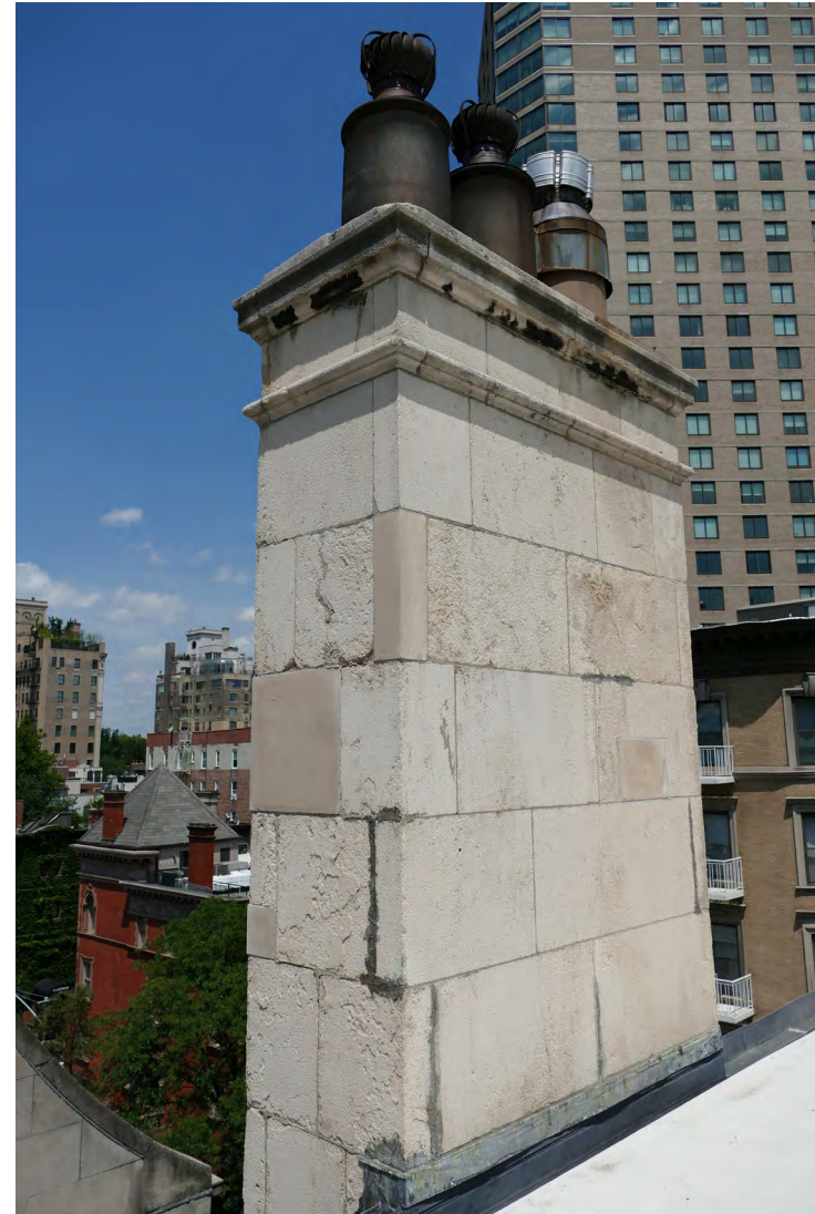
Stone delamination and blackening at chimney. All masonry will be cleaned and repaired.
