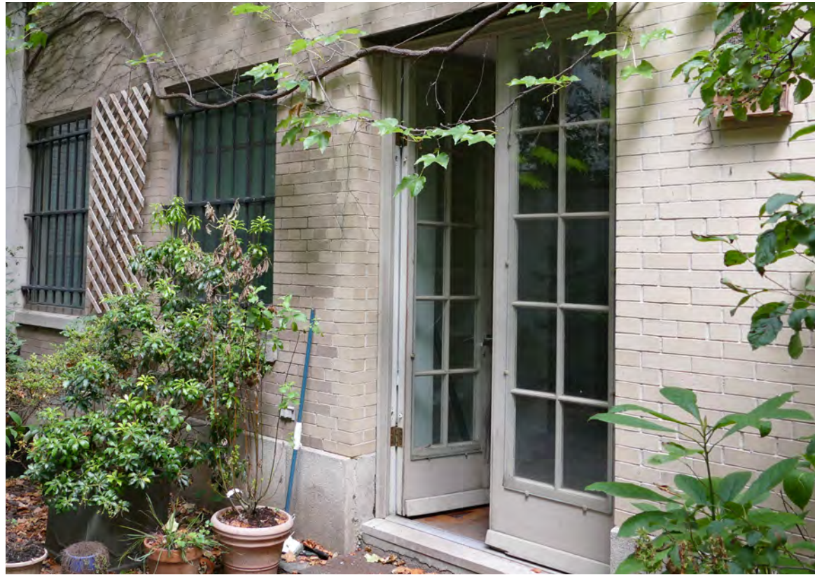
Some masonry openings at the ground floor of the rear elevation have been modified over time.
