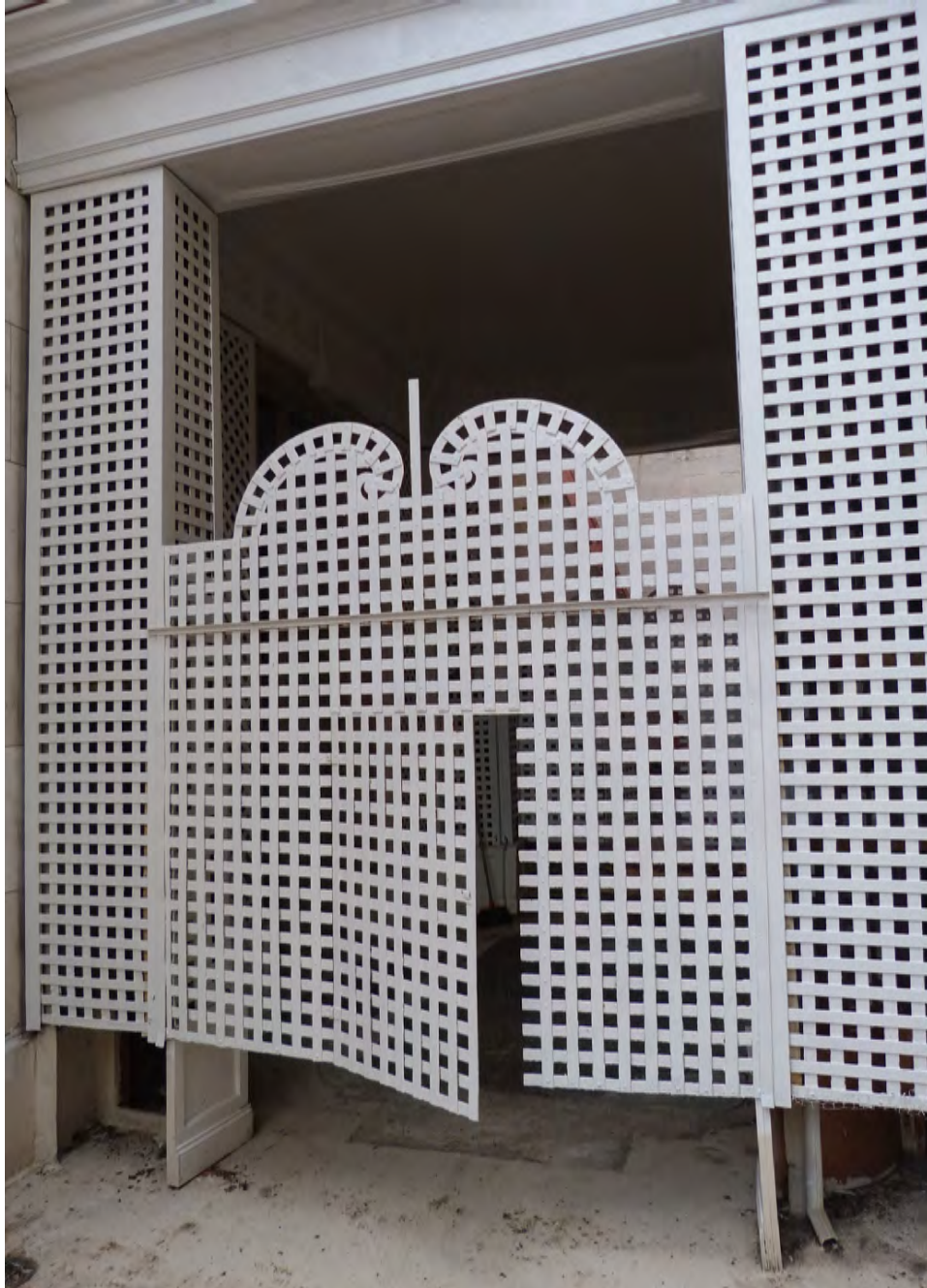
Historic metal to be inspected and repaired as necessary.
