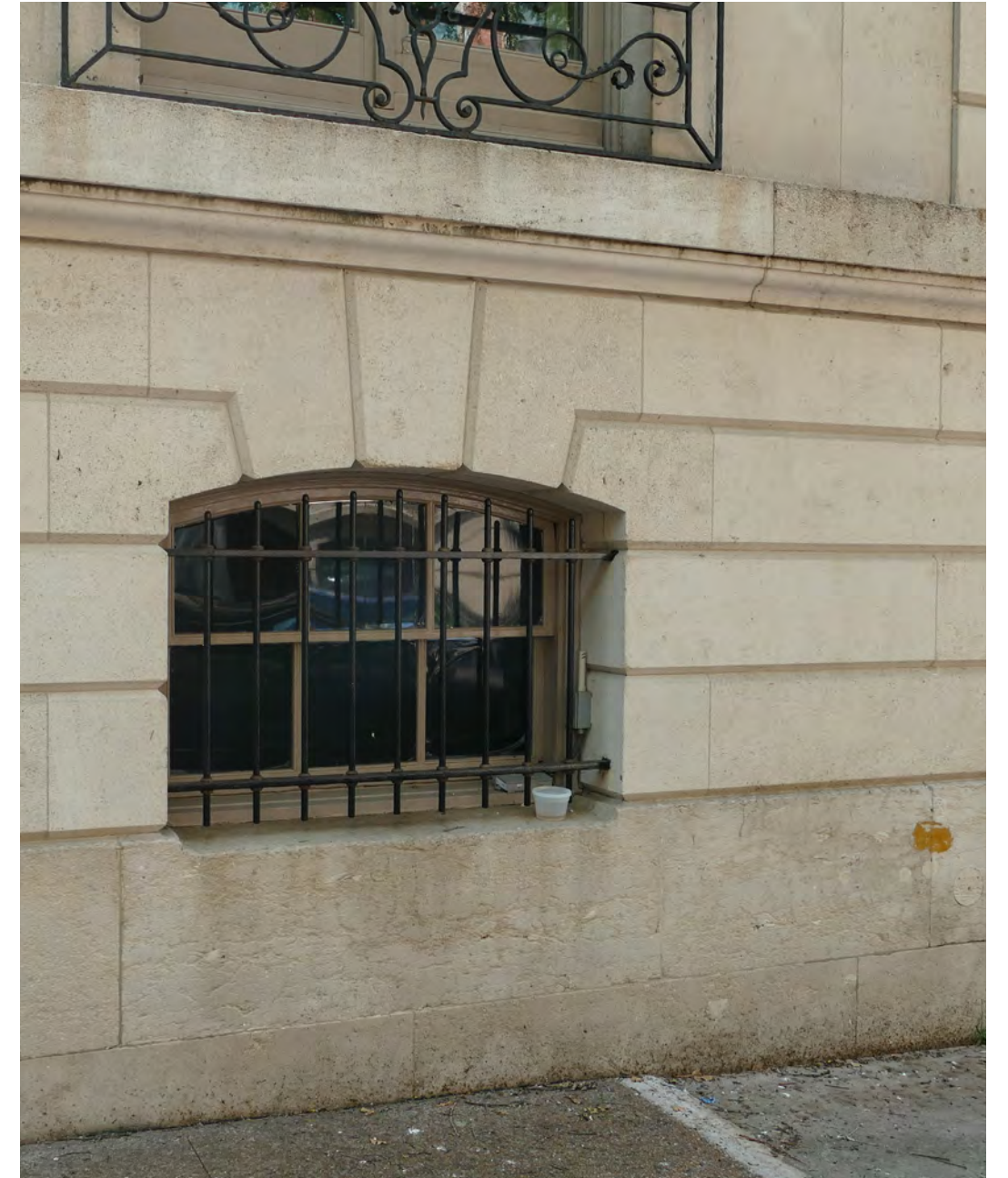
Detail of historic ironwork (to be repaired as necessary) and historic French limestone to be cleaned and repaired.
