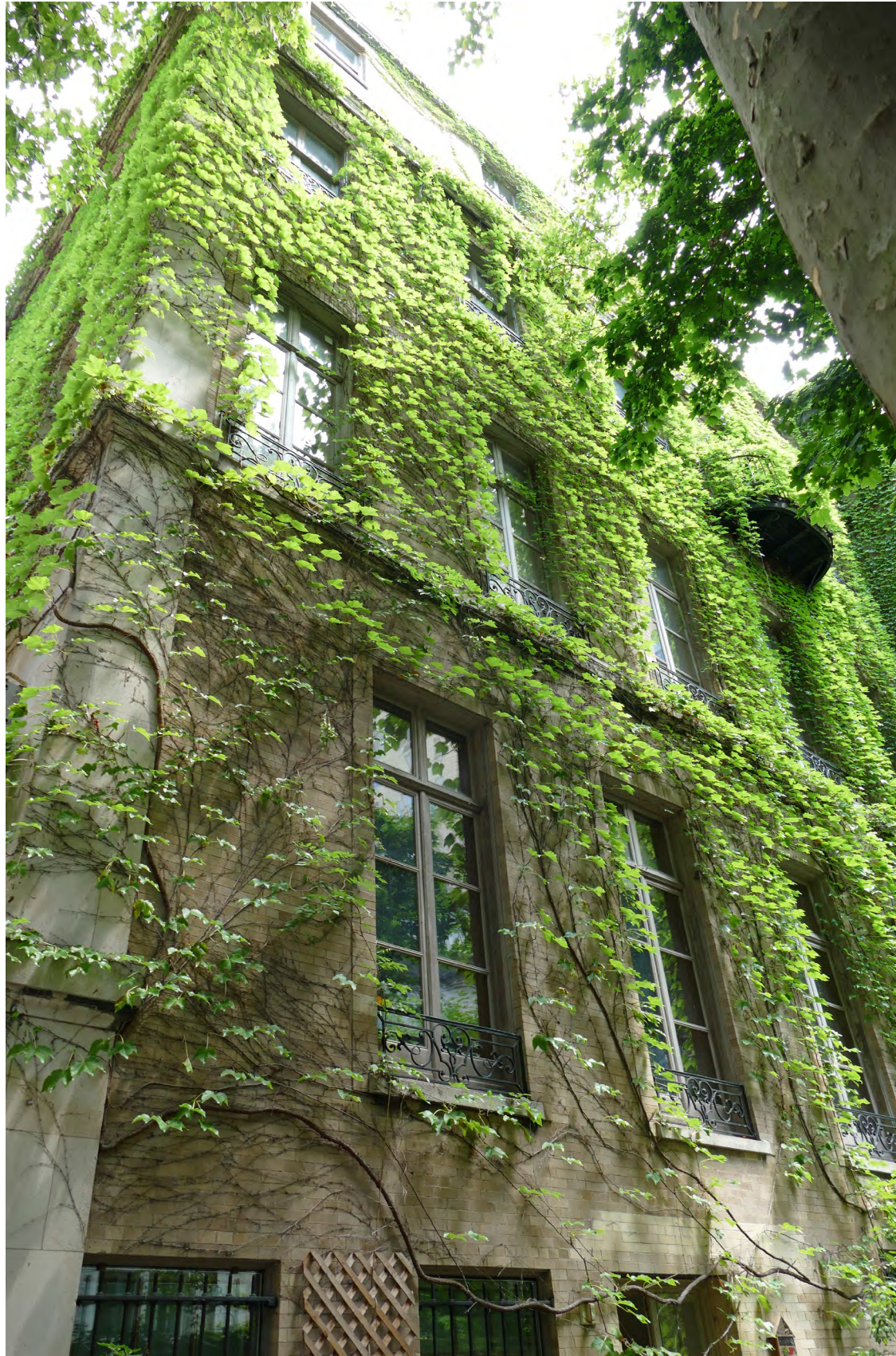
Rear elevation. Vegetation will be removed and the masonry repaired.
