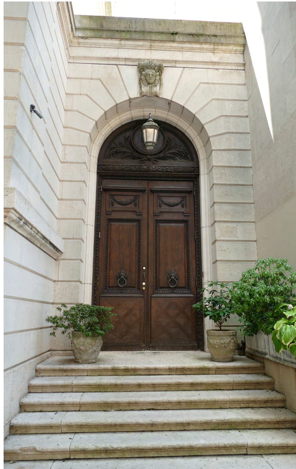
Main entrance. The front entrance door and steps will be restored as part of the preservation scope.
