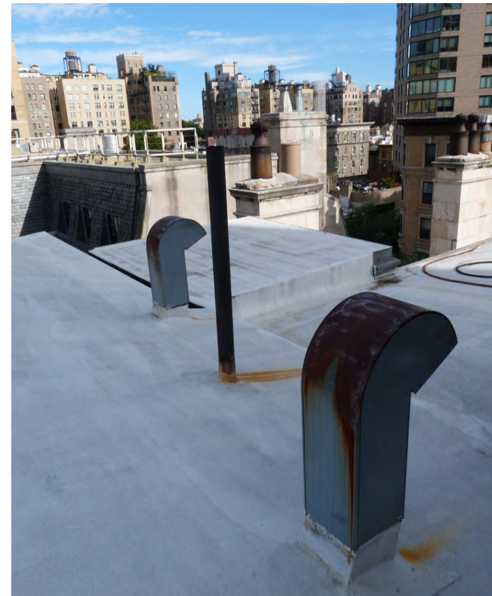
Upper roof, looking northwest
