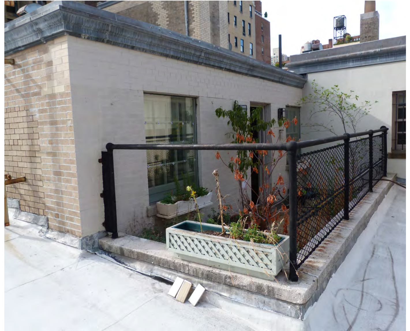
West elevation of historic penthouse
